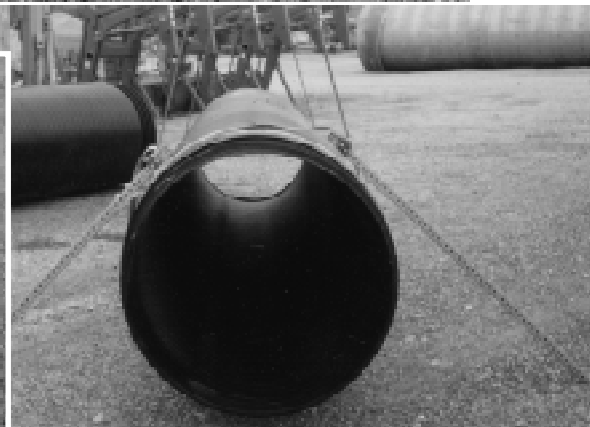
Strap wrenches help twist the liner sections together.
