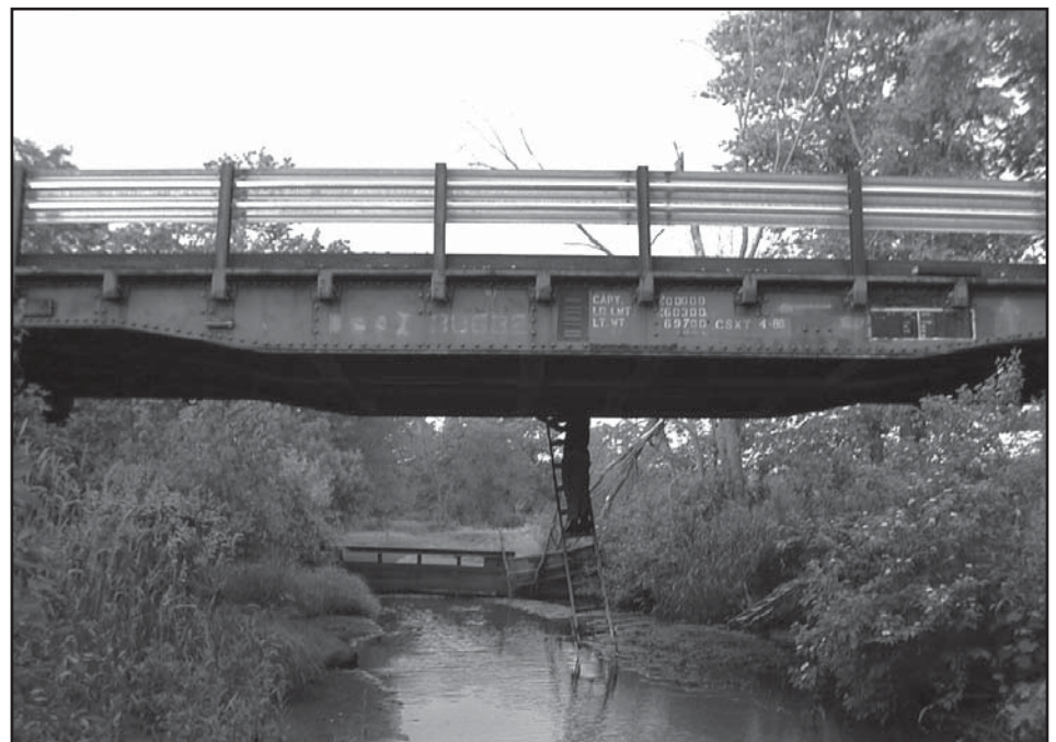
With careful design, engineering, and analysis, Buchanan County is experiencing success with cost-effective railroad flatcar bridges.
