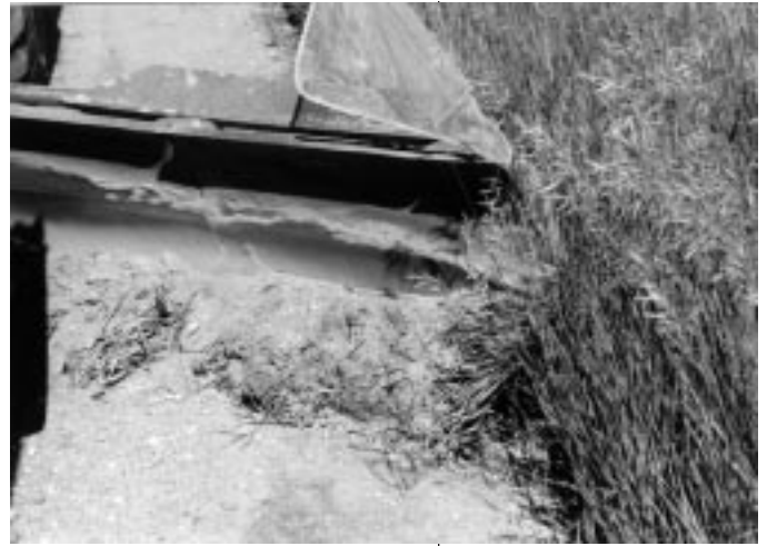
Mix vegetation from shoulders in with the windrow.
