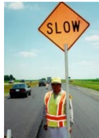
A flagger in the I-35 work zone sports the new safety vest and hat the Iowa DOT is experimenting with this year.
