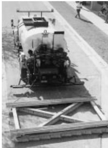
The first truck (left) sprays the asphalt agent and scrubs it into the pavement. A second truck follows, spreading sand and scrubbing that into the pavement as well.
