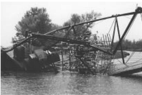
A Boone County bridge was no match for the tractor and field cultivator that crossed on May 10, causing the equipment and bridge to fall into Beaver Creek. *Photo courtesy of the Boone County Engineer.*
