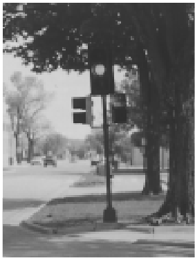
Replacing pedestal mounted signals (top photo) with mast arm mounted signals (bottom photo) contributed to a 36 percent crash reduction.
