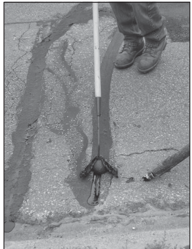
Figure 6. Crack sealing squeegee. Photo courtesy of CCEE Department, ISU.
