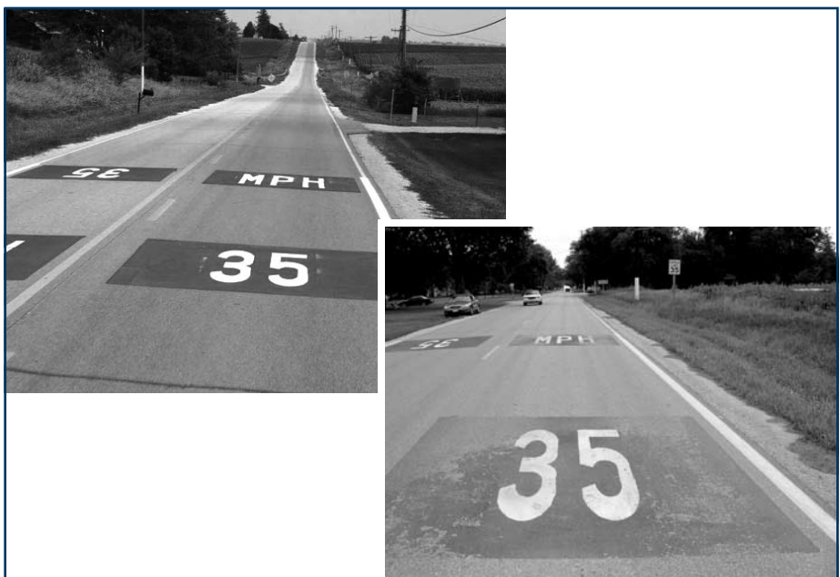
East entrance to Dexter, Iowa, immediately after treatment was installed (left), and west entrance to Dexter after nine months (right).
