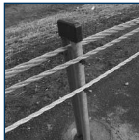
Whenever possible, responders should NOT cut the cable.
