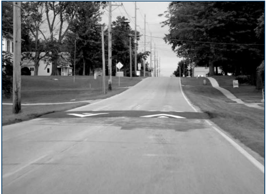
A 30 mph speed table used for residential traffic calming in Gilbert, Iowa.
