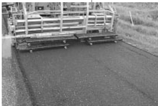
The cold in-place asphalt recycled mat prior to compaction.
