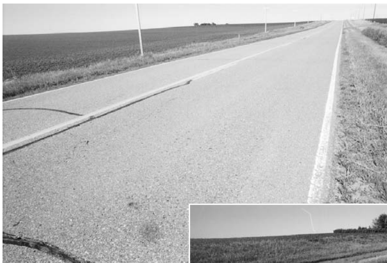
(Below) On the other hand, 26 repair slabs were required on this half-mile section of roadway between a feedlot and a field over which a large, single-axle, dry manure spreader reportedly traveled often. (This view looks east in northern Sioux County.)
