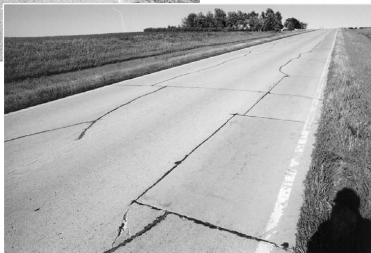
(Below) On the other hand, 26 repair slabs were required on this half-mile section of roadway between a feedlot and a field over which a large, single-axle, dry manure spreader reportedly traveled often. (This view looks east in northern Sioux County.)
