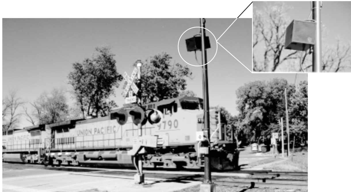
Photos courtesy of the Iowa Department of Transportation
