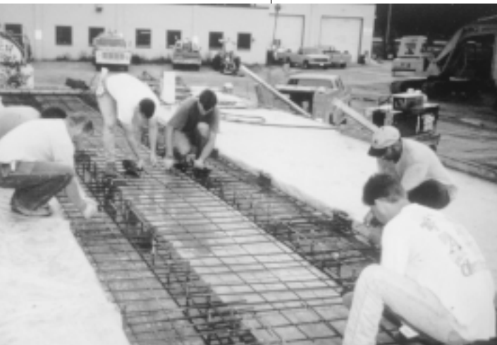
The Black Hawk County bridge crew worked with researchers to build the precast units (left). Below is an overhead view of the units. Photos courtesy of Wayne Klaiber.
