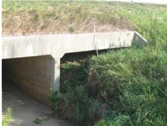
Figure 2.4.5.2.1-1 - Silt Accumulation
