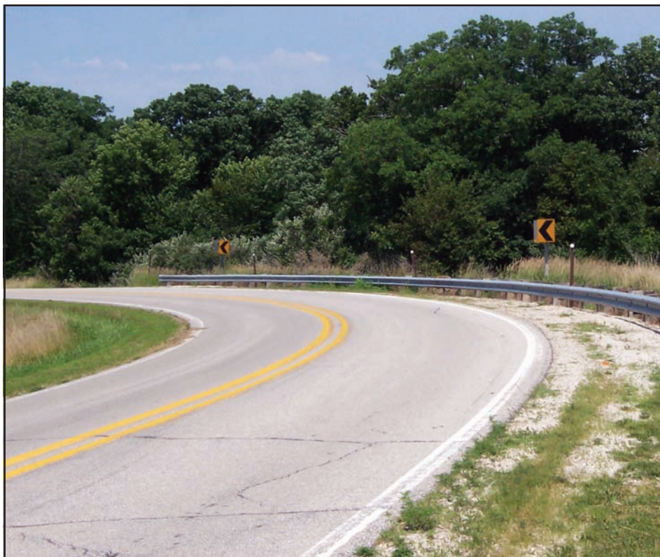
Chevrons installed on a curve. (Photo courtesy of Bob Sperry)
