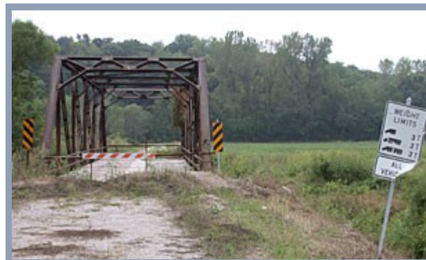
Site of new UHPC bridge to be constructed in Wapello County
