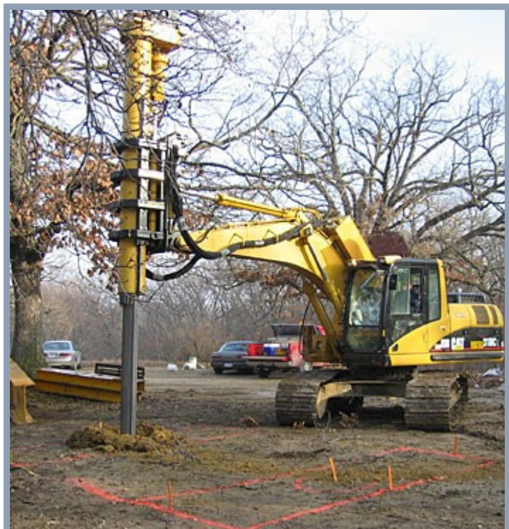
Drilling a Geopier® foundation
