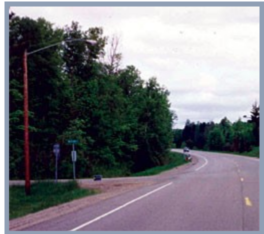
Lights at the Highway 65 and West Bay Drive intersection in Itasca County, Minnesota, improve driver safety at night.
