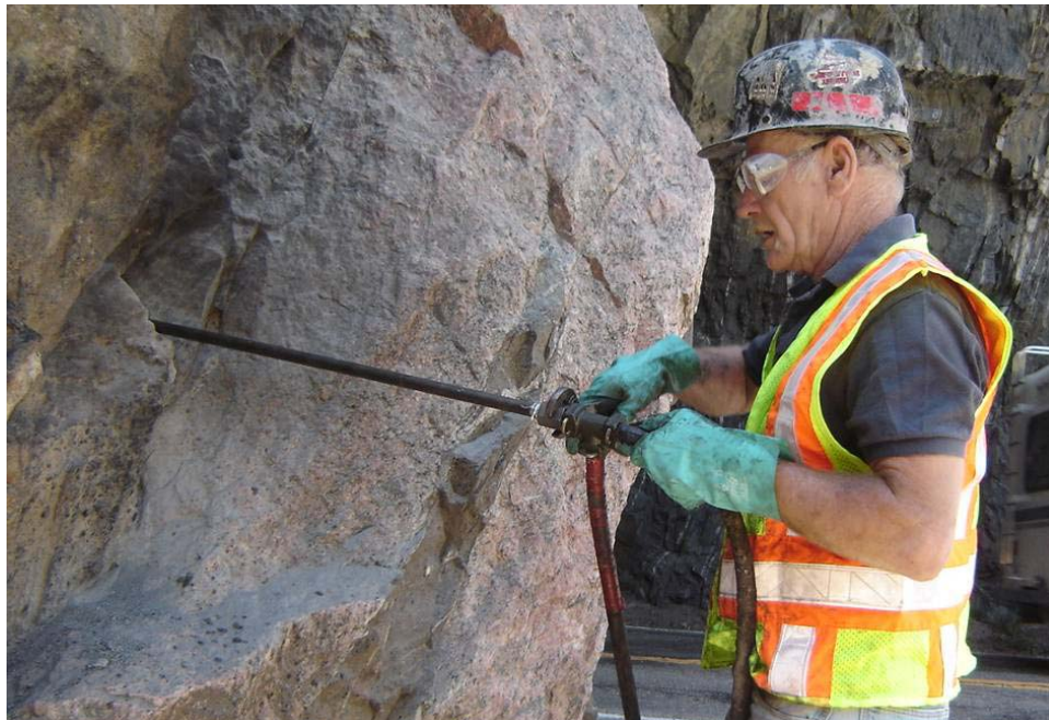
Figure 7. Photo. Connection of PUR Component A and B hoses to injection port.
