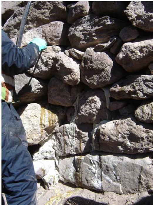
Figure 24. Photo. PUR injection directly between wall facing rocks using a hand-held injection nozzle.
