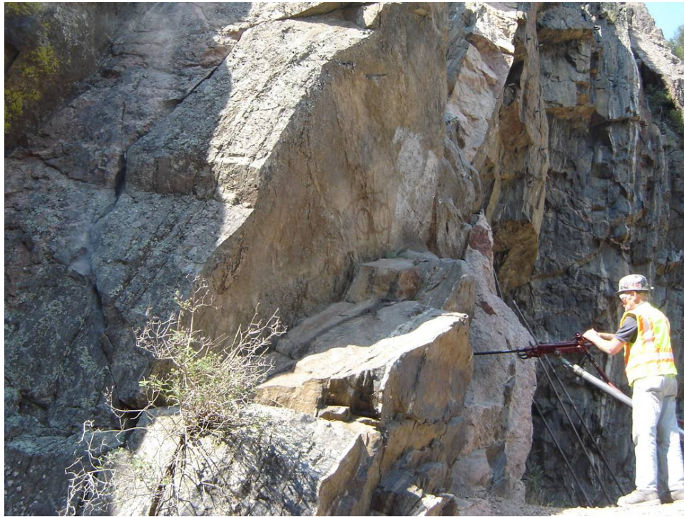
Figure 5. Photo. Jackleg drilling into western portal abutment (Hole # 1).
