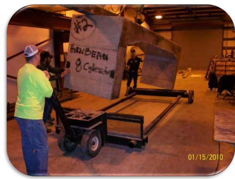
three-sided box culverts. The problem was moving the recently-poured pre-cast concrete structure out of the culvert shop and into the yard safely. The boxes weigh anywhere from six tons to ten tons depending on their sizes; this made using the forklift difficult (if not dangerous) to move over a long distance to the yard. The main concerns were upsetting the forklift, point-loading of the box onto the forks, and the box sliding off the forks en route to the yard.
