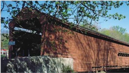
Figure 2.1 Figure 2.1 Gilpin's Falls Covered Bridge (1860) in Cecil County, Maryland, was in danger of collapse due to decaying members. An award of $1,040,000 from the NHCBP program funded a sensitive rehabilitation project in 2009–2010. Left: 2.1a) The deteriorating bridge awaiting repair. Carol M. Highsmith Archive, Library of Congress, Prints and Photographs Division, Washington, D.C., between 1980–2006. Right: 2.1b) Stabilizing the truss during Tim Andrews' rehabilitation. HAER MD-174-4, David Ames, photographer, 2009.
