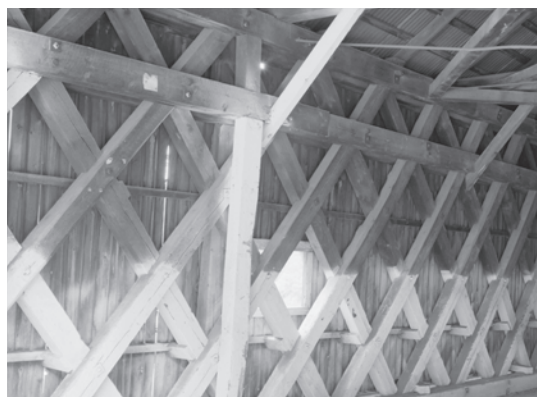
Figure 5.17 A detail of the squared-timber lattice truss on Bela Fletcher and James Tasker’s Cornish-Windsor Bridge (1866). The 6 x 8-inch timbers were connected at each joint by a notch and a single bolt instead of a pair of tree-nails. HAER NH-8-10, Jet Lowe, photographer, 1984.
