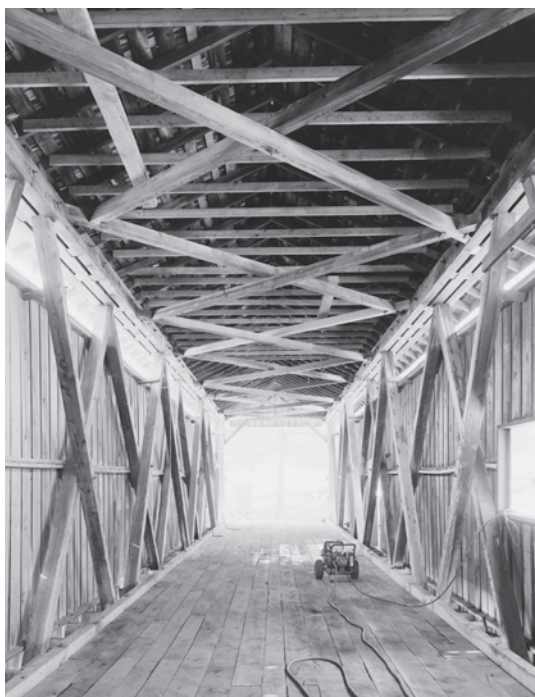
Figure 5.42 Cataract Bridge (1876) is a 140-foot Smith "double-truss" (Wilson type 3). The truss, the portal bracing, and the lateral bracing between the upper chords were all patented by Robert Smith. Note how both tension and compression diagonals are notched into the chords at midspan. HAER IN-104-6, James Rosenthal, photographer, 2004.
