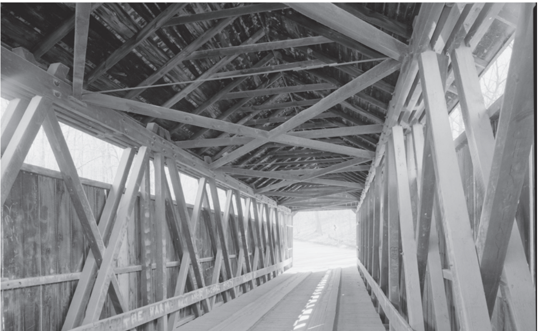
Figure 0.43 White's Bridge (1869) in Kent County, Michigan, was the best surviving example of this truss patented in 1857 by Josiah Brown before it was lost in a fire in 2013. The regional Brown truss featured paired braces and single counters notched and bolted at the chords. HAER MI-331-8, Jet Lowe, photographer, 2004.
