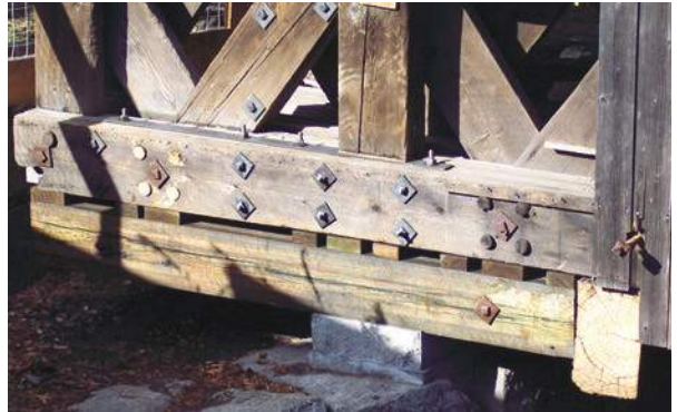
Figure 7.10 The replacement bed timbers installed on Contoocook used a bolted coupling splice inspired by a technique developed for similar structures by Snow and Fletcher in the 1930s. Note the granite pedestal supporting the corbel. Will Truax, photographer, 2007.
