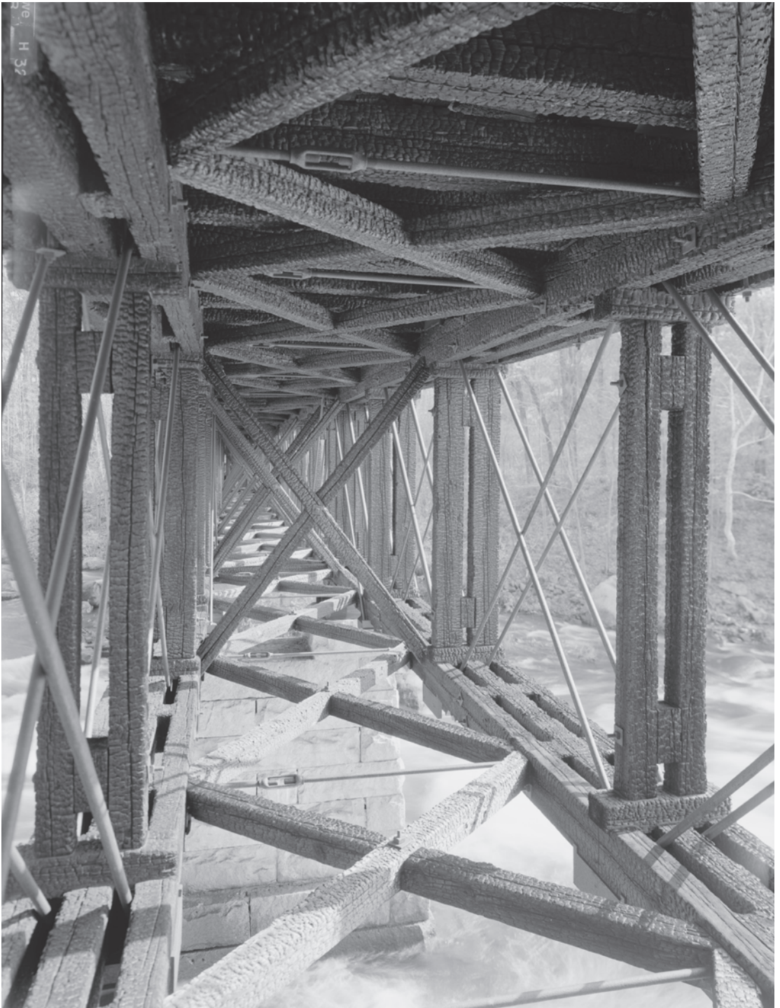
Figure 0.34 Although burned by arsonists in 1980, the Sulphite Railroad Bridge (1896) in Merrimack County, New Hampshire, survives as an example of a wood and iron Pratt deck truss. Patented by Thomas and Caleb Pratt in 1844, the Pratt truss reversed the configuration of the Howe truss, placing the short web members in compression and the long web members in tension, which reduced the danger of structural failure through buckling. Few timber Pratt-truss bridges were built, but the type was successfully adapted to iron and steel. By the late nineteenth century, the all-metal Pratt truss was the standard American truss for moderate railroad and highway spans. HAER NH-36-7, Jet Lowe, photographer, 2003.
