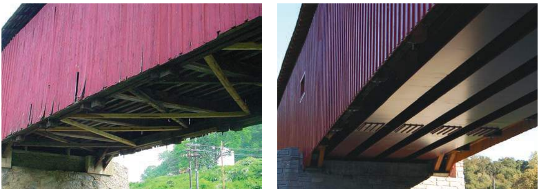
Figure 7.14 In 2002, the HAER documentation team found the original lower chord, lateral bracing, and stone abutments of Pine Grove Bridge in Lancaster County, Pennsylvania, as constructed by Elias McMellen in 1884, still intact. While the Pennsylvania Department of Transportation saved the Burr-arch trusses in 2008, they unfortunately replaced the lower timbers with steel I-beam and removed all of the stonework, constructing new concrete abutments with a form liner surface treatment. Top: 7.14a) HAER field photo, 2002; Above: 7.14b) Tom Vitanza, photographer, 2009.
