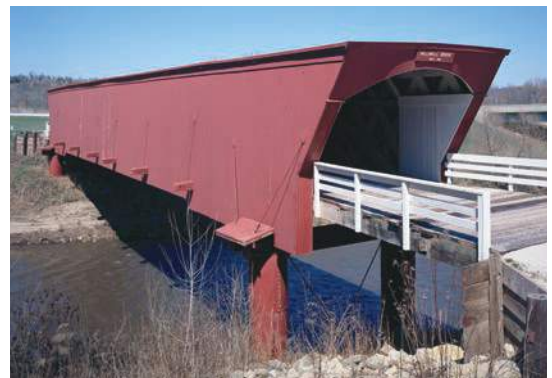
Figure 3.16 Top Left: 3.16a) Dreibelbis Station Bridge (1869) in Berks County, Pennsylvania, exhibits the masonry approach walls and stepped gables that were original characteristics of covered bridges in southeastern Pennsylvania. HAER PA-587-4, Jet Lowe, photographer, 2002. Top Right: 3.16b) Holliwell Bridge (1880) in Madison County, Iowa, exhibits the nearly flat roof and gracefully arched portals that were used in several of the county's covered bridges. HAER IA-64-27, Jet Lowe, photographer, 2004. Left: 3.16c) Swann Bridge (1933) in Blount County, Alabama, is clad in the corrugated metal roofing and siding adopted to house a number of the county's covered bridges in the 1930s. HAER AL-201-4, Jet Lowe, photographer, 2002.
