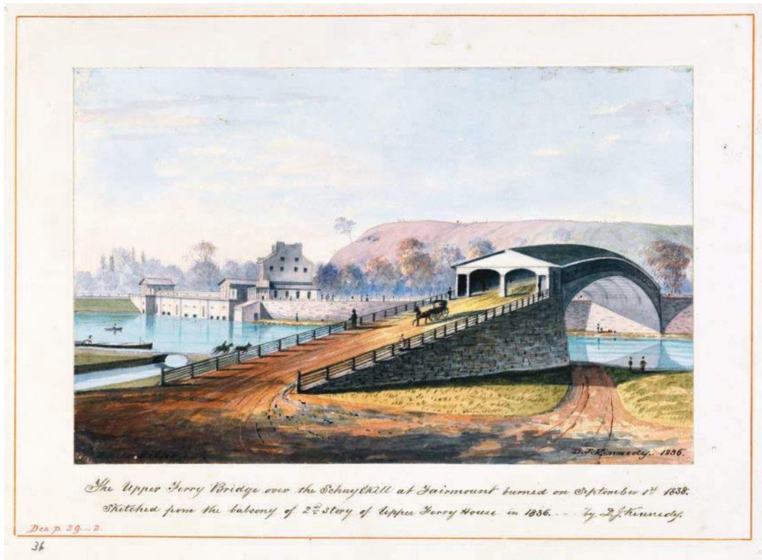
Figure 3.6 Upper Ferry Bridge over the Schuylkill, watercolor by David J. Kennedy, 1836. Erected in 1812 by German-born mechanic Lewis Wernwag, the Upper Ferry Bridge, also known as the Colossus, was an early masterpiece of American civil engineering. Spanning the Schuylkill River at Philadelphia, the 340-foot structure was the longest clear-span bridge in the world at the time of its construction, and the second-longest timber bridge built during the historic era of covered bridge construction. The Colossus carried traffic for a quarter of a century before it was destroyed by fire in 1838. Courtesy of Historical Society of Pennsylvania, Philadelphia, Pennsylvania, David J. Kennedy watercolors.
