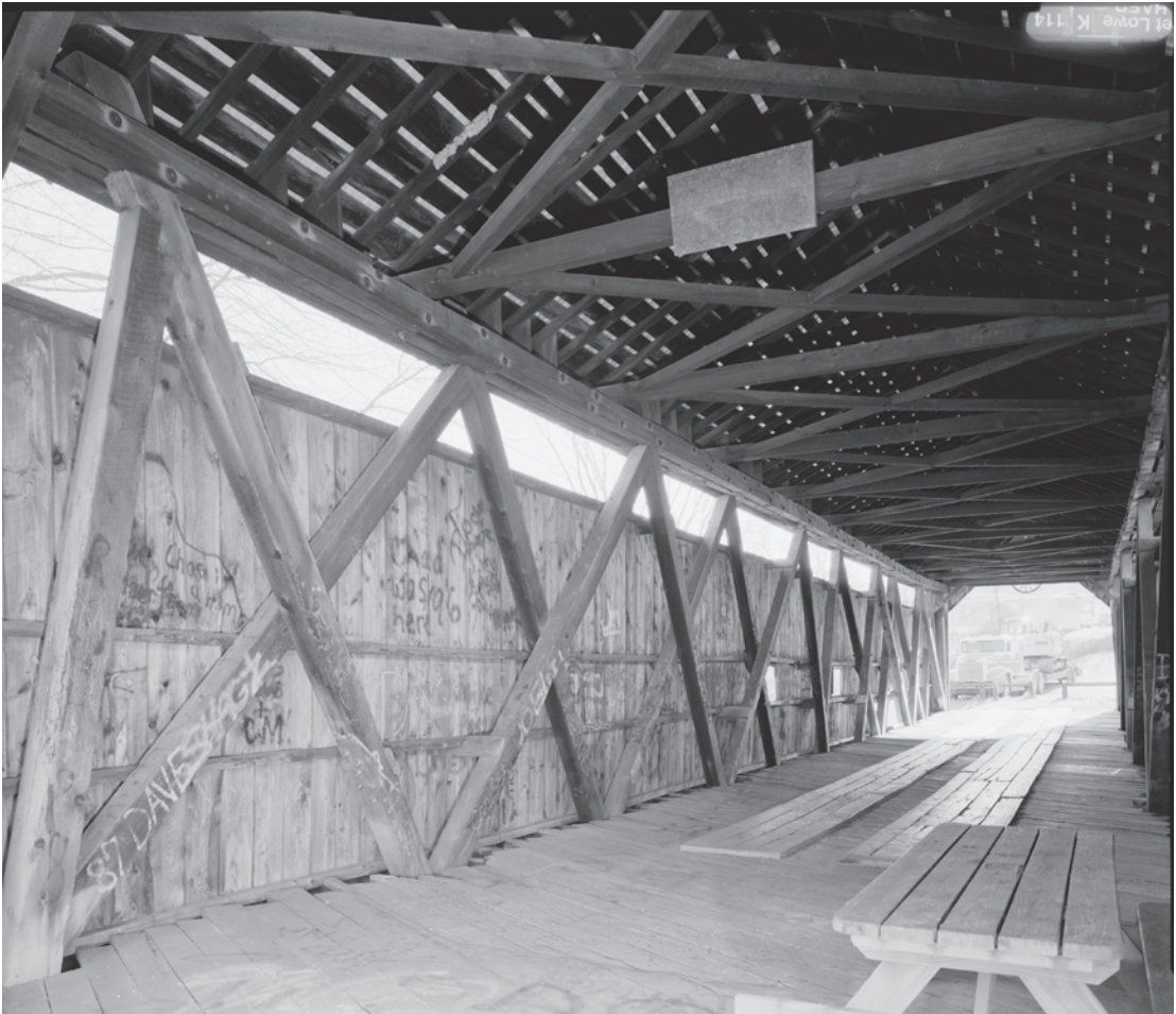
Figure 0.35 This end panel of Kidd's Mill Bridge (1868) in Mercer County, Pennsylvania, shows the extra, steeply inclined compression brace common to trusses patented by Robert W. Smith, who successfully introduced industrial processes into covered bridge construction through his two Ohio companies. HAER PA-622-5, Jet Lowe, photographer, 2006.
