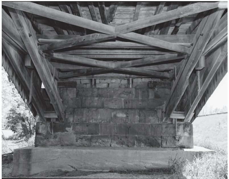
Figure 6.11 A view underneath West Union Bridge (1876) in Parke County, Indiana, shows how J. J. Daniels played his arches around the bottom chords of the trusses. HAER IN-105-9, James Rosenthal, photographer, 2004.
