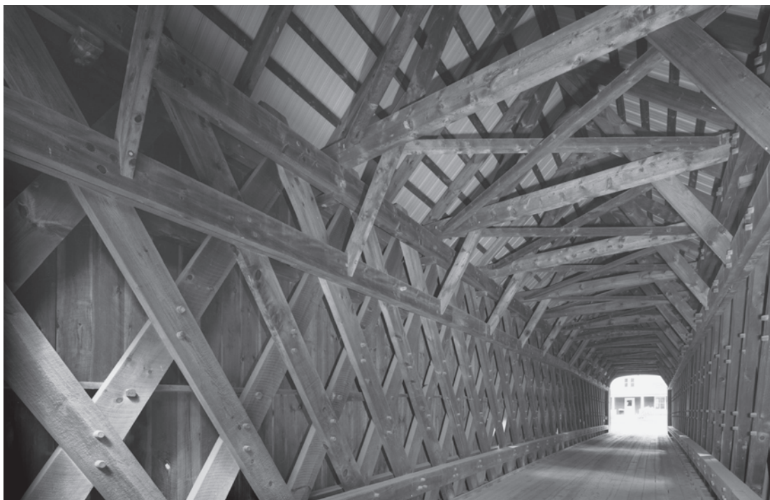
Figure 0.22 The interior view of Milton and Arnold Graton's Hall Bridge (1982) in Windham County, Vermont, showcases the twentieth-century craftsmen's knowledge of traditional timber framing and detailing in constructing a modern authentic covered bridge. HAER VT-40-11, Jet Lowe, photographer, 2009.
