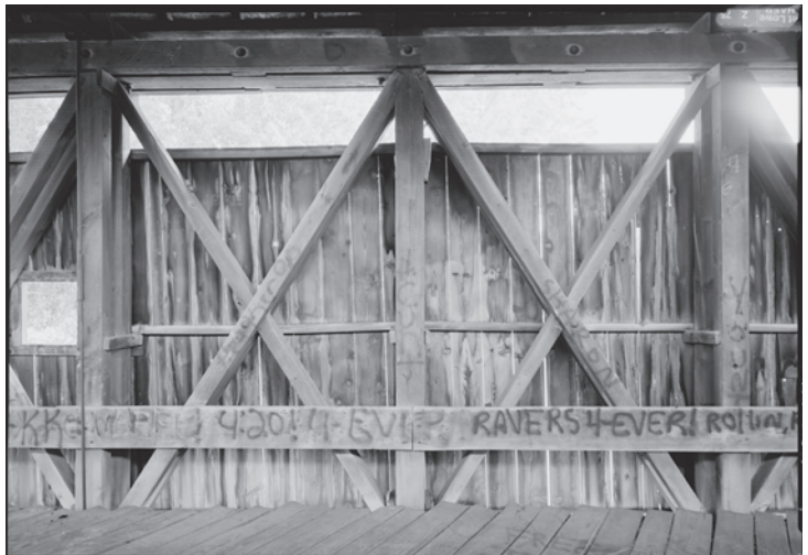
Figure 5.23 Left: 5.23a) Detail view of one of the wedges hammered into the base of each counterbrace on the Eldean Bridge. William G. Keener, photographer, 1998. Courtesy of Ohio History Connection. Right: 5.23b) Interior elevation of Eldean Bridge's Long truss. The wedge connection details are out of view, just below the deck. HAER OH-122-14, Jet Lowe, photographer, 2002.
