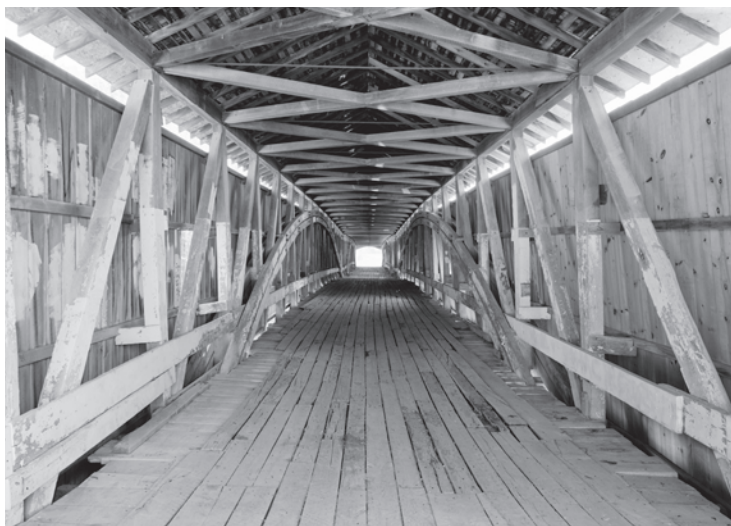
Figure 4.21 To transfer horizontal or lateral wind forces to the abutments, designers conceptualized and designed horizontal trusses and two-dimensional, or plane , frames as shown here. The horizontal trusses are at the plane of the floor and at the plane defined by the two top chords. For pony-type bridges, it was not possible to carry wind load and stabilize the top chord through a horizontal truss, so outriggers were installed. Examples of bracing include Top Left: 4.21a) horizontal lateral bracing to resist wind on the West Union Bridge (1876), Parke County, Indiana, HAER IN-105-13, James Rosenthal, photographer, 2004; Middle: 4.21b) Portal frames to transfer loads taken by the top chord on the Flint Bridge (1874), Orange County, Vermont, HAER VT-29-5, Jet Lowe, photographer, 2003; Bottom L: 4.21c) outriggers to stabilize top chords on the Beaverkill Bridge (1865), Sullivan County, New York, HAER NY-329-10, Jet Lowe, photographer, 2003.
