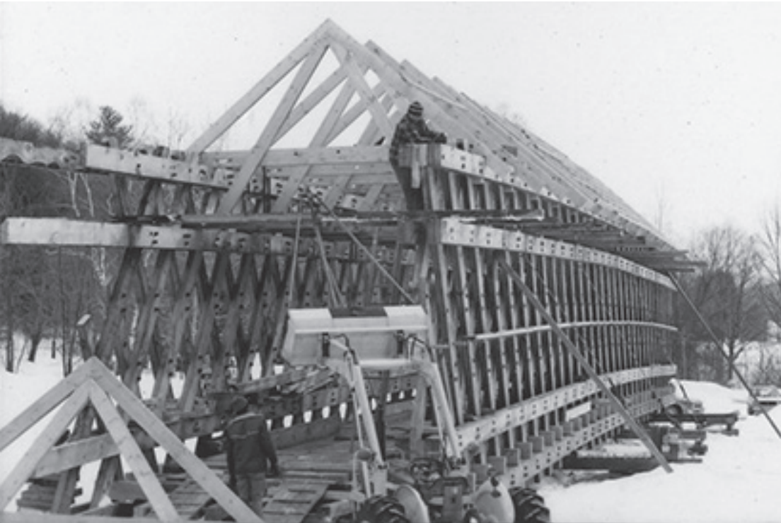
Figure 6.6 Arnold Graton erected a replacement for the Hall Bridge across Saxtons River in Windham County, Vermont, in 1982. Using traditional techniques, Graton Associates developed rough specifications from the original 1867 bridge and then framed it in a nearby field using traditional joinery and treenails. A team of oxen hauled the completed structure out across the river, and the bridge opened to traffic on September 6, 1982. Jack Peters, photographer, 1982. (See “Hall Bridge,” HAER VT-40 for additional information.)
