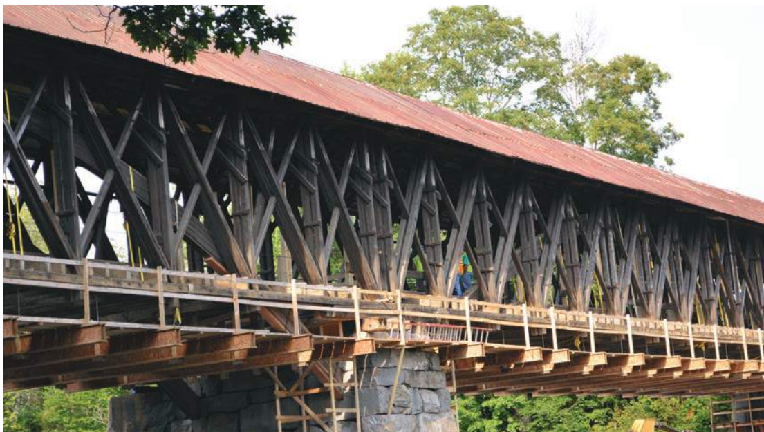
Figure 2.4 The rehabilitation of the Long truss on the Blair Bridge (1869) in Grafton, New Hampshire, required the use of staging, a technique discussed in the forthcoming “Guidebook for Restoring Structural Integrity of Covered Bridge Members.” Ron Anthony of Anthony & Associates, Inc., photographer, 2012.
