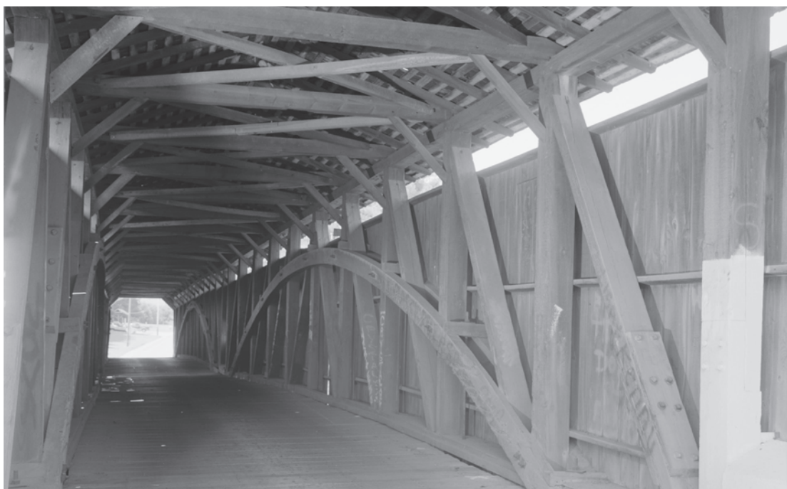
Figure 0.13 Pine Grove Bridge (1884) between Chester and Lancaster Counties, Pennsylvania, is one of eleven bridges by Elias McMellen that still stand. Although it has been rehabilitated, it still exhibits some of the finest examples of Burr-arch truss framing. HAER PA-586-7, Jet Lowe, photographer, 2002.
