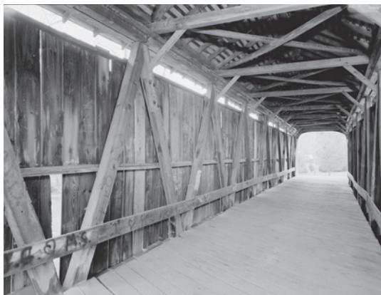
Figure 5.40 The 83-foot-long Salt Creek Bridge (1876) uses a single-web Smith truss with all inclined posts and braces in a single plane. HAER OH-127-9, Jet Lowe, photographer, 2004.
