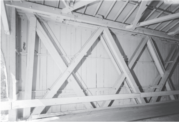
Figure 5.43 The Powder Works Bridge, built in 1872 by the Pacific Bridge Company, is a 180-foot Smith “triple truss” (Wilson type 4). One set of diagonals is sandwiched between and offset from two other sets of web members, connecting to four-piece chords. The image also shows the extra, inclined compression brace on the end panel, common to most Smith trusses (a block of wood obscures the notched joint). Note Smith-type castings fitted over notched joints in upper lateral braces. HAER CA-313-8, Jet Lowe, photographer, 2004.
