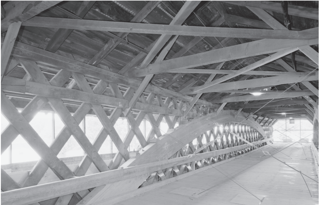
Figure 0.14 Built in 1829, the Bath-Haverhill Bridge in Grafton County, New Hampshire, is the oldest existing Town lattice bridge in the country. The laminated arches were added in 1922 to increase load capacity. HAER NH-33-14, Jet Lowe, photographer, 2003.
