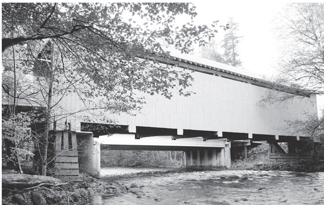
Figure 6.3 Top: 6.3a) The sides of the Howe trusses in Linn County, Oregon, as in Short Bridge (1945), were left open. HAER OR-120-6, Jet Lowe, photographer, 2004. Above: 6.3b) Covered bridges in Lane County, Oregon, like Horse Creek Bridge (1930, moved 1990), were covered nearly to the top chord. HAER OR-15-2, James Norman, photographer, 1987.
