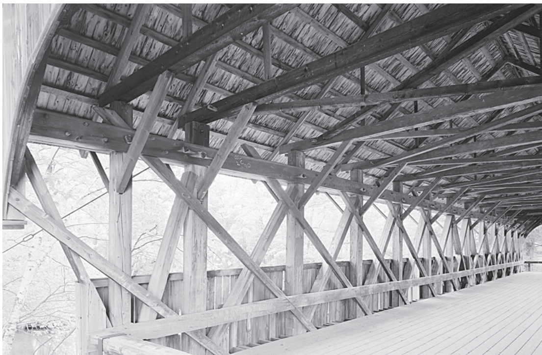
Figure 6.4 Sunday River Bridge (1872) in Oxford County, Maine, is a good example of the Paddleford truss, which became the dominant regional truss in parts of New Hampshire, Maine, and Vermont in the late-nineteenth century. HAER ME-69-11, Jet Lowe, photographer, 2003.
