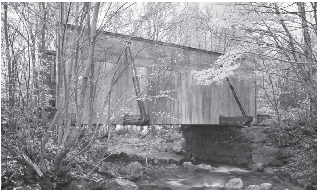
Figure 0.31 The 36-foot-long Snyder Brook Bridge (1918) in Coos County, New Hampshire, is a rare surviving Howe boxed pony truss (with supplemental outriggers), a once common bridge type built for short spans by the Boston and Maine Railroad. HAER NH-49-4, Jet Lowe, photographer, 2009.
