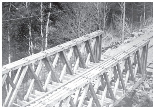
Figure 4.19 Historic examples of through, pony, and deck trusses include: Top Left: 4.19a) Dover Toll Bridge, a Howe through truss, carrying a train across Great Bay in Dover Point, New Hampshire, prior to being covered (stereograph by H. Copeland, 1873); Top Right: 4.19b) a Howe pony truss on the Portland and Ogdensburg Railroad in Crawford Notch through the White Mountains in New Hampshire (stereograph by B. W. Kilburn, ca. 1870); and Left: 4.19c) an uncovered Howe deck truss on the Troy and Greenfield Railroad (stereograph by Horton & Wise, undated). All stereograph halves courtesy of a private collection.
