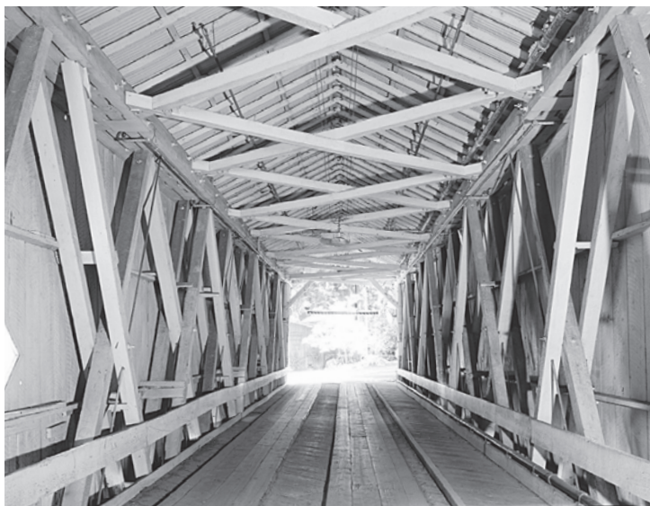
Figure 6.12 Powder Works Bridge (1872) in Santa Cruz Couty, California, is an excellent example of the early work of the Pacific Bridge Company and of the Smith type 4 triple-web truss. HAER CA-313-10, Jet Lowe, photographer, 2004.
