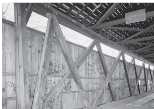
Figure 5.41 Kidd's Mill Bridge (1868) is a 122-foot-long Smith "double truss" (Wilson type 2). Note the steeply inclined extra brace at the end panel, with a lightning bolt shaped notch. HAER PA-622-5, Jet Lowe, photographer, 2006.
