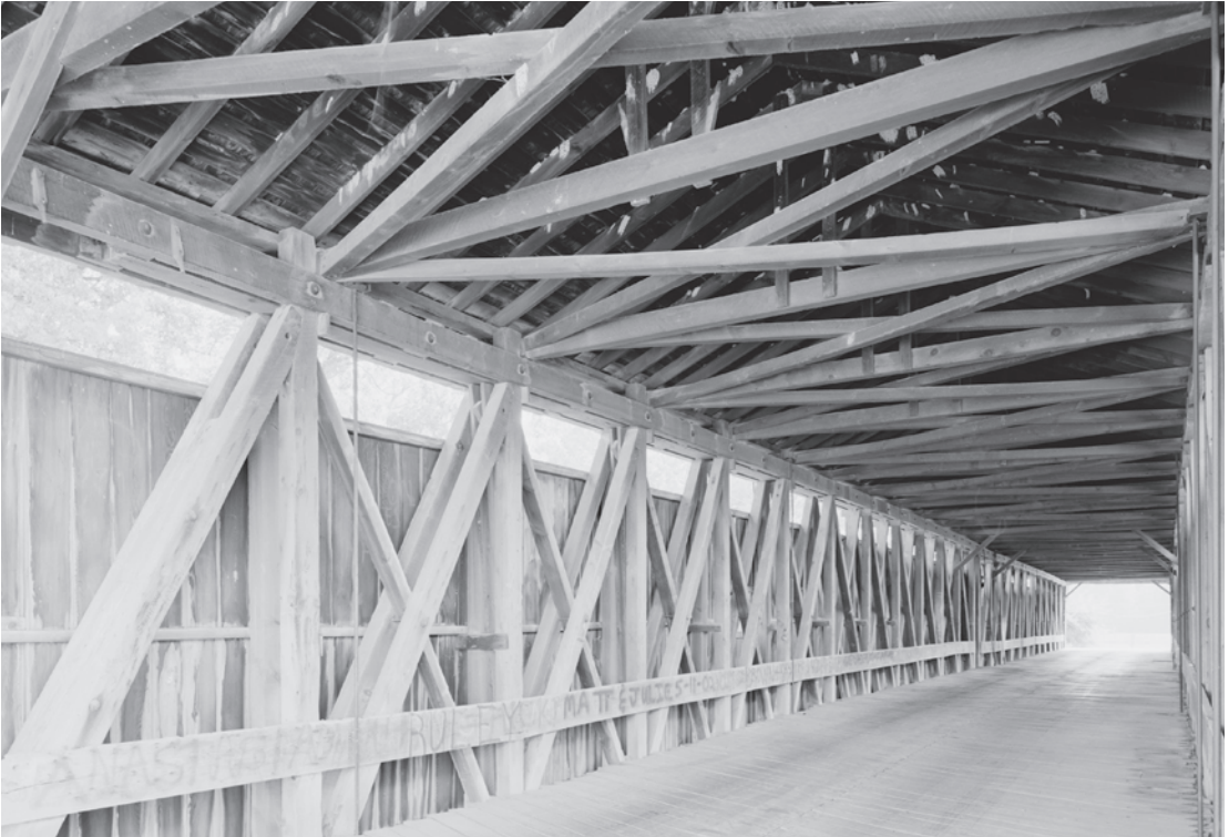
Figure 0.24 The Eldean Bridge (1860) in Miami County, Ohio, is one of the few remaining Long trusses that still retain their adjustable wooden wedges at the counterbrace panel points for prestressing. The designer of the truss, Col. Stephen Long, is credited with introducing mathematical theory to American bridge design. HAER OH-122-10, Jet Lowe, photographer, 2002.
