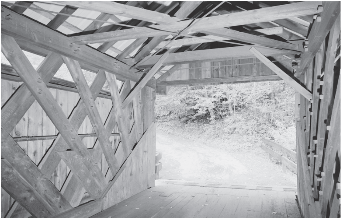
Figure 0.15 The Beaverkill Bridge (1865) is distinctive for its fan-like radiating planks at the ends of the lattice trusses. Carpenter John Davidson built this regional variation of the Town lattice in Sullivan County, New York, where two other examples survive from the 1860s. HAER NY-329-5, Jet Lowe, photographer, 2003.
