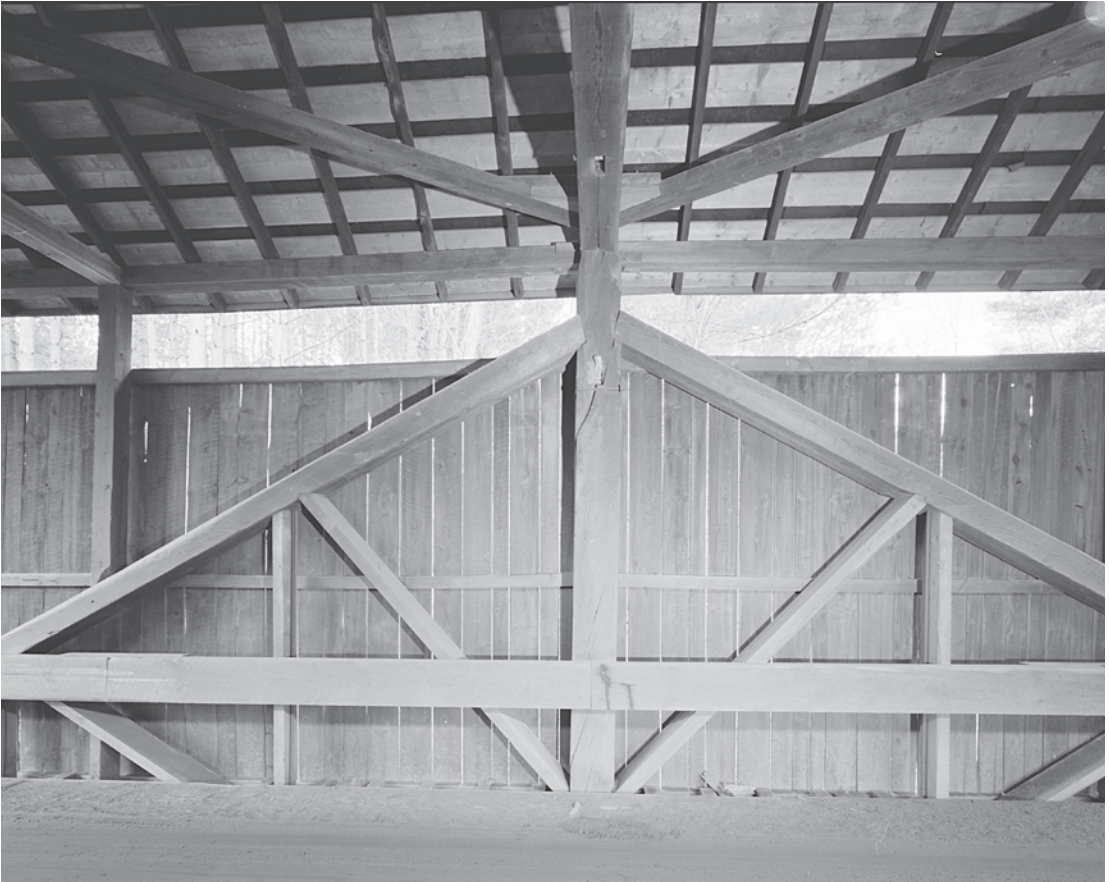
Figure 0.3 Pine Brook Bridge (1872) in Washington County, Vermont, is a 48-foot-long kingpost-truss bridge, rehabilitated by Milton Graton in 1977. The kingpost truss, a simple truss design commonly used for roof framing for centuries, was a common truss type sufficient for modest spans. There are only about twenty historic examples of kingpost-truss covered bridges remaining in the United States. HAER VT-37-8, Jet Lowe, photographer, 2006.
