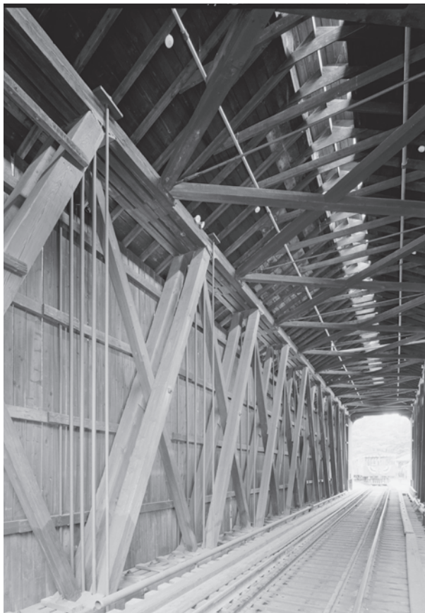
Figure 0.30 Clark's Railroad Bridge (1904) in Grafton County, New Hampshire, which was originally located upstate in Coos County on an important link on the granite-hauling Barre Branch Railroad, features substantial Howe trusses. Today it remains active on the steam excursion line at Clark's Trading Post. HAER NH-39-8, Jet Lowe, photographer, 2003.
