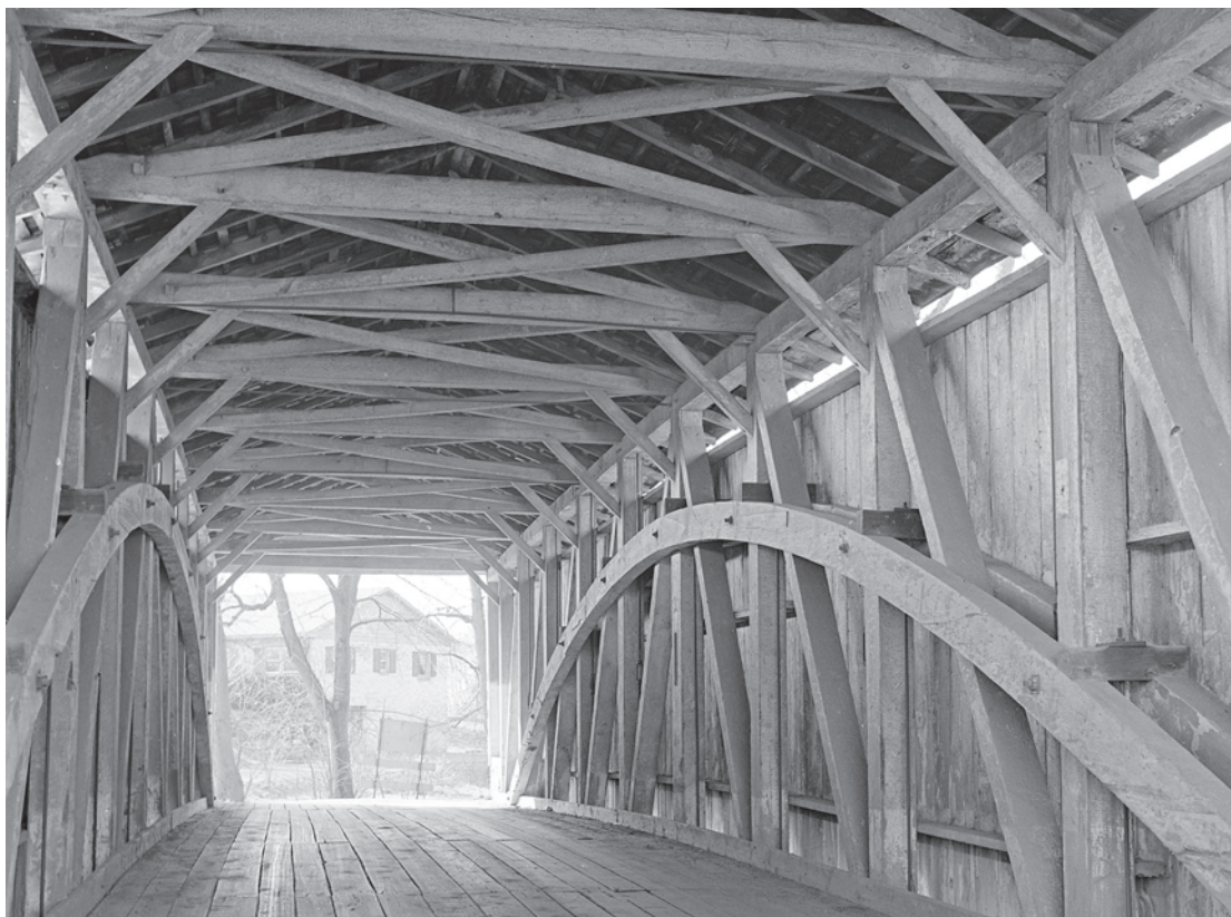
Figure 6.16 Elias McMellen's bridges, like the Kauffman's Distillery Bridge (1874) in Lancaster County, Pennsylvania, are known for their perfectly formed arches. Joseph Conwill, photographer, 1980.
