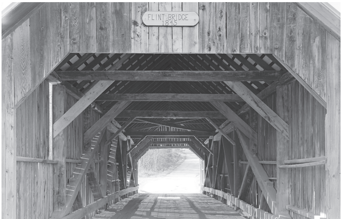
Figure 0.5 The Flint Bridge (1874) in scenic Orange County, Vermont, is a queenpost-truss bridge restored by Milton Graton in 1969. HAER VT-29-5, Jet Lowe, photographer, 2003.
