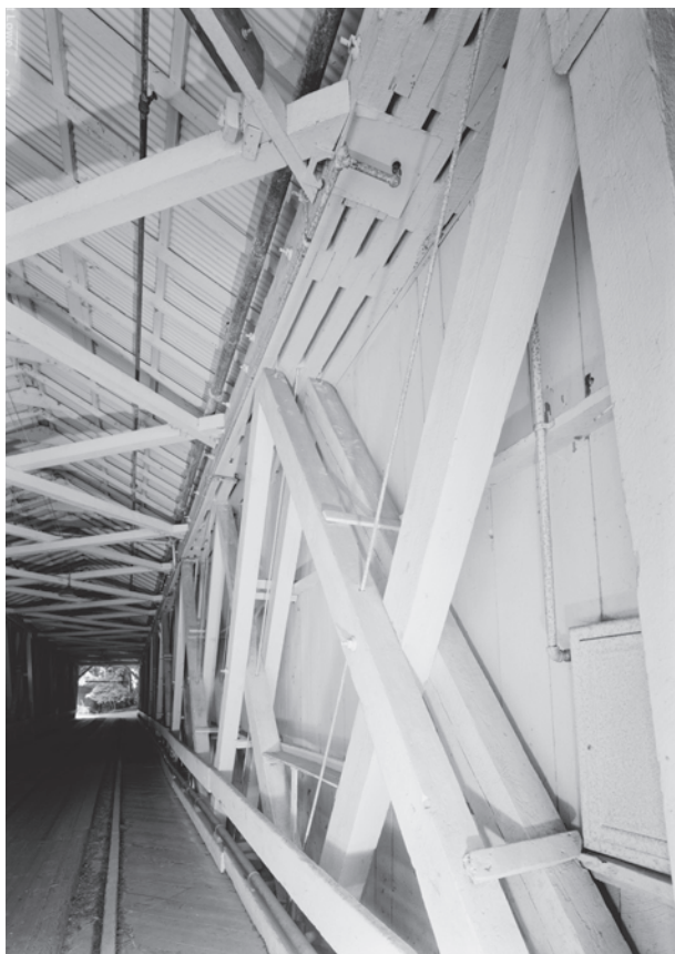
Figure 0.36 The Powder Works Bridge (1872) in Santa Cruz County, California, is a triple-web Smith truss built by William Gorrill's Pacific Bridge Company, which introduced the Smith patent to the northwestern part of the country and built several wooden bridges in California and Oregon in the 1870s. HAER CA-313-9, Jet Lowe, photographer, 2004.
