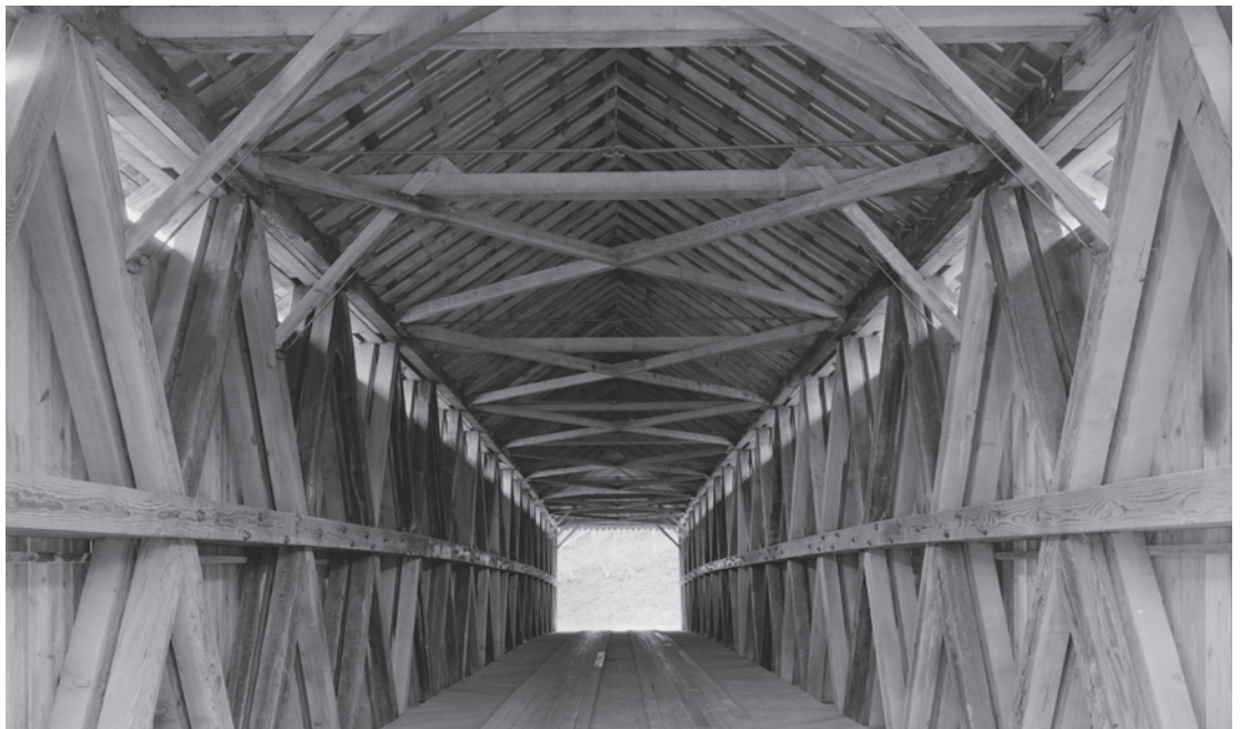
Figure 0.45 The Bennett's Mill Bridge (1875) in Greenup County, Kentucky, was the sole surviving historic Wheeler truss until it was rebuilt in 2004. Isaac Wheeler's truss design, featuring paired tension members, double-offset compression members, and an intermediate chord, was briefly popular in the Sciotovalle, Ohio, area from 1870 to 1875. HAER KY-49-9, Jet Lowe, photographer, 2004.
