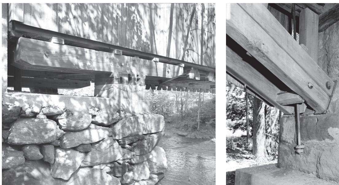
Figure 4.28 Examples of bolster beams and skewbacks. Left: 4.28a) Bolster beam detail on Hall Bridge, Windham County, Vermont, installed by Graton Associates in 1982. HAER VT-40-7, Jet Lowe, photographer, 2009. Right: 4.28b) Cast-iron skewback and rod tying the Burr arch into the limestone abutment of J. J. Daniels's West Union Bridge (1876), Parke County, Indiana. The arches bear on an inclined bearing surface called a skewback. HAER IN-105-11, James Rosenthal, photographer, 2004.
