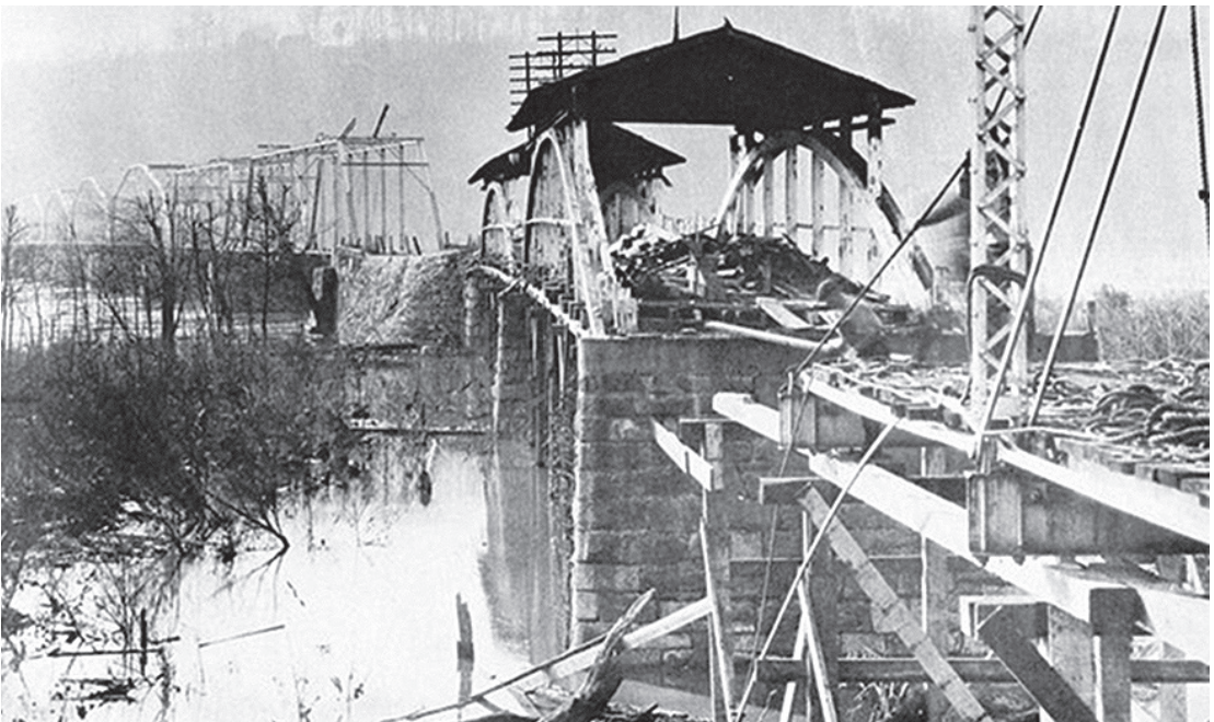
Figure 7.2 Built in 1859, the ten-span Conowingo Bridge crossed the Susquehanna River in Maryland. This photograph from ca. 1925 shows the new steel trusses being constructed in the background while the original wooden Burr-arch trusses are being dismantled. Courtesy of Richard Sanders Allen Collection, National Society for the Preservation of Covered Bridges.
