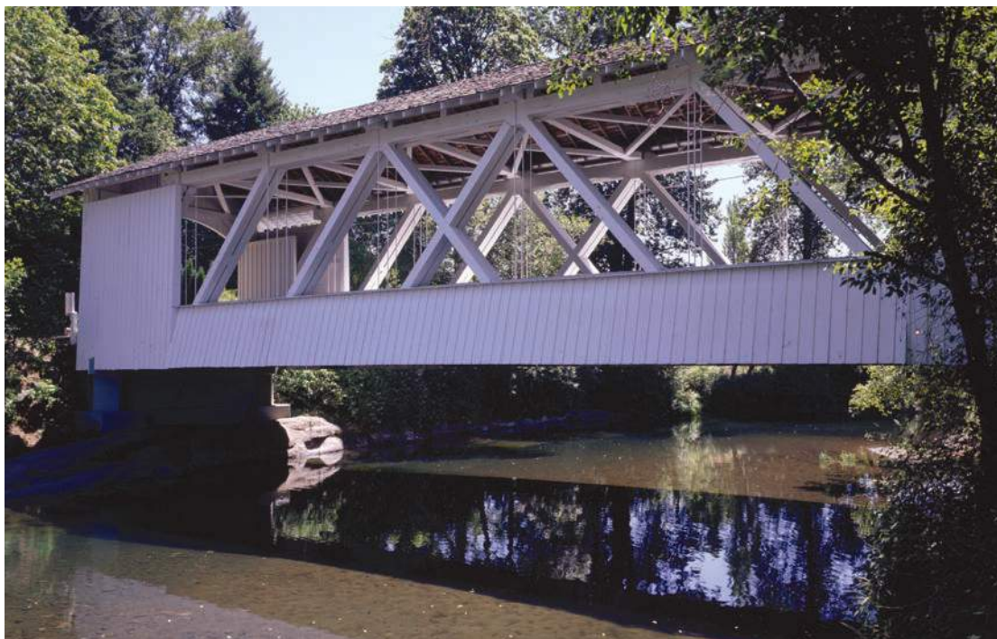
Figure 3.23 Built by the Linn County Engineering Department in 1941, Larwood Bridge is one of the best surviving examples of Oregon's standard-plan Howe trusses. HAER OR-124-13, Jet Lowe, photographer, 2004.
