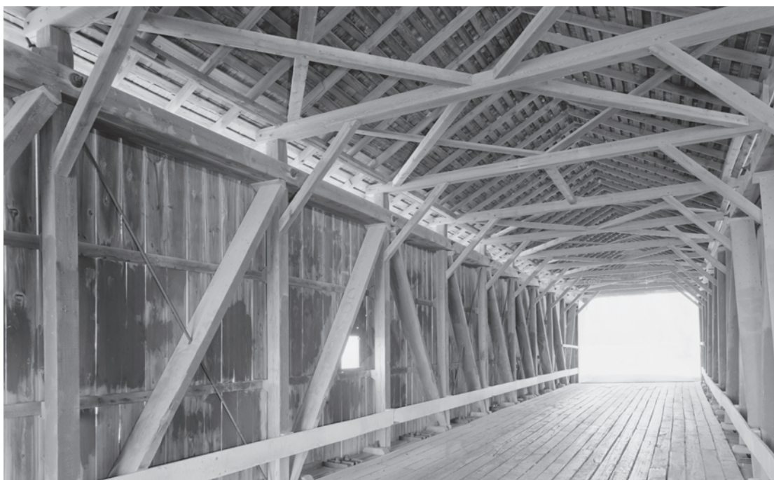
Figure 0.41 Harshman Bridge (1894) is one of seven surviving Childs trusses built by Everett Sherman in Preble County, Ohio, in the 1880s and 1890s. Horace Childs, a nephew and agent of Stephen Long, patented the design in 1846. HAER OH-126-10, Jet Lowe, photographer, 2004.
