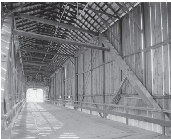
Figure 5.37 A 128-foot-long Pratt truss can be found in the center span of the Honey Run Bridge (ca. 1886), Butte County, California. HAER CA-312-5, Jet Lowe, photographer, 2004.
