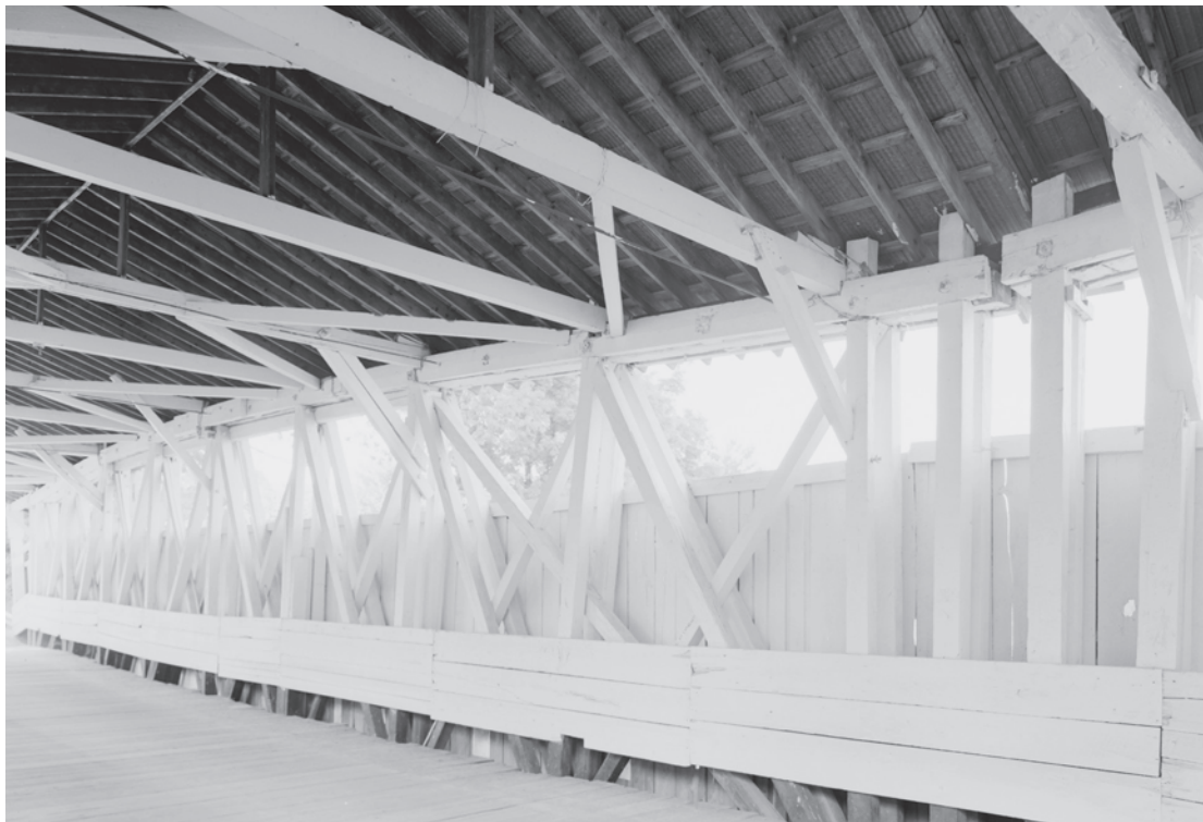
Figure 0.40 Patented by Daniel McCallum in 1851, the McCallum truss featured an arched upper chord and prestressed counterbraces and was used on North American railroads during the 1860s. The Powerscourt Bridge (1861), crossing the Chateauguay River in Huntingdon County, Quebec, is the only surviving example of this truss type. HAER NY-332-8, Jet Lowe, photographer, 2003.
