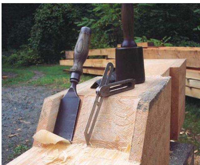
Figure 6.22 Top: 6.22a) The work done by Tim Andrews during the rehabilitation of Gilpin's Falls Covered Bridge in Cecil County, Maryland, carefully ensured the preservation of historic details. Above: 6.22b) Traditional timber-framing tools used in carving out the step in a vertical post on the Gilpin's Falls project include (left to right): a framing chisel, a corner chisel, a ca. 1930 line bevel, and a urethane carver's mallet. Will Truax, photographer, 2009
