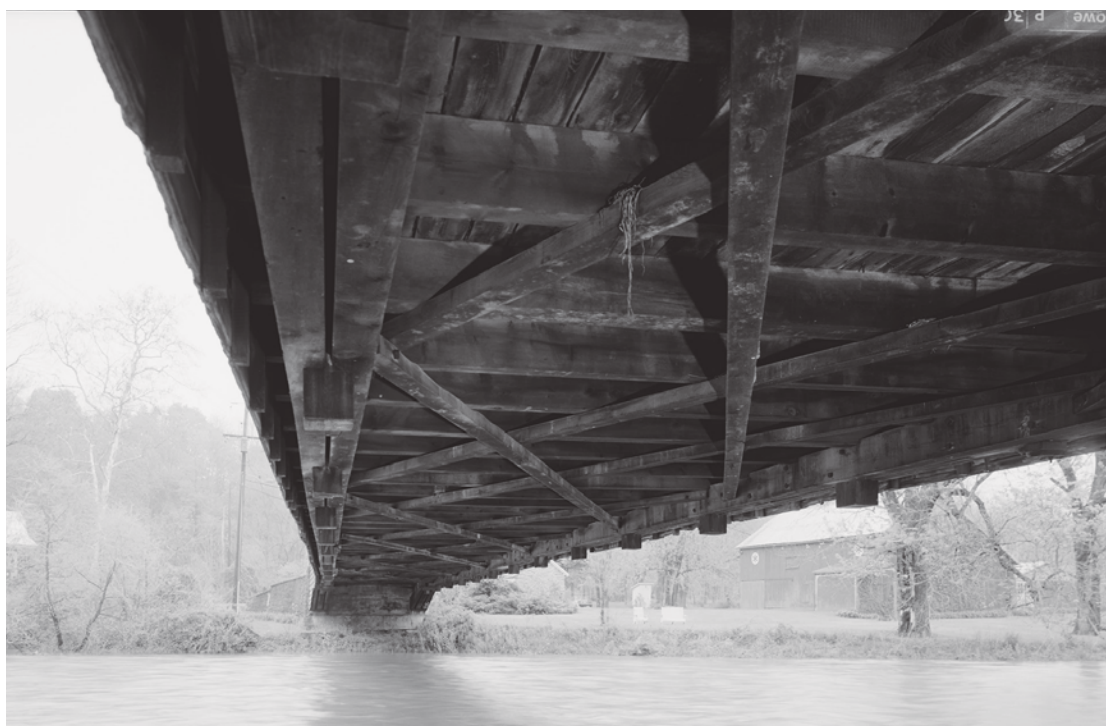
Figure 6.2 Top: 6.2a) Pine Grove Bridge (1884) once illustrated the general pattern of X-braced floor framing found in covered bridges in Lancaster County, Pennsylvania. Since the decking and stone abutments have been replaced by steel beams and concrete, these floor details no longer exist. HAER PA-586-2, Jet Lowe, photographer, 2002. Above: 6.2b) On the other hand, Dreibelbis Station Bridge (1869) retains the three-panel-long latticed style floor framing typical of covered bridges erected in Berks County, Pennsylvania. HAER PA-587-7, Jet Lowe, photographer, 2002.
