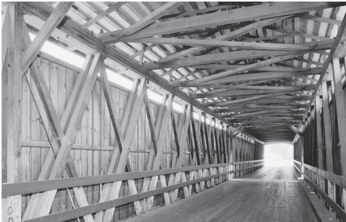
Figure 0.26 Knight's Ferry Bridge (1863) in Stanislaus County, California, is a 379-foot-long, four-span Howe truss built as a major crossing on the Stockton to Sonora Road. Its high integrity as one of the best remaining examples of a wood and iron Howe truss contributed to its designation as a National Historic Landmark in 2012. HAER CA-314-8, Jet Lowe, photographer, 2004.
