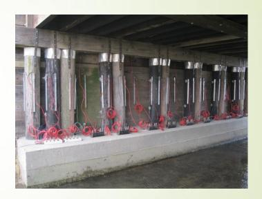
Abutment piles and backwall encapsulated by additional planking and concrete infill
