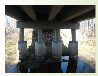
Corrugated metal pipe used as concrete form to encapsulate deteriorated timber pile
