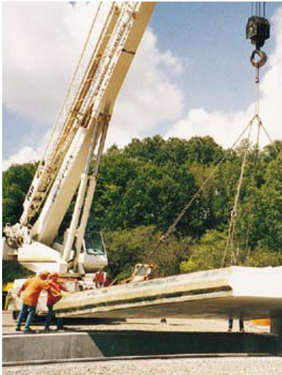
New prefab bridge panel 50 feet long x 20 feet wide
