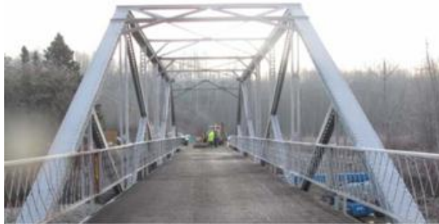
Bridge paved with HL4 Asphalt
