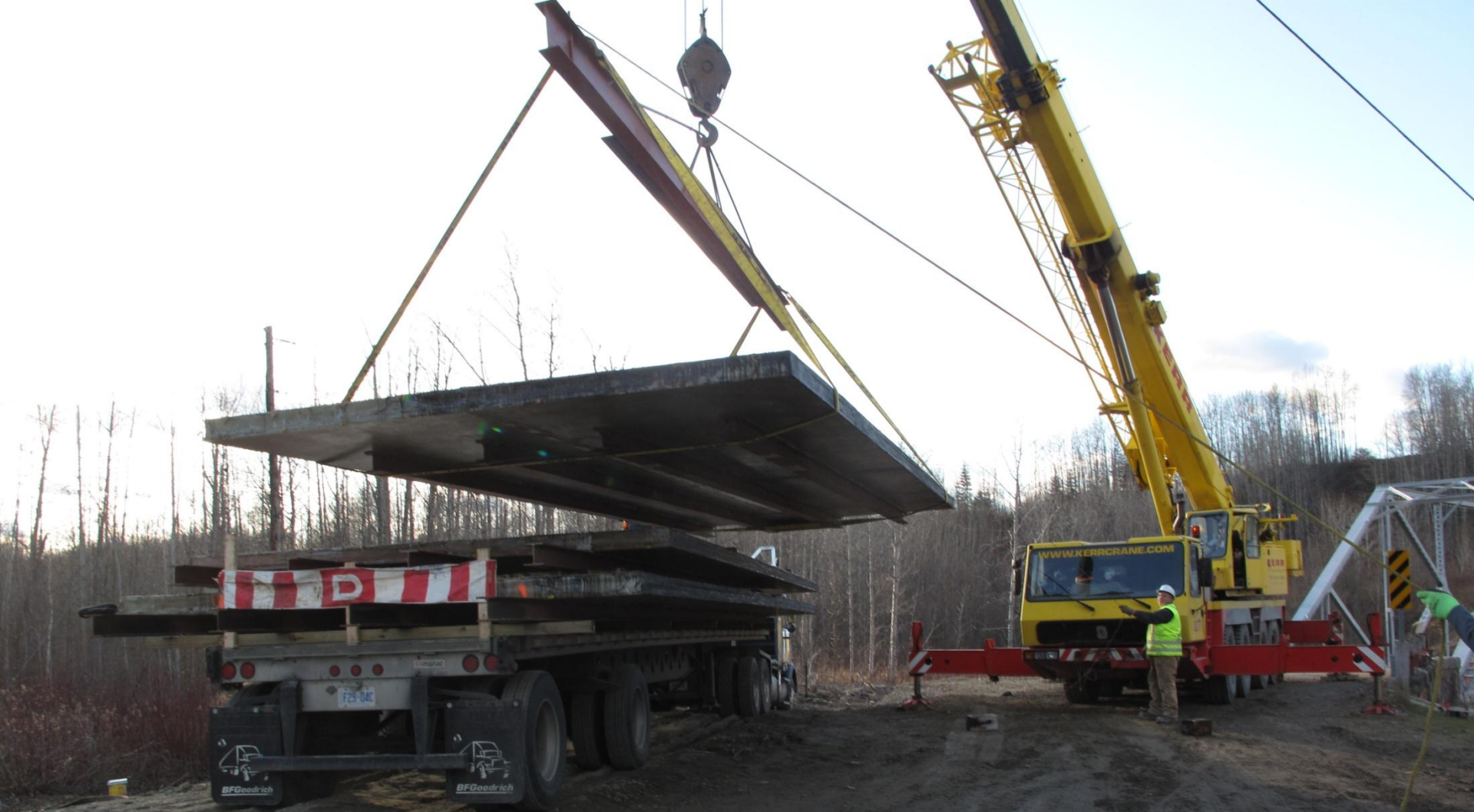
3 Prefabricated bridge decks Removed by crane
