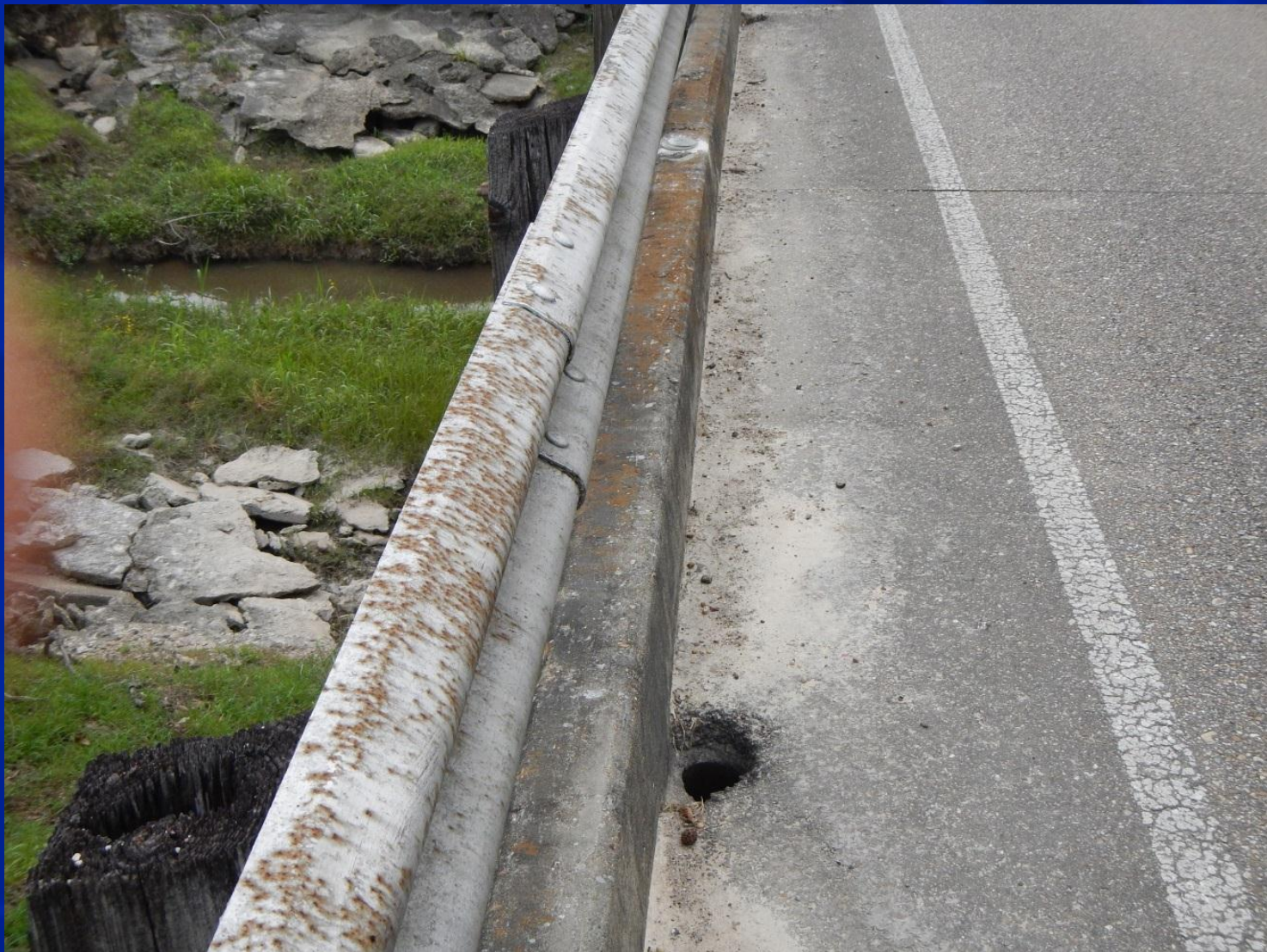
Bridge 62-2, Drains in Concrete Deck
