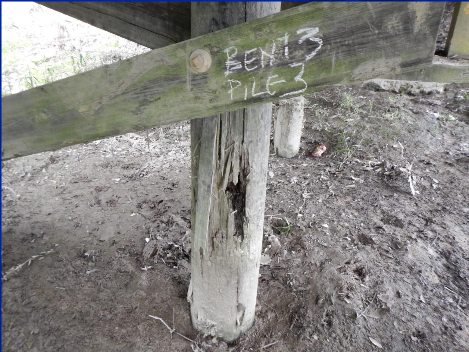
Bridge 62-1, Decayed Pile
