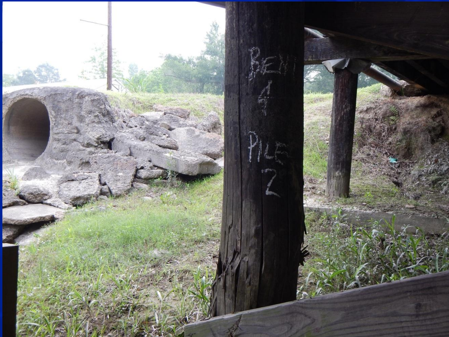
Bridge 62-2, Damaged Pile
