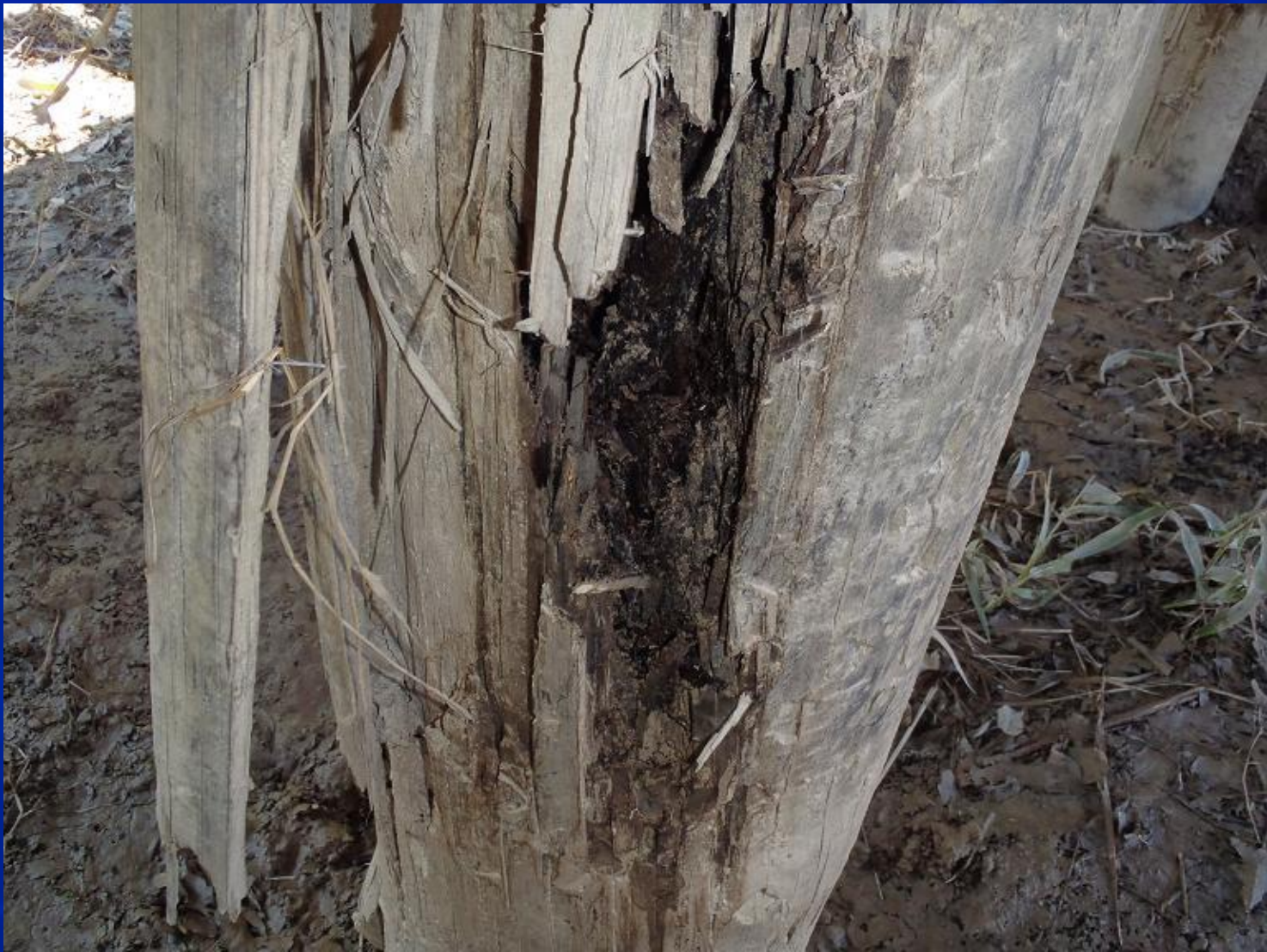
Bridge 62-2, Pile Damage
