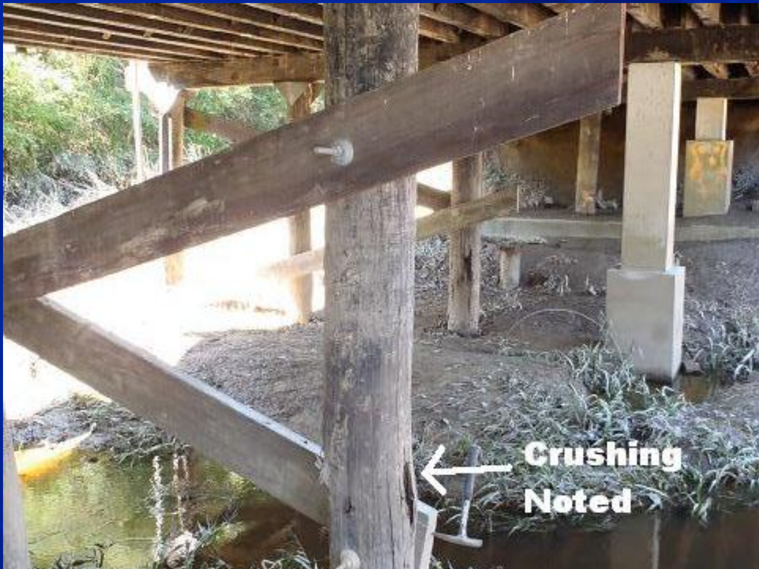
Bridge 62-1, Pile Damage
