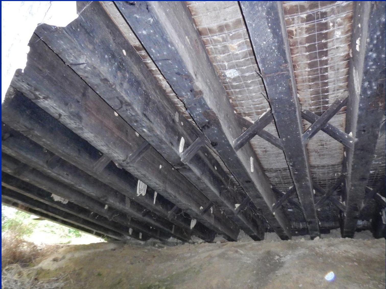
Bridge 62-2, View of Concrete Deck and Stringer Bracking
