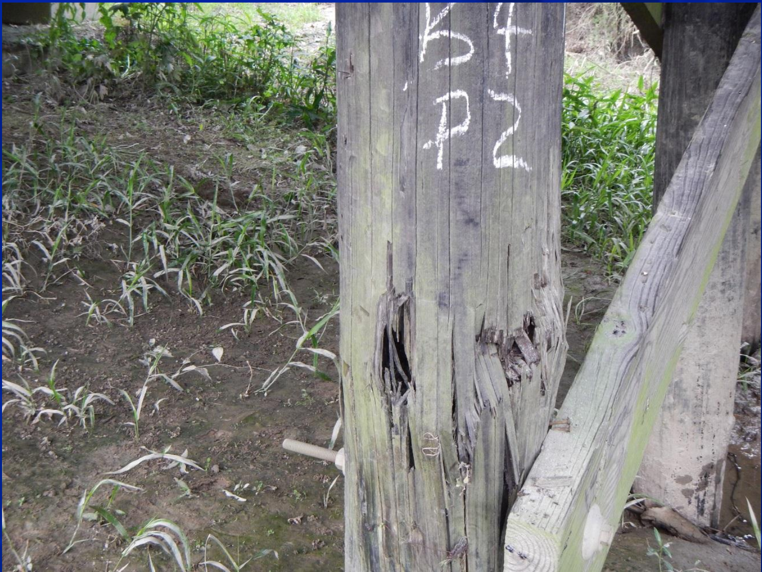
Bridge 62-2, Pile Damage
