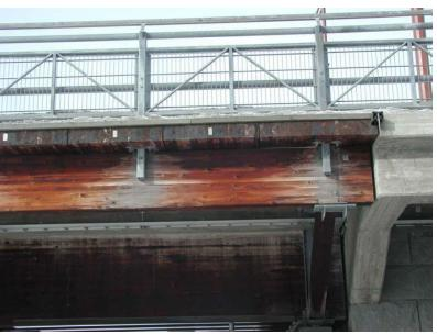
The outer surface of the utmost beam at the end of the bridge is similarly blotchy at railing pole positions
