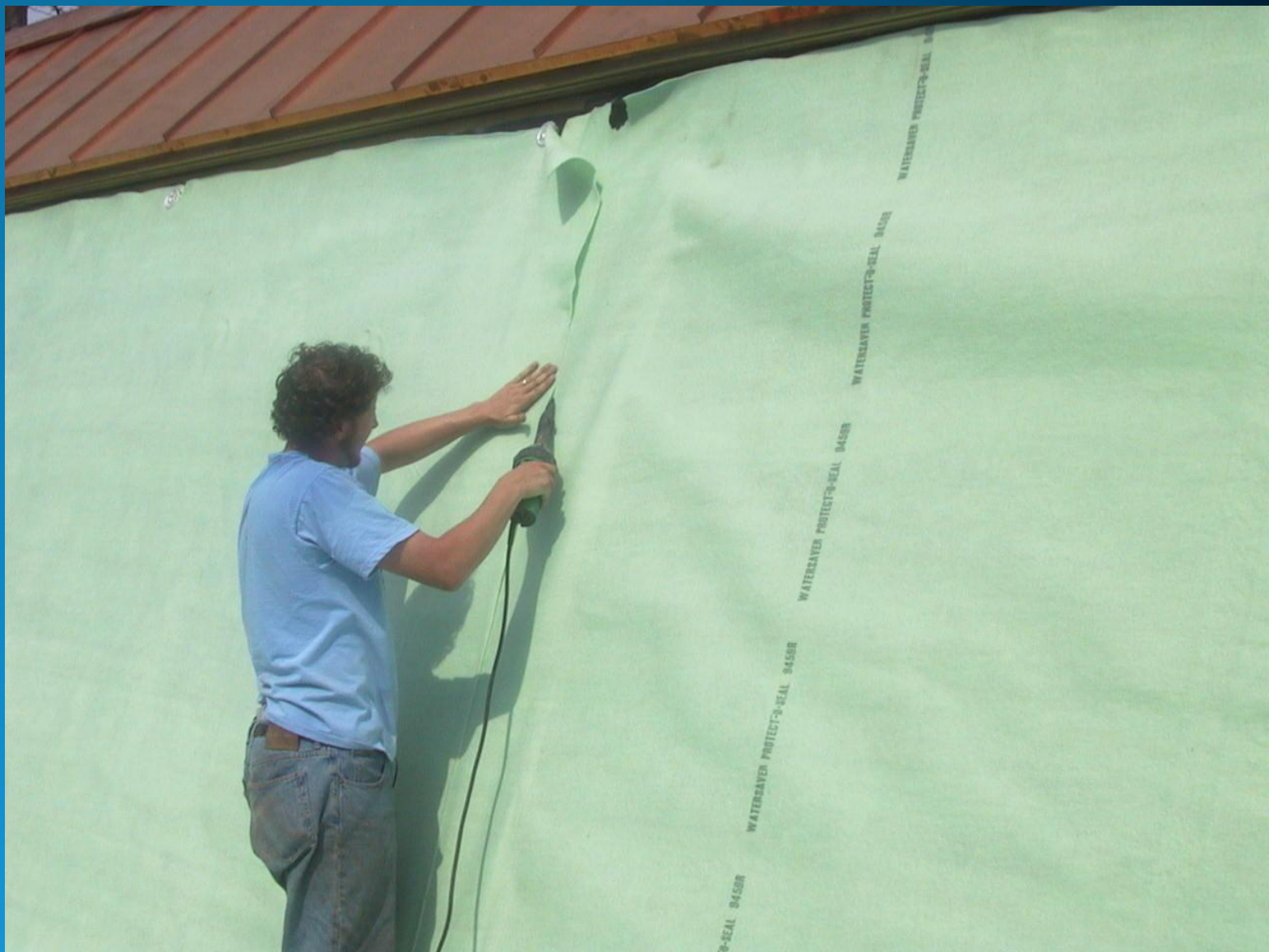
Detail – trunk liner system – welding seams
