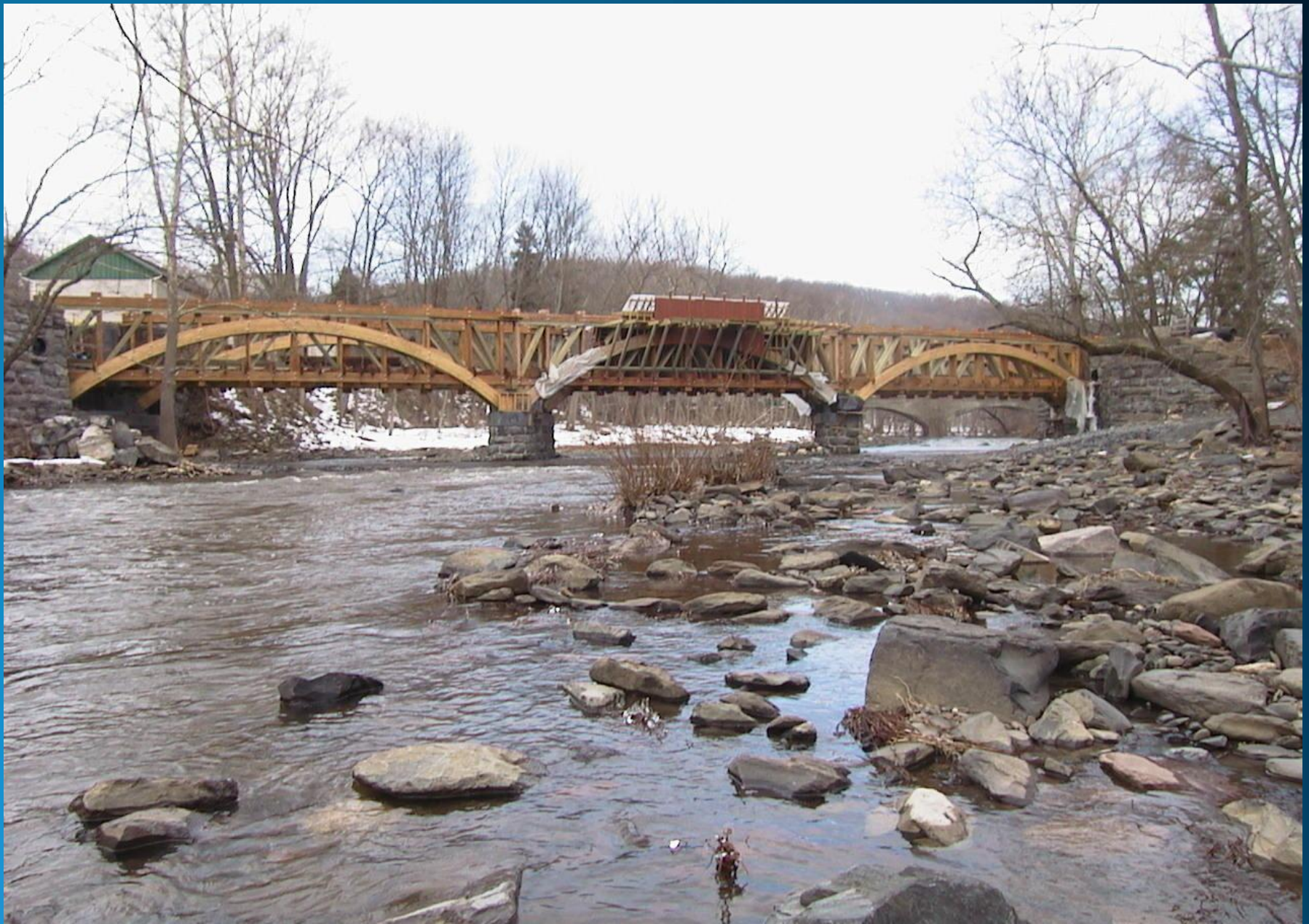
New superstructure on rehabilitated substructures
