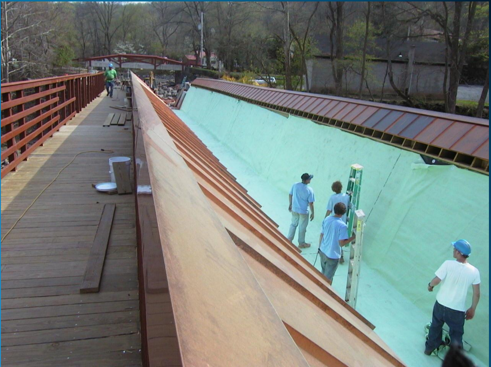
Detail – trunk liner system (ultimately modified)
