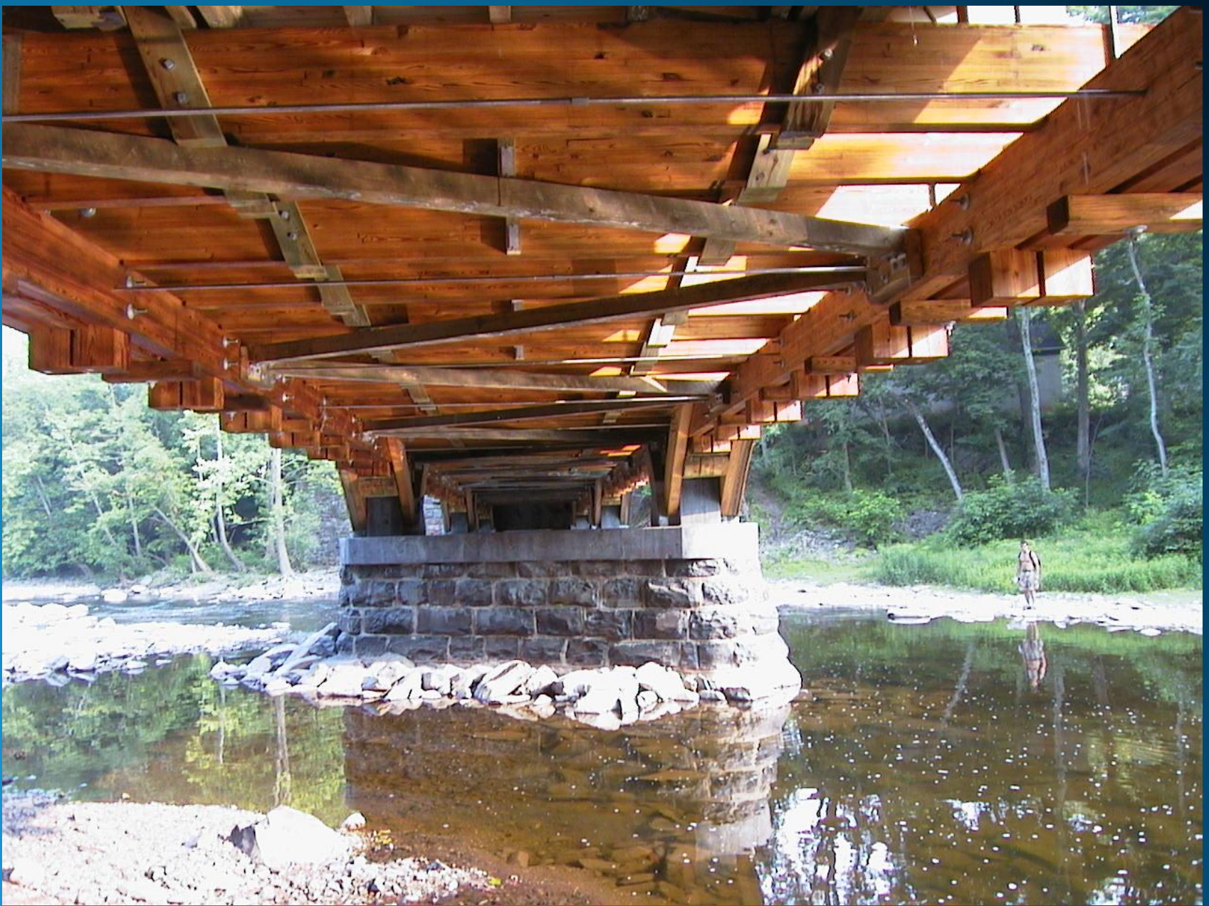
Detail – FRPs were applied to transverse beams
