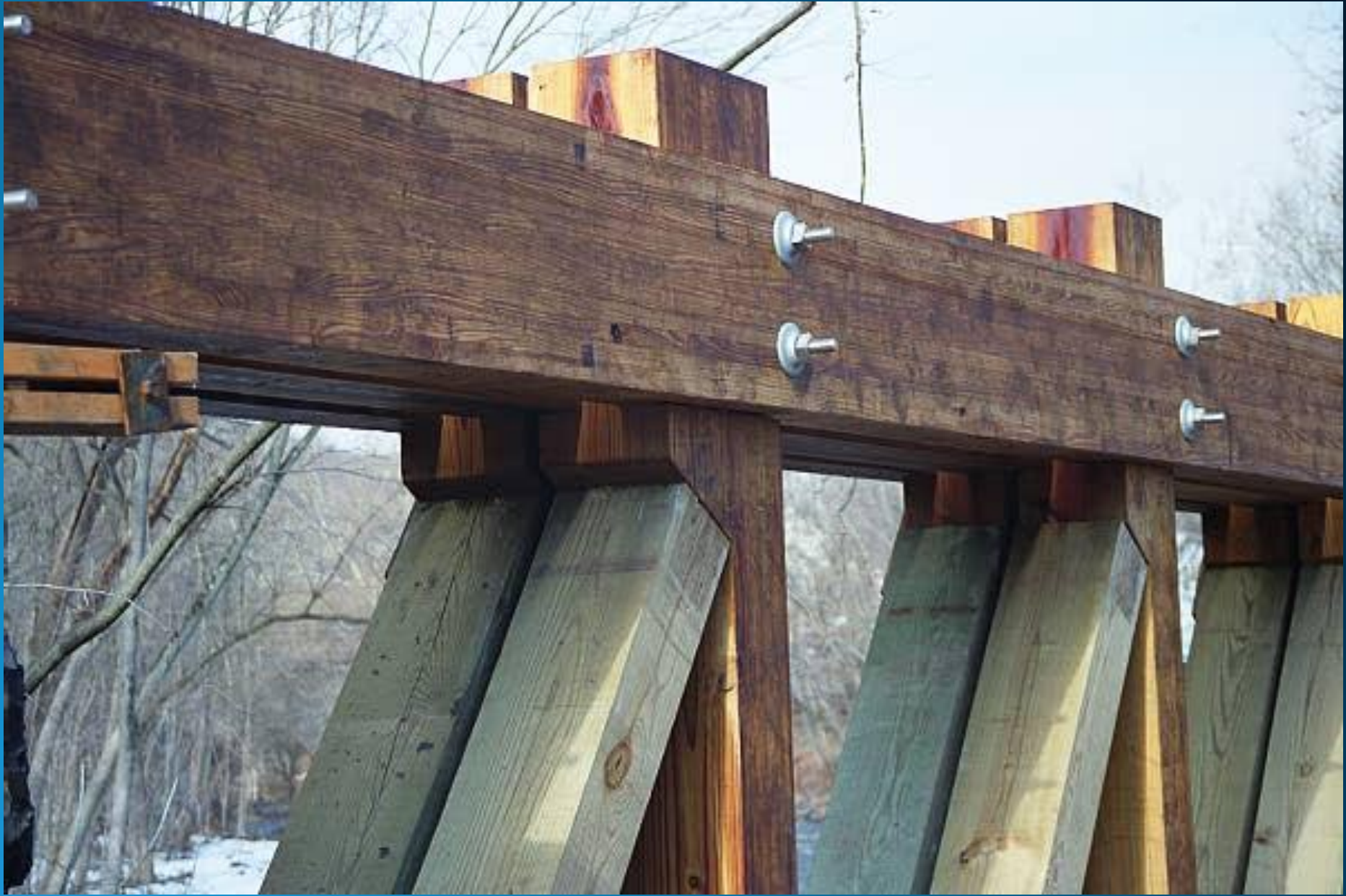
Detail – upper truss chord
