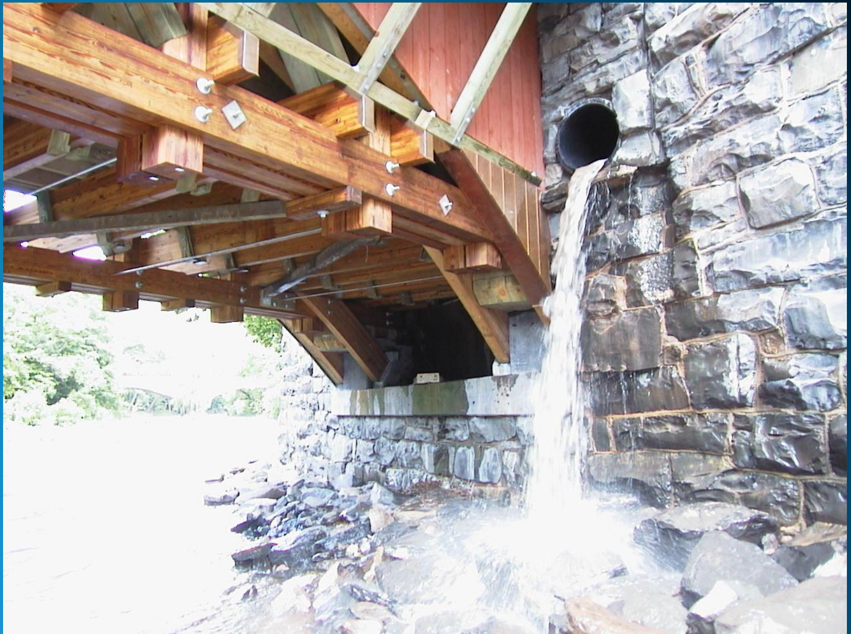
Detail – Bearing at north abutment
