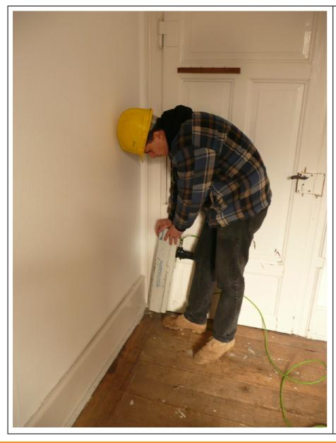
Locating 'hidden' beams and assessing their condition with resistance drilling without taking off the floor (or stucco).
