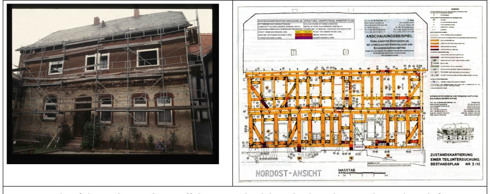
Historic building (1652): wall beams hidden behind wooden shindels and/or bricks => resistance drilling was used for locating beams and assessing their condition.
