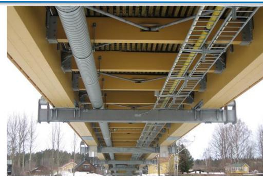
The total amount of glulam is almost 400 m<sup>3</sup> or 200 tonnes. There are also 80 tonnes of steel in the form of castings and fixtures of different kinds
