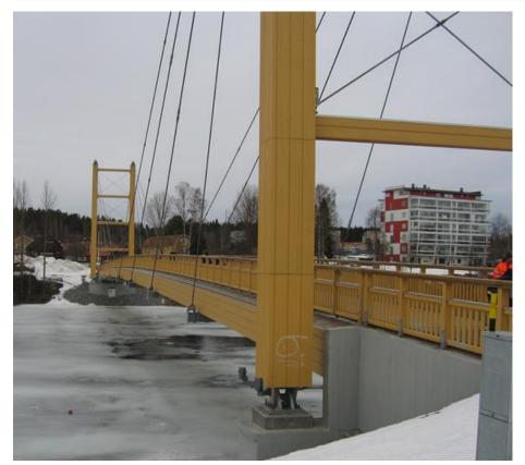
Free span: 130 meters (426 ft.) and very slender with a width of only 4 meters
