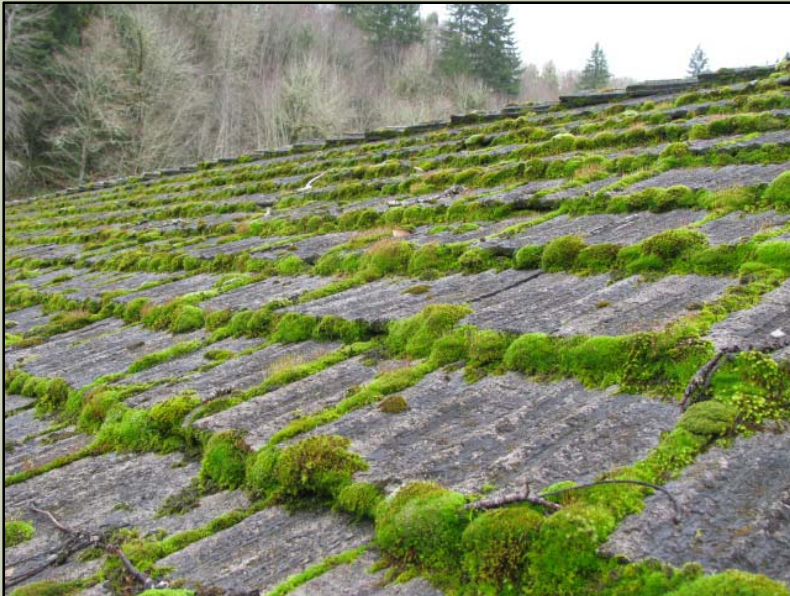
Very heavy cement/wood fiber composite roofing was leaking
