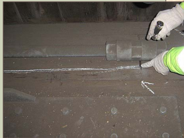
Broken splices leaving gaps to \frac{1}{2} "
