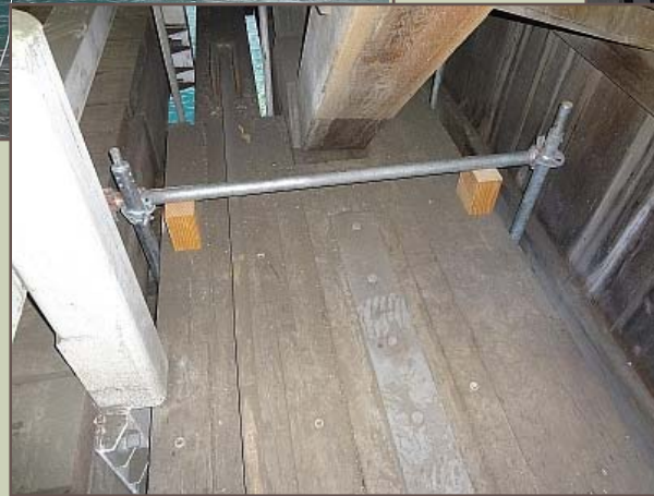
Suspended from truss bottom chords
