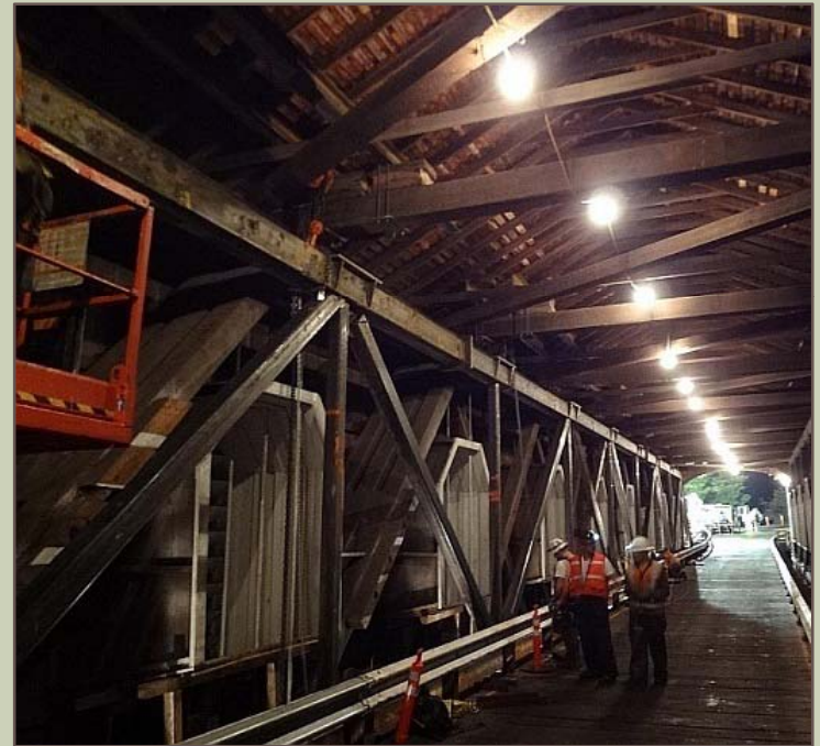
Temporary rail in place Ready for traffic
