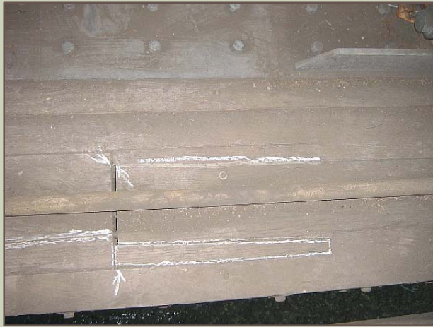
Broken splices leaving gaps to \frac{1}{2} "
