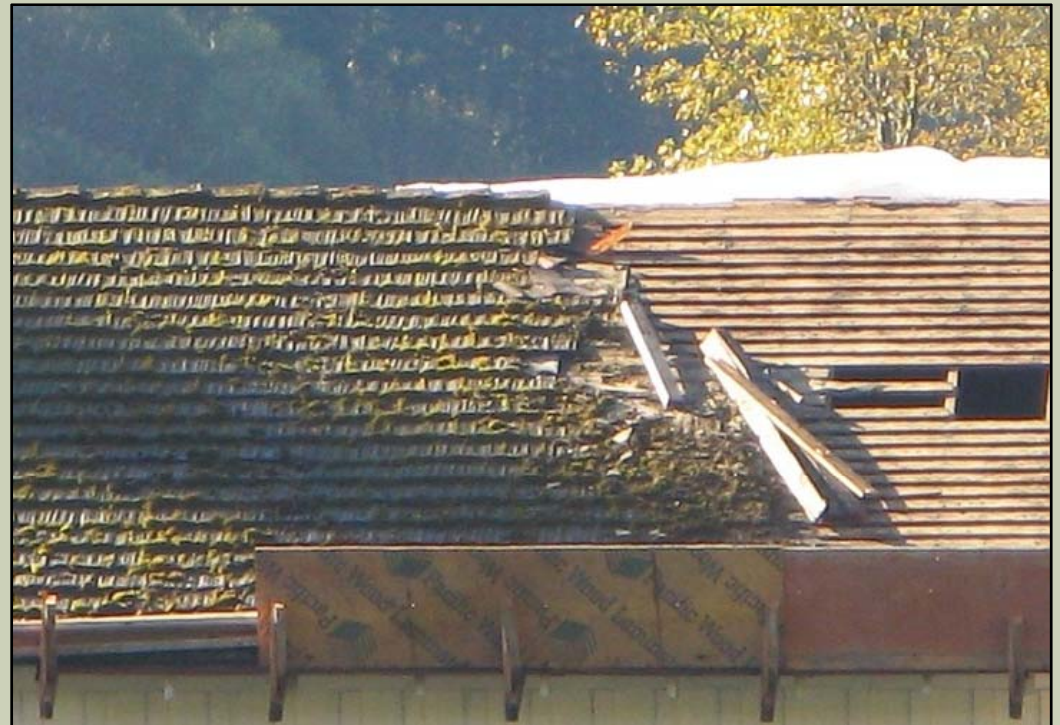
Replaced with much lighter and historically more appropriate cedar shingles
