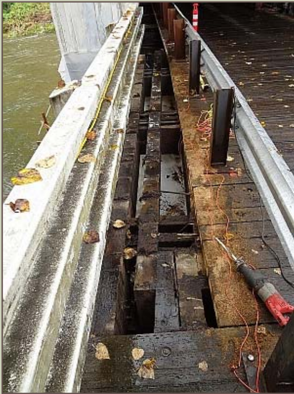
Temporary rail installed and deck cut
