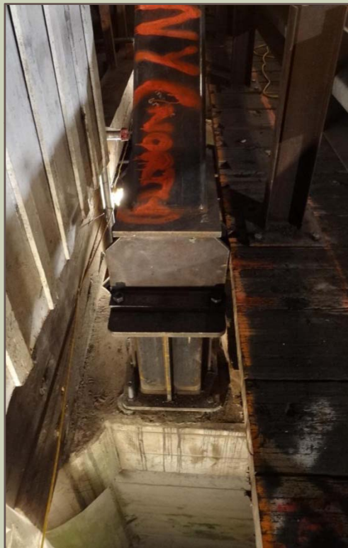
Bearing on concrete pier
