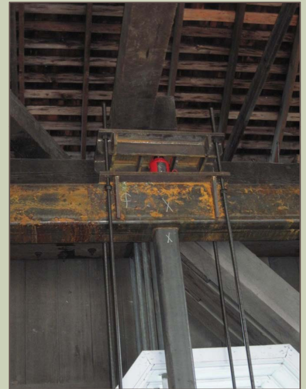
One of 20 50-ton hydraulic jacks
