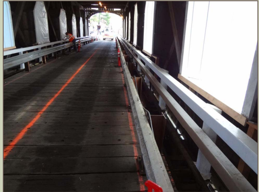
Reinstalling bridge rail
