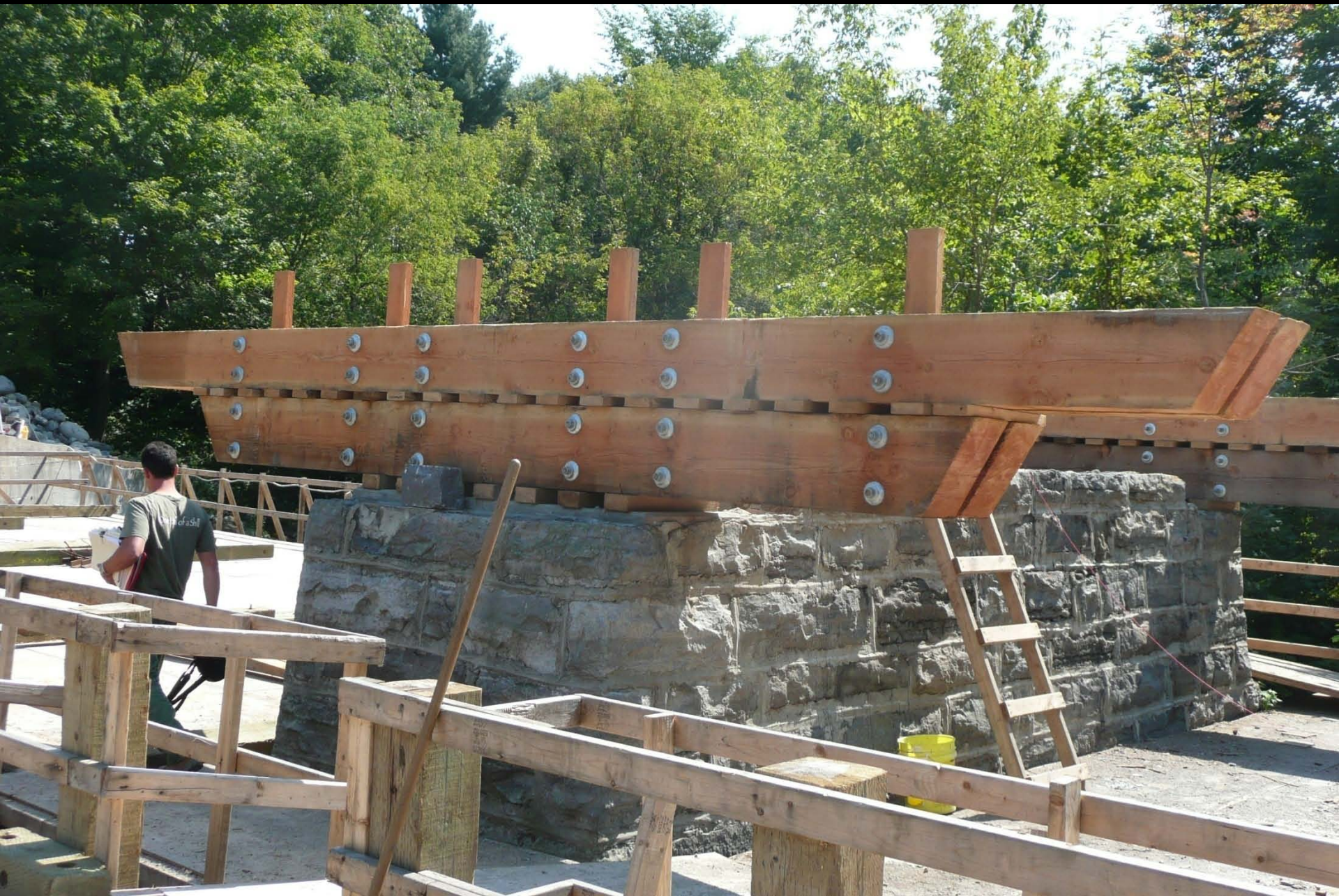
New bolster beams at central pier, 2009
