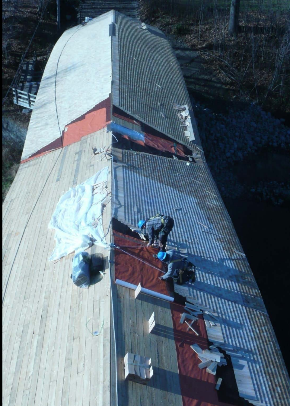
Laying cedar shingles over membrane and cedar breather
