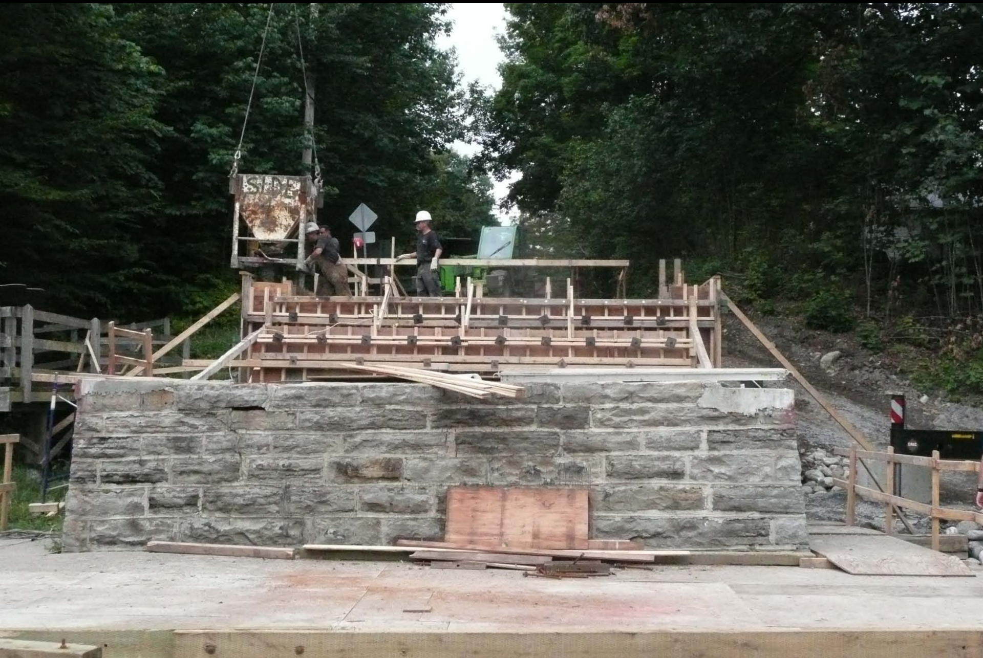
Rebuilding west abutment, Supplementary 1960s pier in foreground
