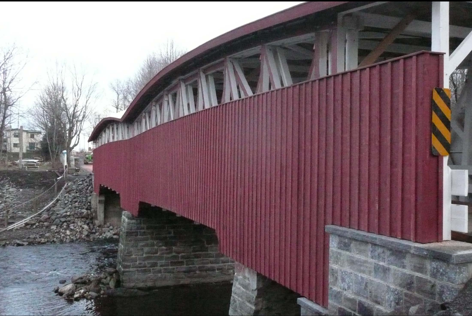
Stone faced abutment side wall
