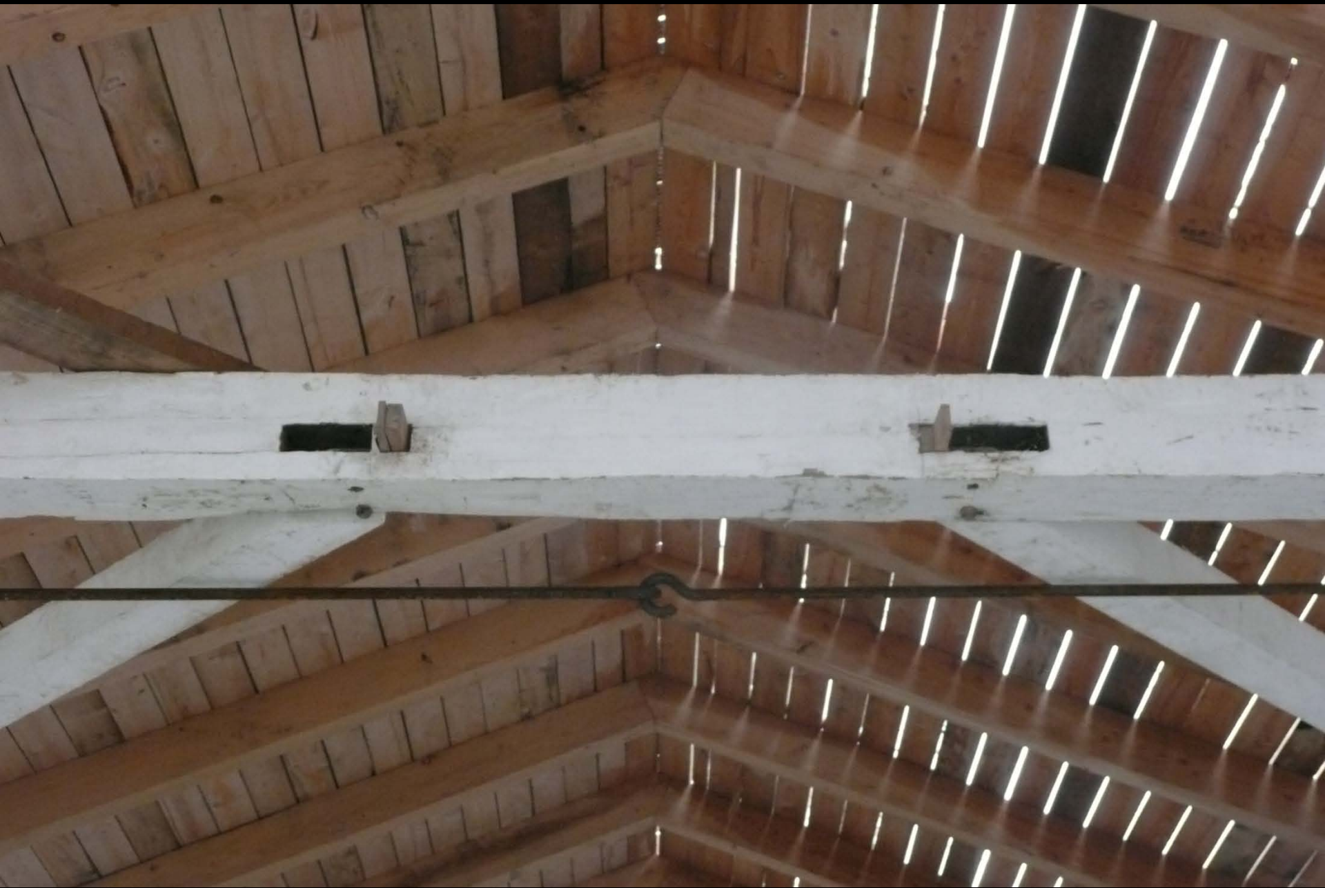
Modified roof structure with former tie rod
