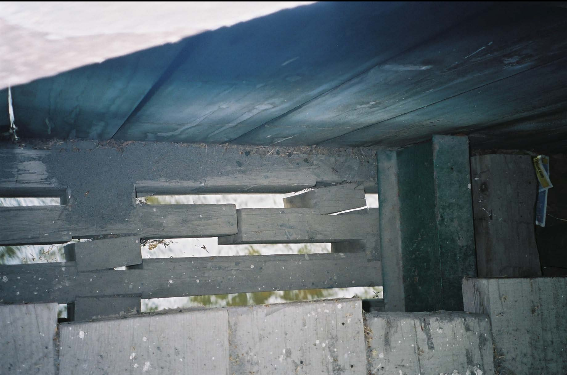
Rotating shear keys in lower chord, 2007
