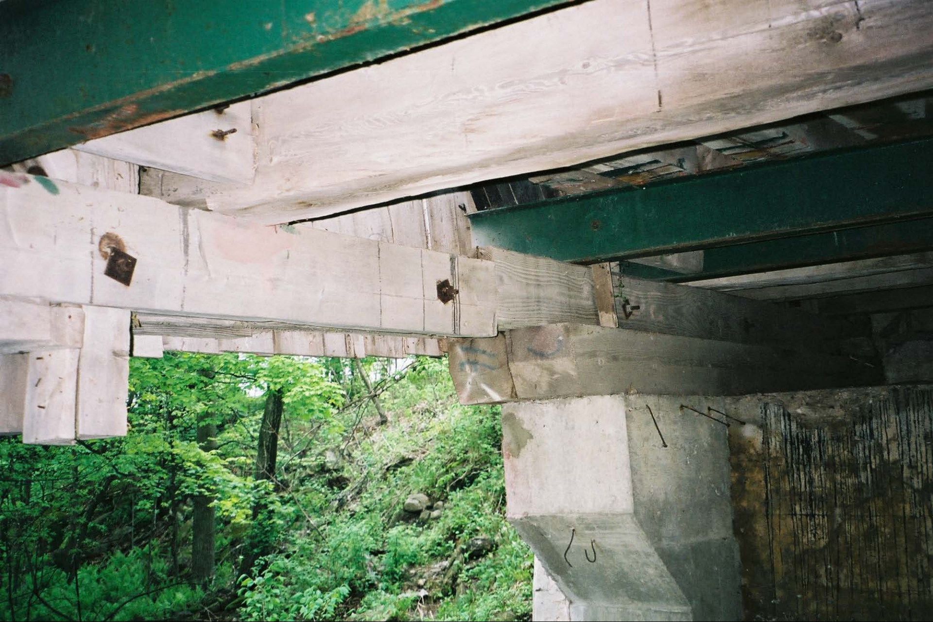
Slipped joint (poorly located) in lower chord, 2007. (Steel floor beams inserted in 1980s.)
