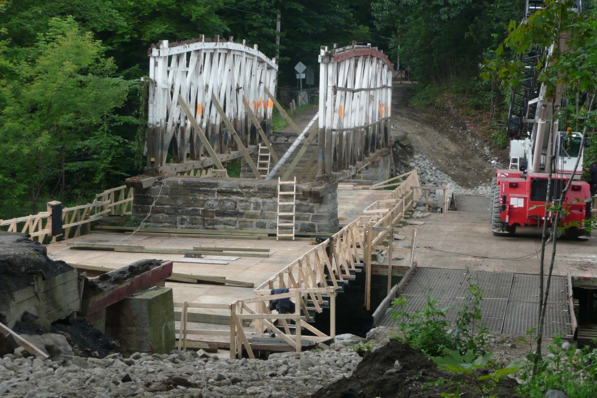
East span removed; note lack of containment road materials at east abutment
