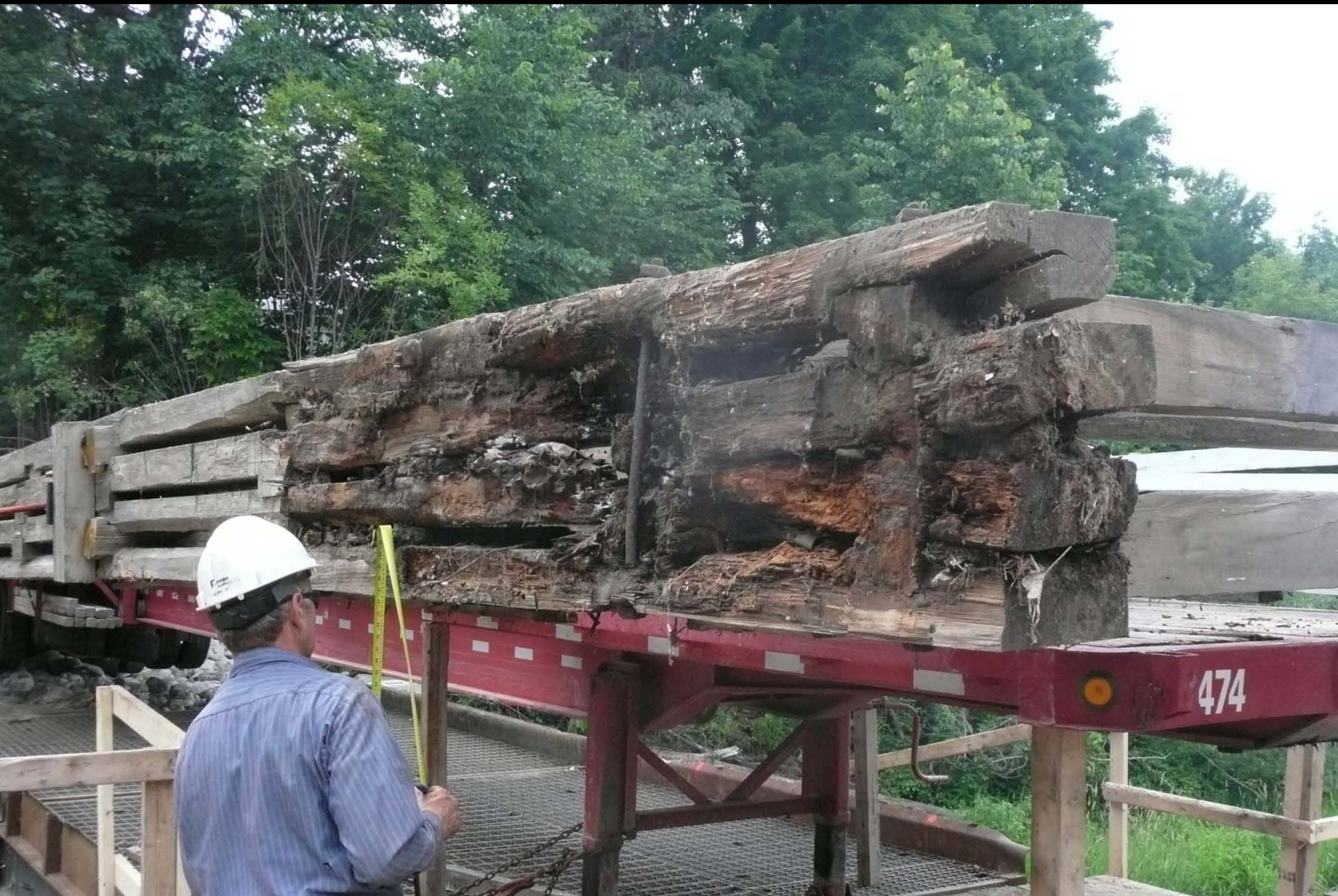
Deteriorated bottom chords at east abutment, 2009
