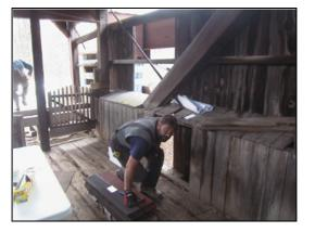
Fig. 2 Human and livestock gates at east portal. Note the diagonal repair rods through the truss braces, which were installed early in the twentieth
