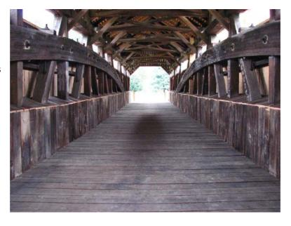
Rough-hewn cedar shingles were installed to the lath. Most of the siding was replaced in-kind, with some reused as battens. The wainscoting and cap material was stockpiled and then reinstalled.
