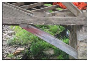
Fig. 6: Arch "tied" to chord and strut below to abutment.
