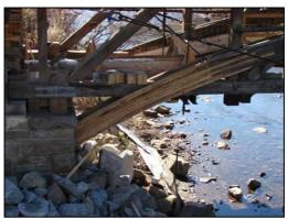
Fig 7: Laminated arch extended to reinforced abutment.
