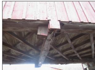
**2.6 Sheathing**: The trusses were clad with board and batten siding. The roof consisted of deteriorated asphalt shingles installed on top of deteriorated wood shingles on circular sawn nailers that had been mounted on sawn rafters fastened at the apex with trunnels. Wainscoting and a canted cap were in place to protect the lower area of the inside of the trusses from traffic debris.
