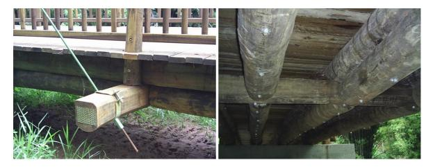
Fig. 9 Connections are stayed the transversinas stringers and double pieces.
