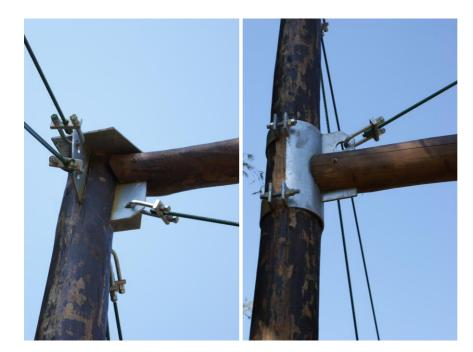
Fig. 8 Connects the poles of the footbridge.
