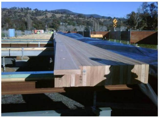
Figure 12 – Construction of the SLT deck showing laminate lay-up
