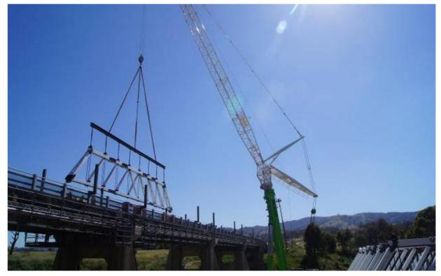
*Figure 10 – Truss being lifted into place using a 400t mobile crane*
