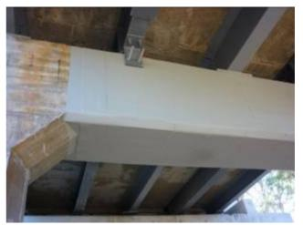
Figure 5 – FRP strengthening of the headstocks
