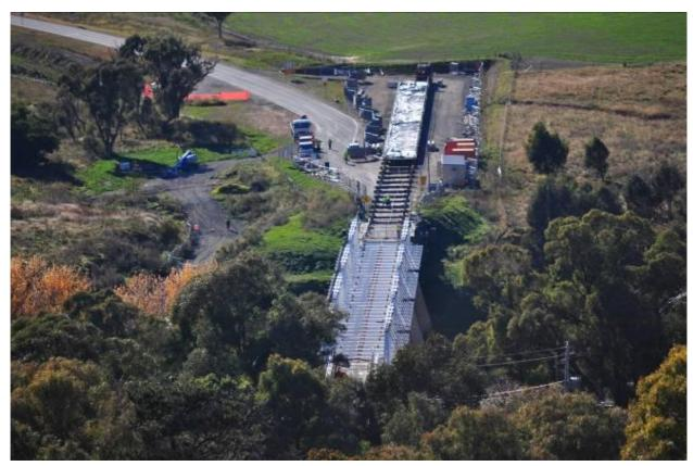
*Figure 14 – Launching of the SLT deck*
