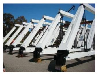
Figure 8 – Truss Assembly on site
