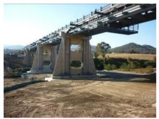
Figure 4 – Strengthening of the approach spans
