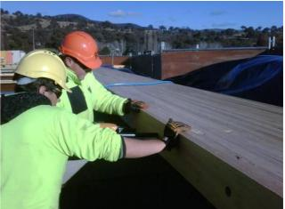
Figure 9 – Assembling the SLT deck on site
