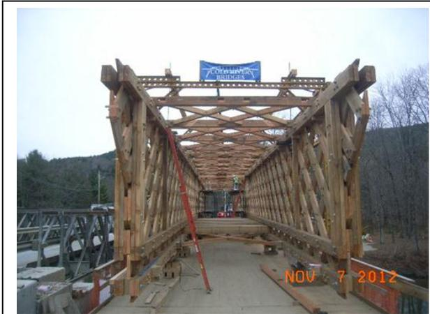
*Figure 3 - Replacement timber bridge being built on a work platform bridge. The temporary vehicular bridge is at left in this photo. They were racing to beat bad weather, but looking good.*
