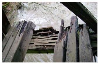
Fig.5 Bridge deterioration
