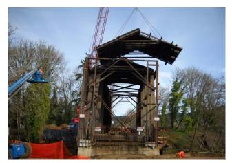
Fig. 6 Bridge being dismantled
