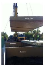
Fiberglass composite abutments, Panel One & Two
