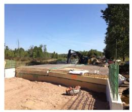
Fiberglass Composite Rigid Span installed
