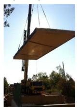
Panel One Fiberglass Composite Bridge Slab
