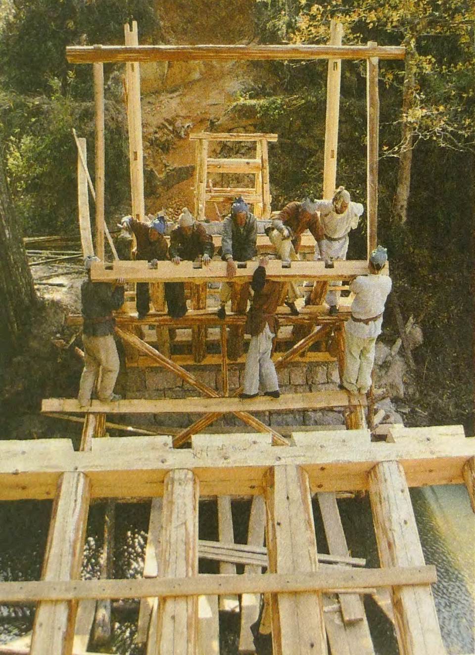
Construction of San Jie Miao, horizontal Miao (the 3 segment frame of the structure)
