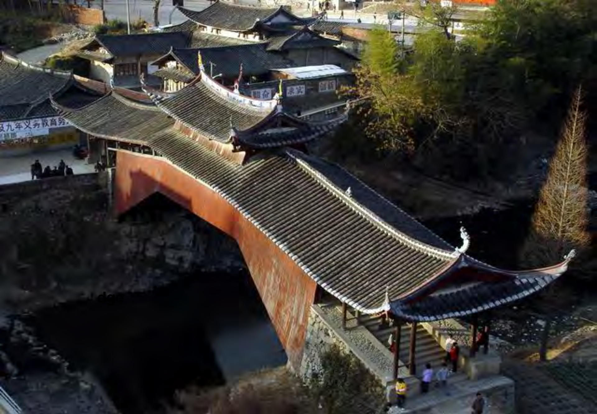
Xidong Bridge Taishun County, Zhejiang province Built in 1746 Length: 41.7 m Width: 4.9 m Net span: 25.7 m
