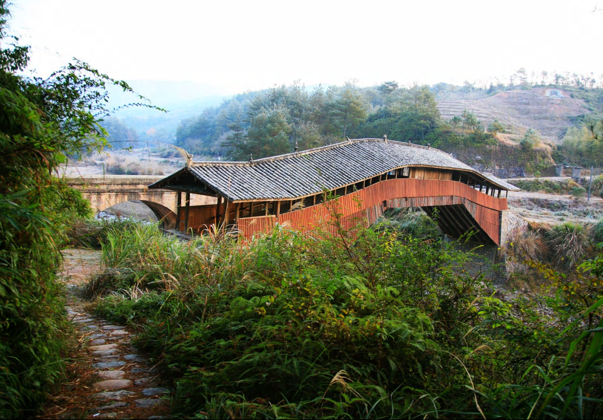
Xianju Bridge Taishun County, Zhejiang Province Rebuilt in 1673 Length: 41.83m Width: 4.89m Net span: 34.14m
