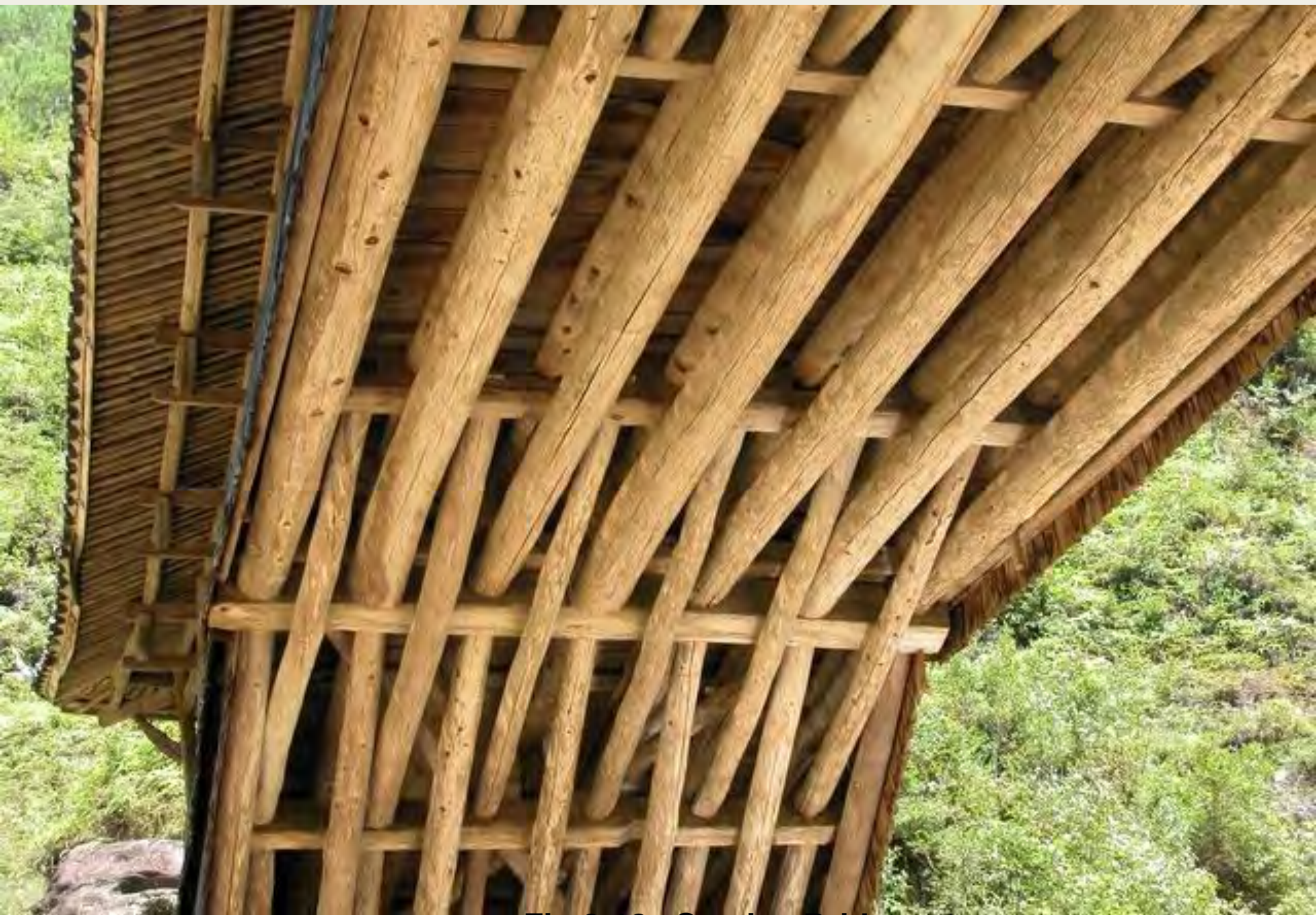
The Woven Timber Arch-Beam Structure of Santiao Bridge
