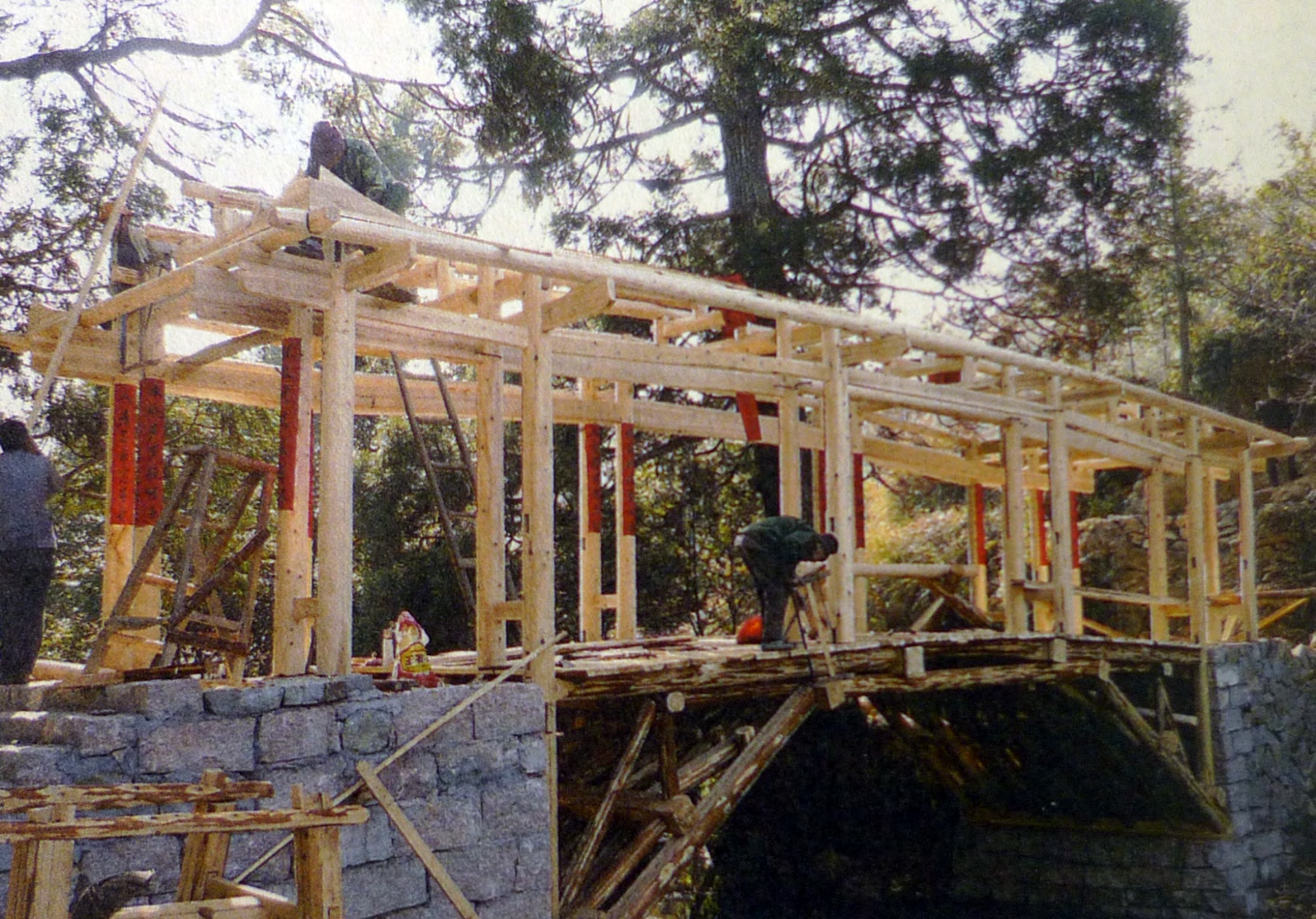
Erecting bridge house
