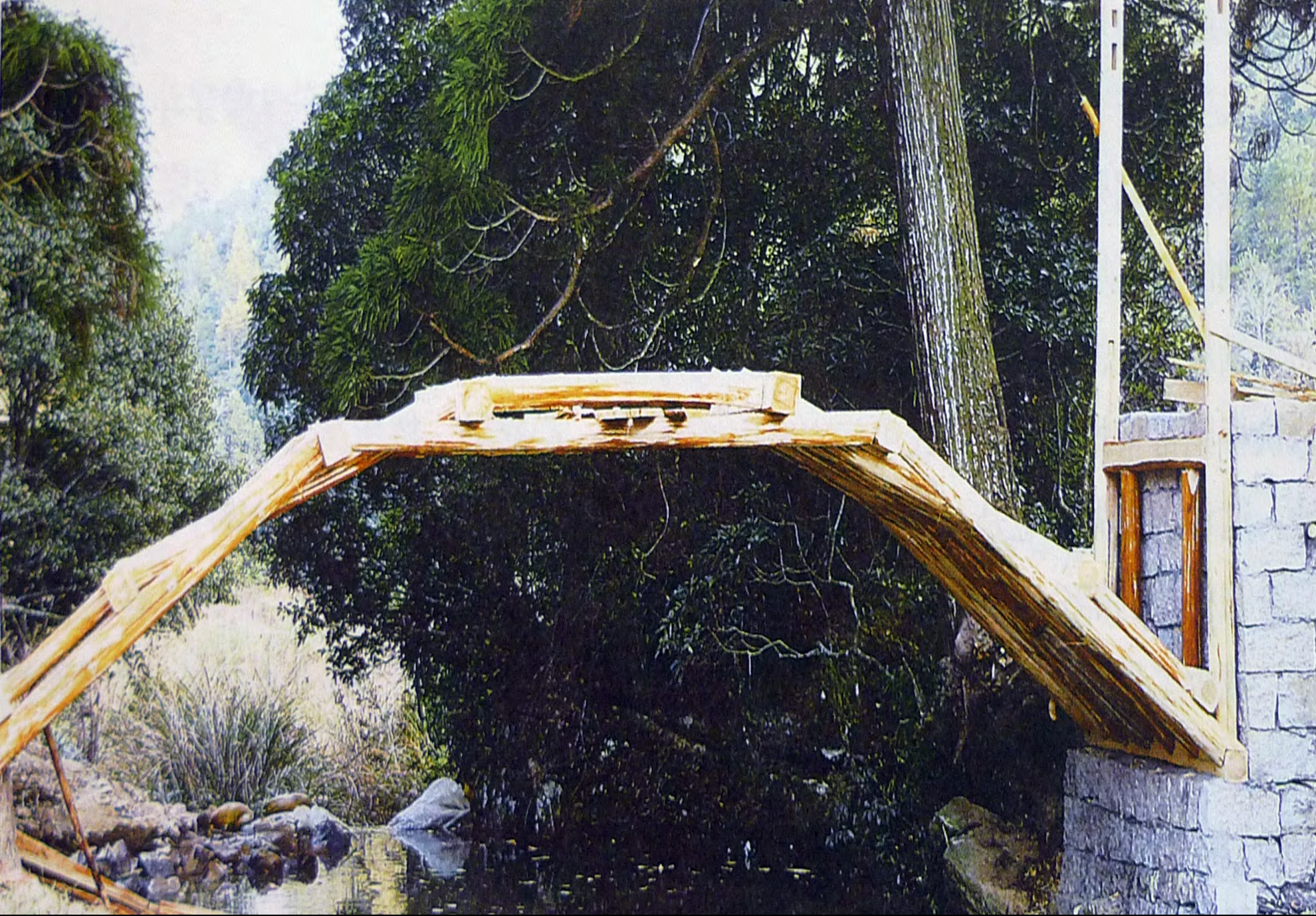
Finishing timber arch frame woven structure
