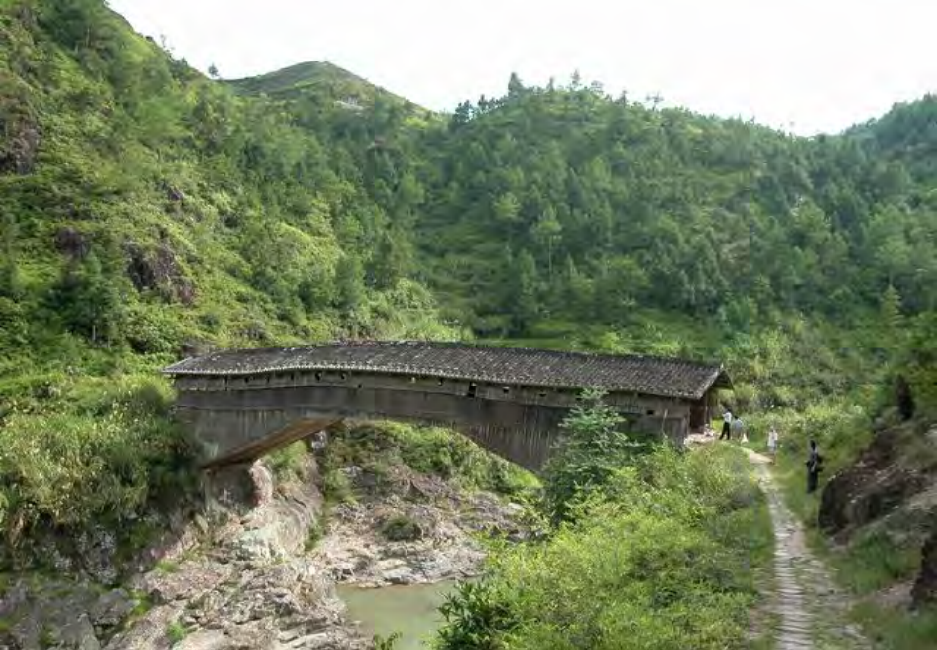
Zhangkeng Bridge, Shouning County, Fujian Province Built in 1828 Length: 40m Width: 5m Net span: 33.4 m
