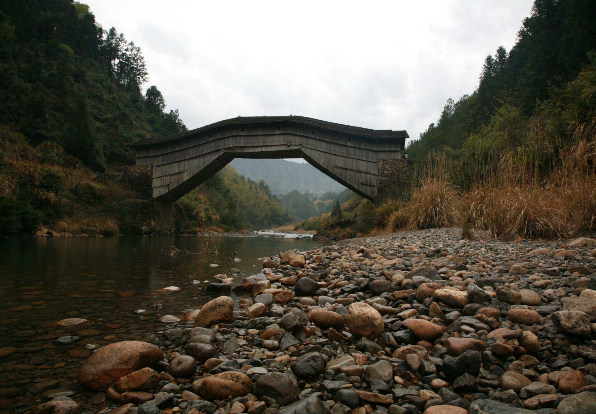
Red Army Bridge Taishun County, Zhejiang Province Rebuilt in 1954 Length: 39m Width: 5m Net span: 32.9m
