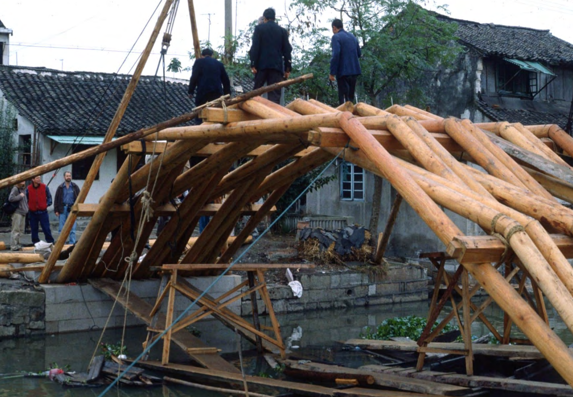
The lifting equipment used by NOVA during the construction of Rainbow Bridge is manual hoisting.
