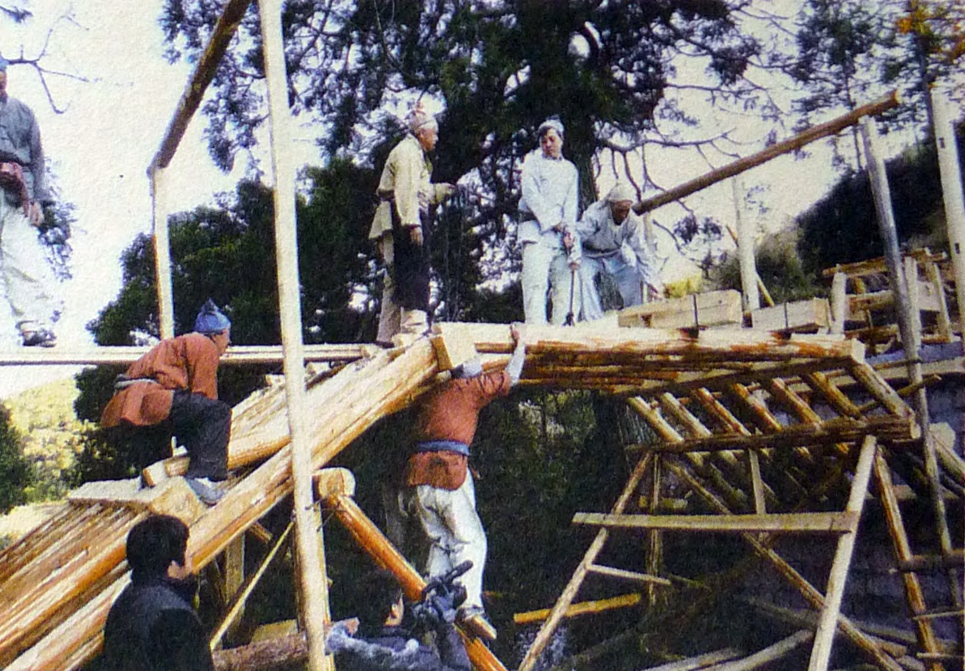
Setting up Wu Jie Miao, acclivitous Miao (the 5 segment frame of the structure)
