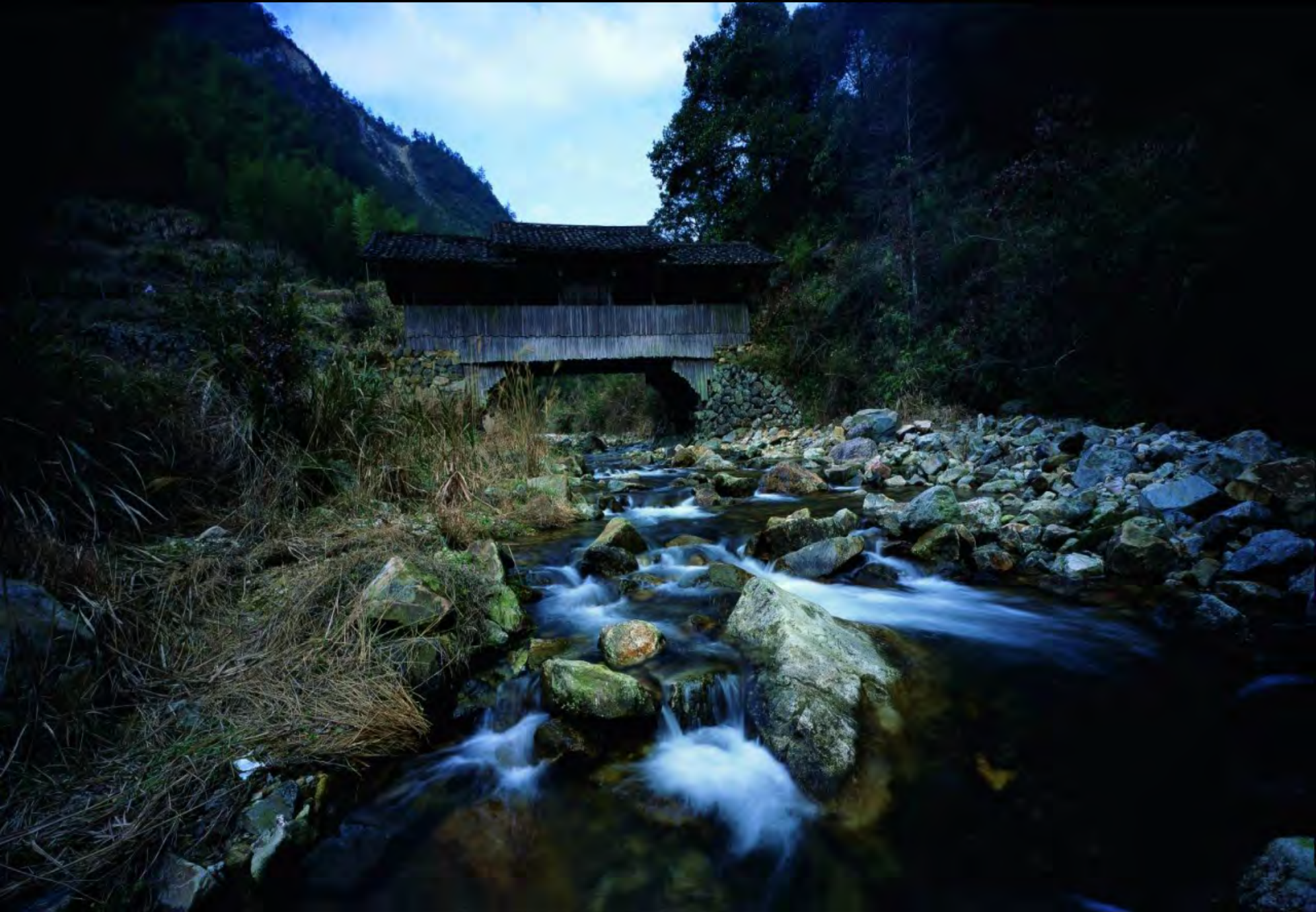
Chengshui Bridge, Taishun County, Zhejiang Province Built in 1942 Length: 15m Width: 4.6m Net span: 11.2m
