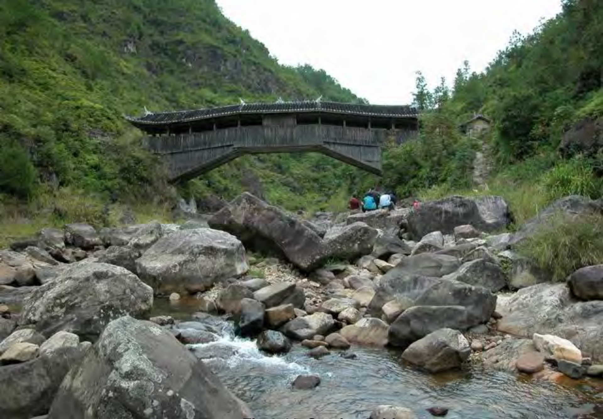
Santiao Bridge Taishun County, Zhejiang province Built in 1843 Length: 32 m Width: 3.96 m Net span: 21.26 m
