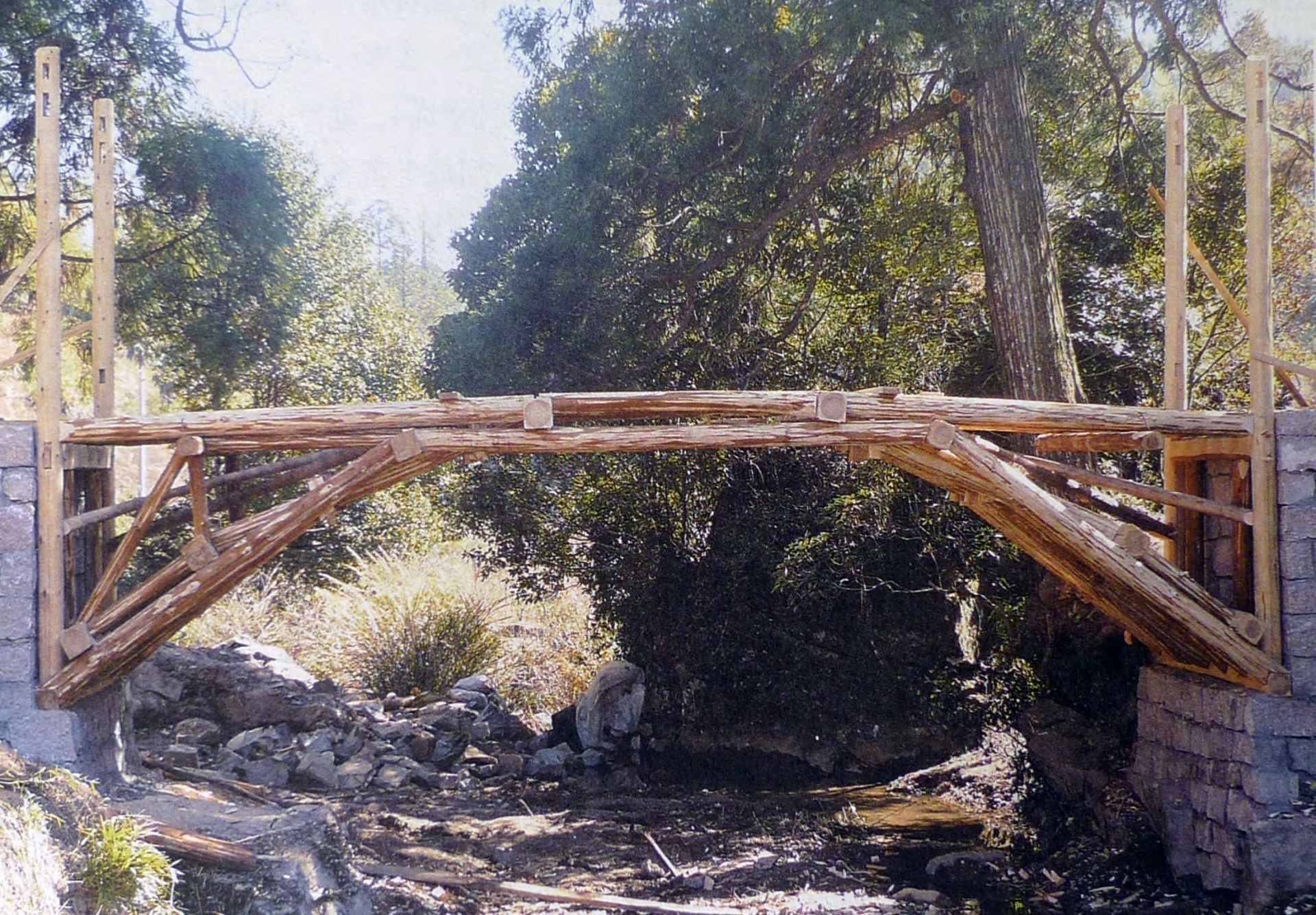
Arch frame system after construction completion
