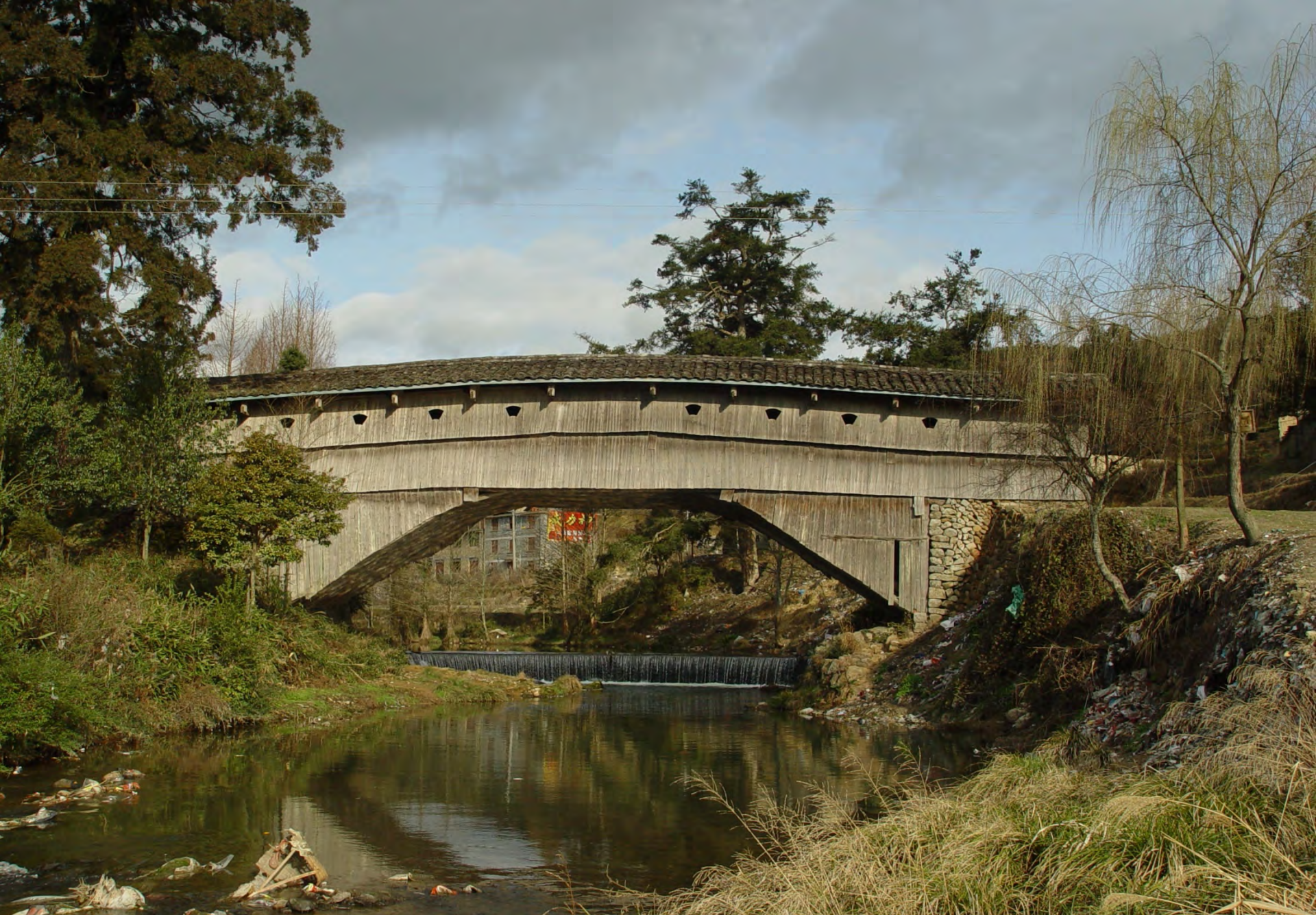
Guangli Bridge, Pingnan County, Fujian province Rebuilt in 1774 Length: 30.5m Width: 4.5m Net span: 20.6m
