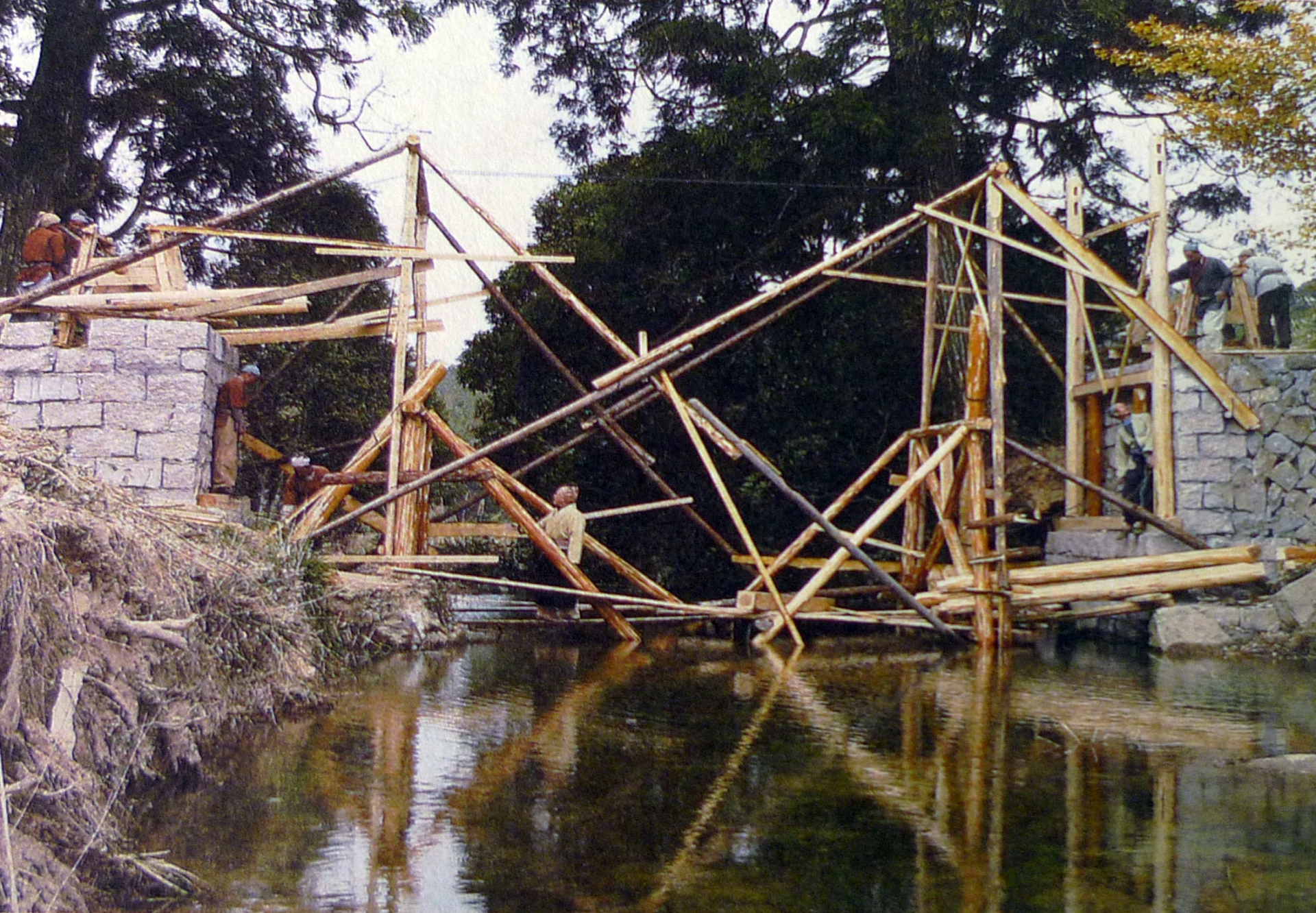
Building bridge abutment and erecting frame and columns in the water(a kind of manual hoisting)
