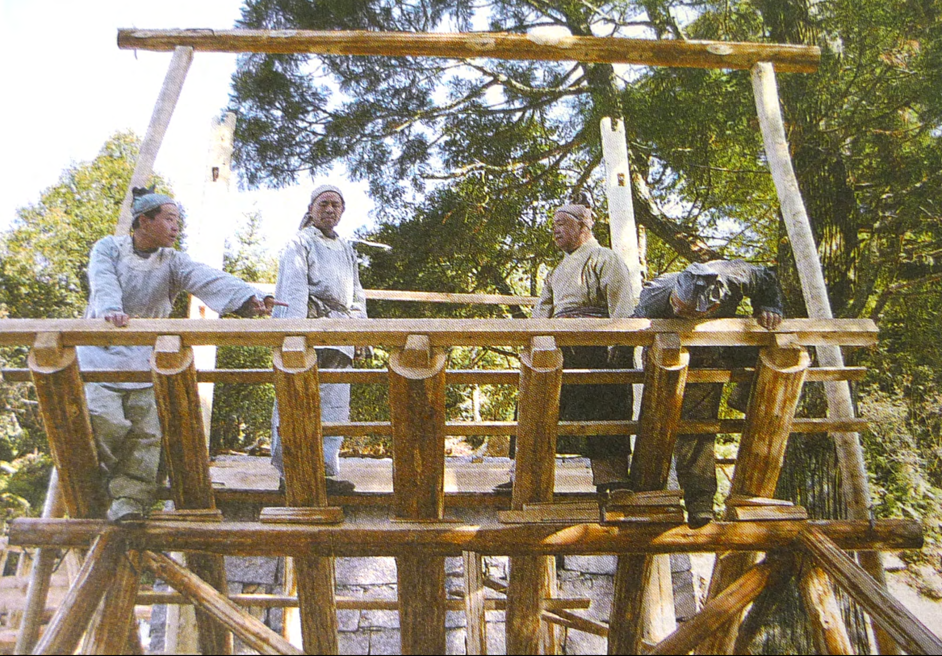
Construction of SanJieMiao (the 3 segment frame of the structure)
