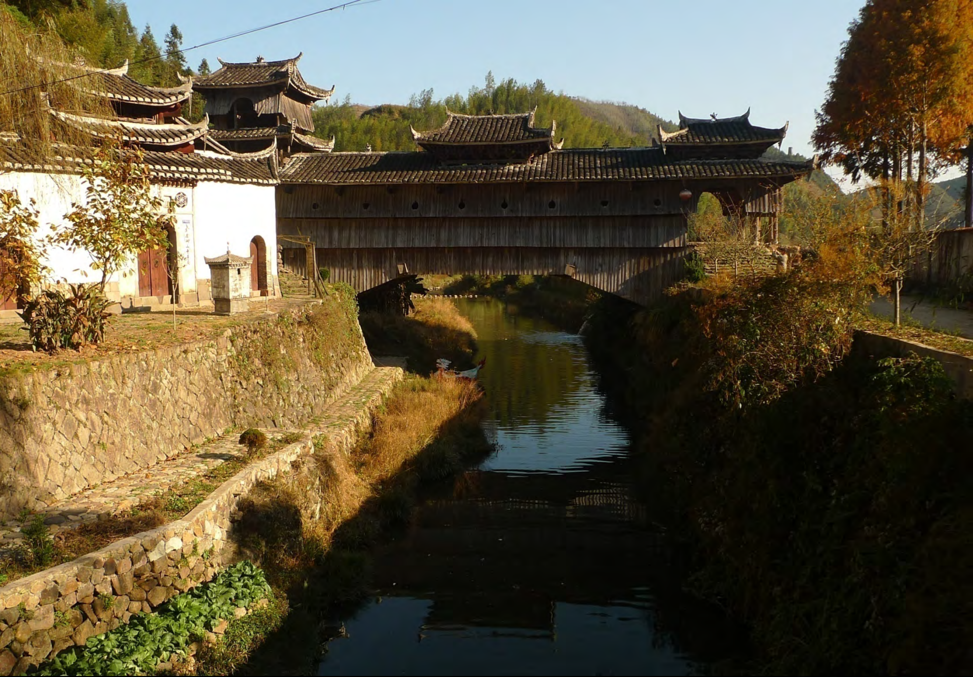
Rulong Bridge, Qingyuan County, Zhejiang province Built in 1625 Length: 28.2m Width: 5.1m Net span: 19.5m
