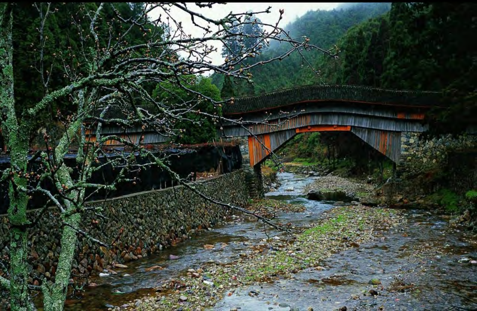
Huangshuichang Bridge Qingyuan County, Zhejiang Province Rebuilt in 1872 Length: 54.3m Width: 4.9m Net span: 17.45m
