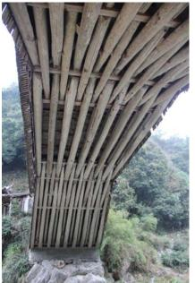
While the woven arch is almost equal to the whole structure of the Rainbow Bridge, it serves only partial for that of the mountain bridges. Beyond the two woven-together systems, the deck system works as the third arch system, shown in blue, and the diagonal elements and struts in between help to form a 3-dimensional spatial structure.
