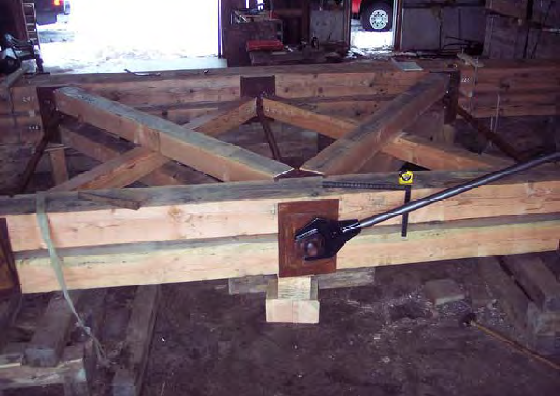
Final fit and assembly of mid-span braces and counters. Third time's a charm.
