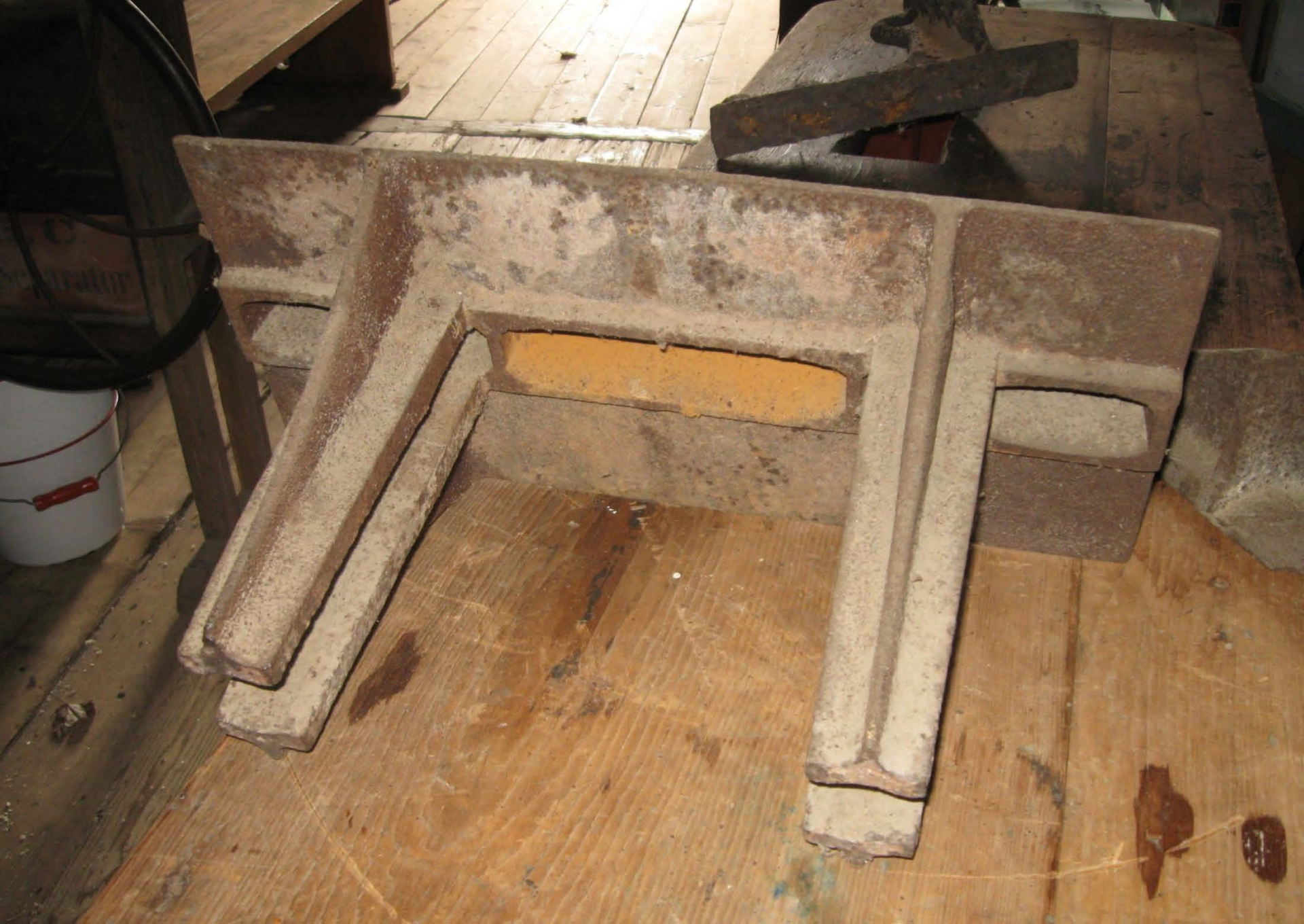
Nodal Castings from Rexleigh Covered Bridge, New York
