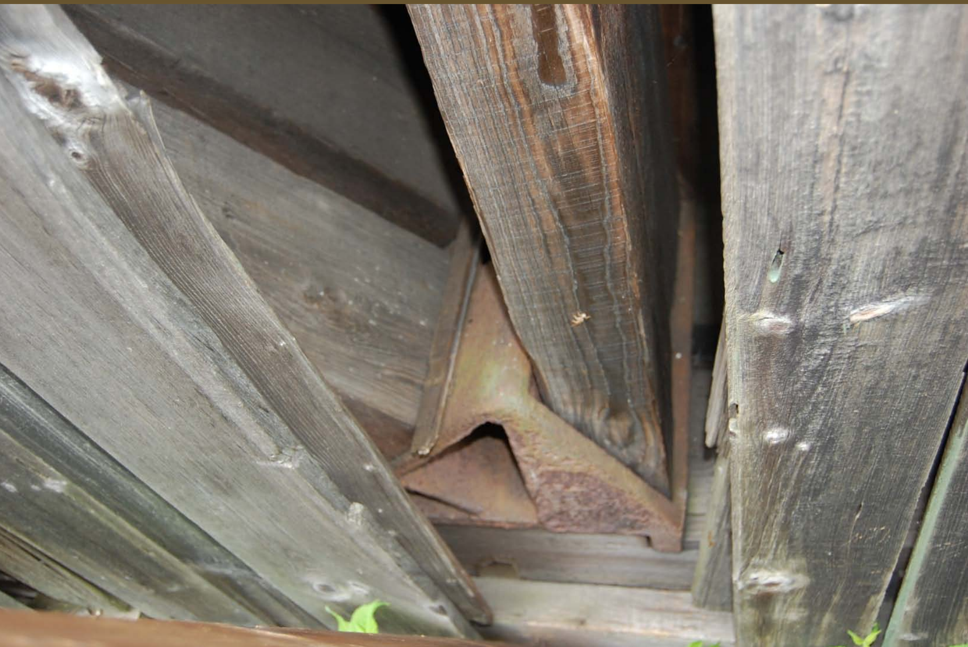
Revealed end post casting, Snyder Brook Bridge
