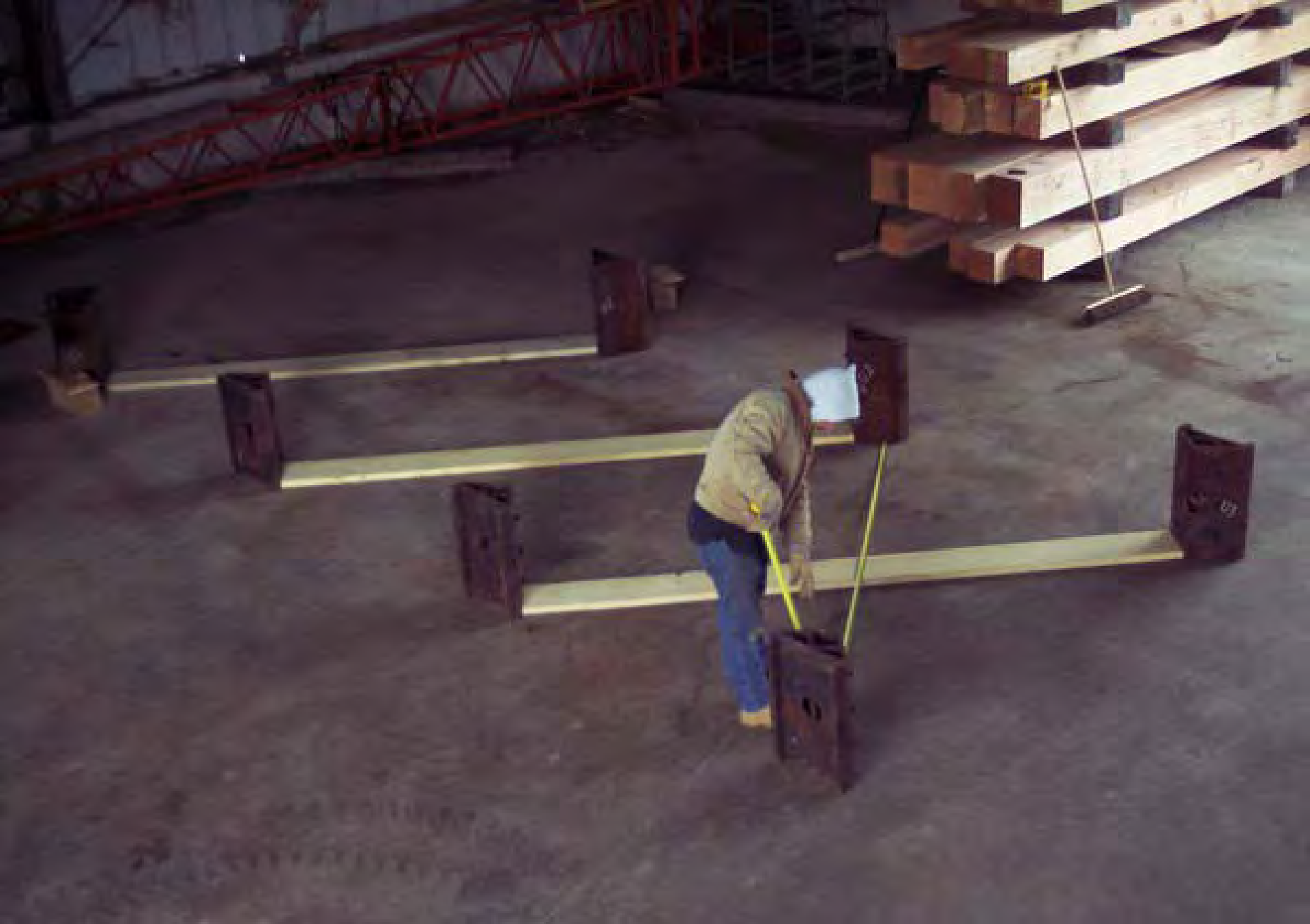
Lofting truss members based on forensic geometry
