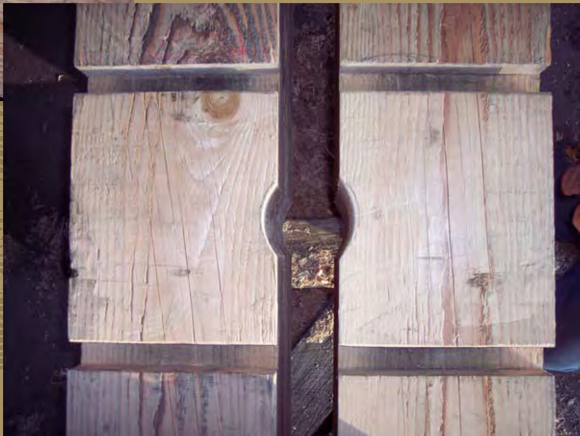
Hand-tooled housings for truss vertical rods and cast shoes
