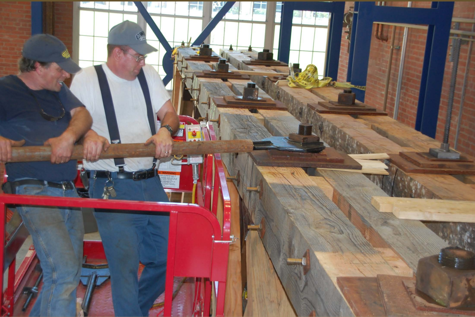
Tightening bolts on second truss, Mar 19, 2012
