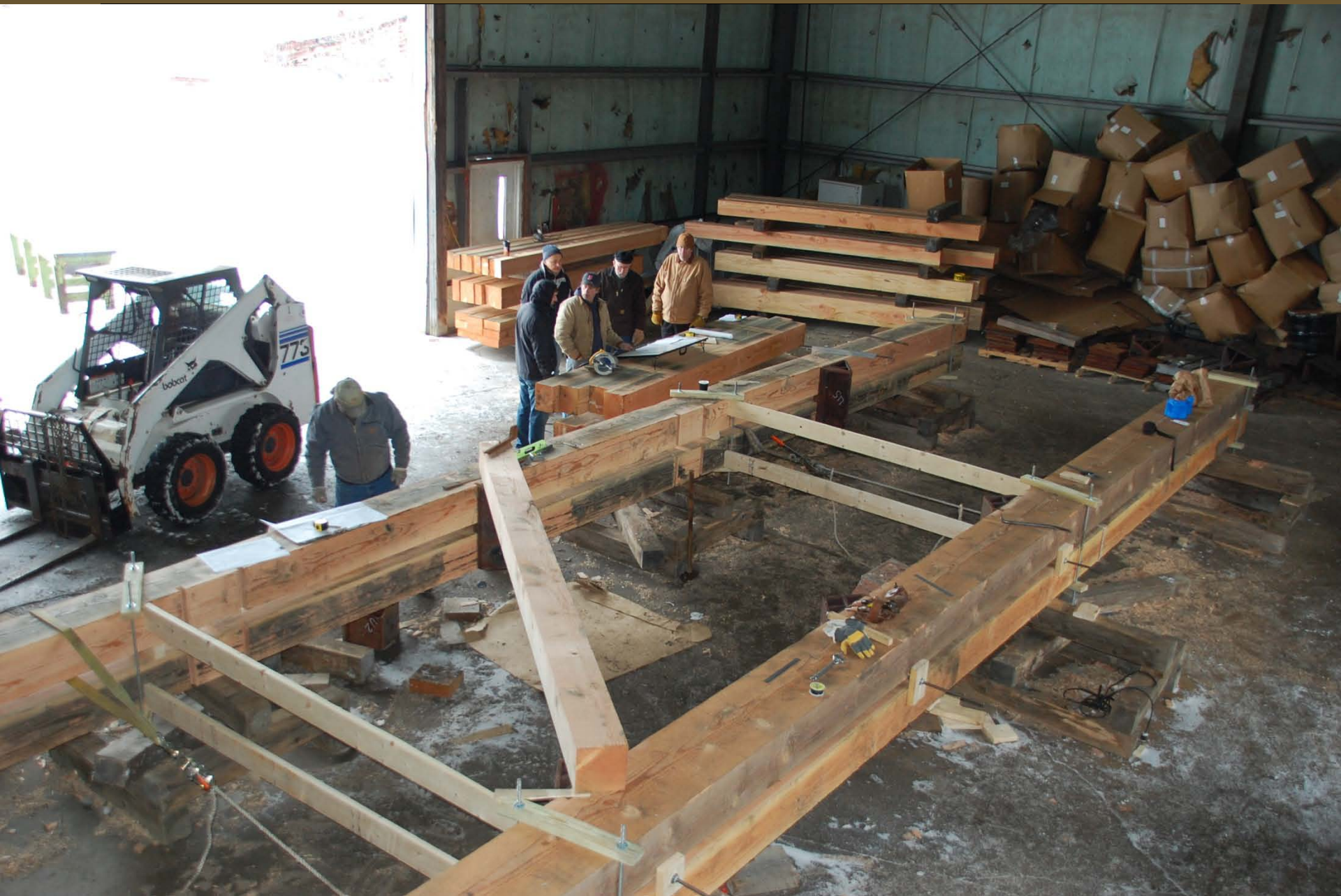
Lofting and plumb scribe layout of first diagonals, March 10, 2011
