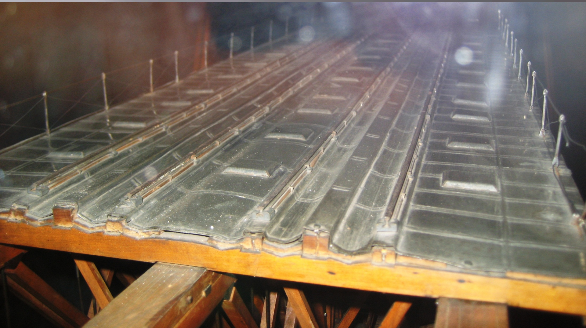
Weather protection of top deck, Verebja Bridge
