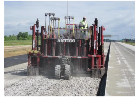
Rubblizing - Photo courtesy of Antigo Construction
