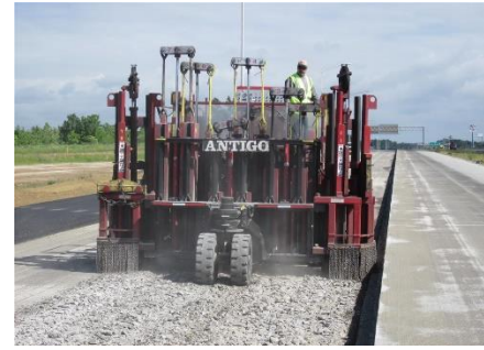
Rubblizing - Photo courtesy of Antigo Construction
