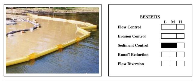
**Description:** A flotation silt curtain (also called a turbidity curtain) consists of a geosynthetic fabric that is suspended vertically in a body of water. The top of the curtain is attached to floats, and the bottom is weighted.
