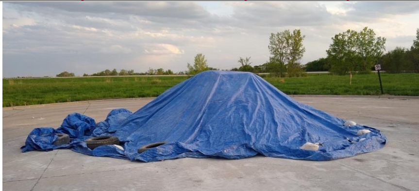
Figure 7E-XX.01: Small Material Stockpile with Protective Tarp Cover
