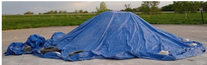
Figure 7E-30.01: Small Material Stockpile with Protective Tarp Cover
