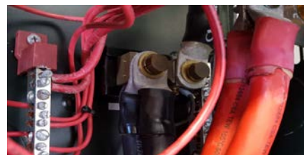
Existing Battery Shunt 500A @ 50mV
