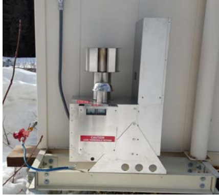
External Mounted TEG on custom platform
