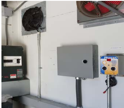
Installation of RMS-300 in control box and conduit
