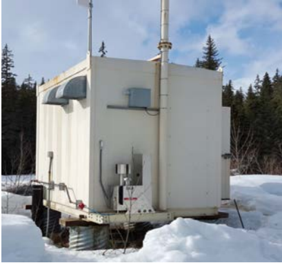
External Mounted TEG and propane line/regulator
