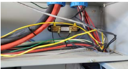
TEG Current Shunt 10A @ 50mV
