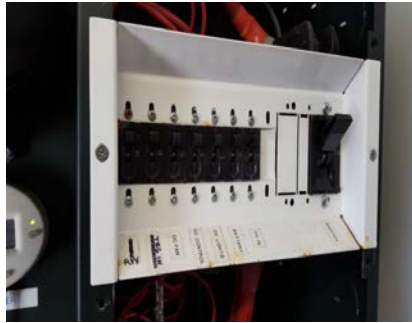
Existing DC breaker panel with labeled TEG breaker
