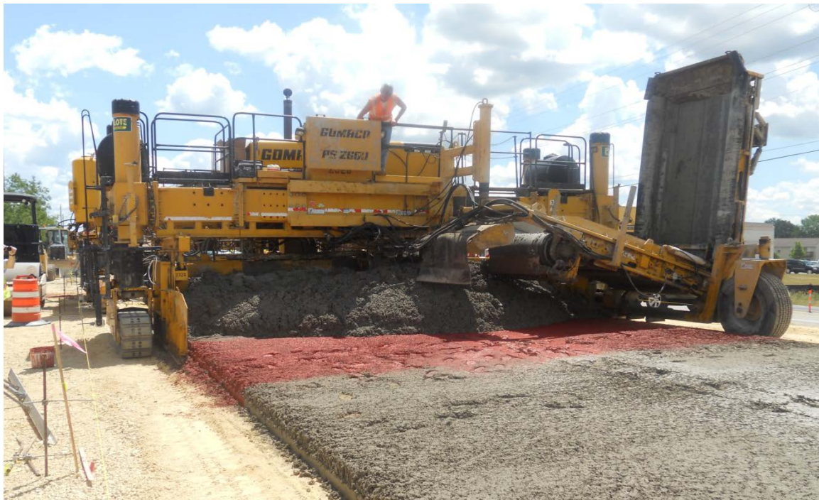
Figure 3. Top Lift Being Placed on the Unconsolidated Lower Lift
