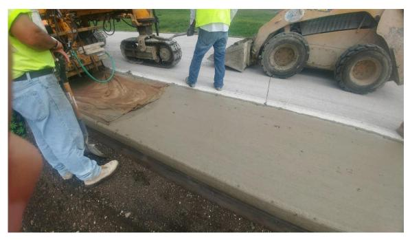
Figure 6: Paving with PEM Shoulder Mix
