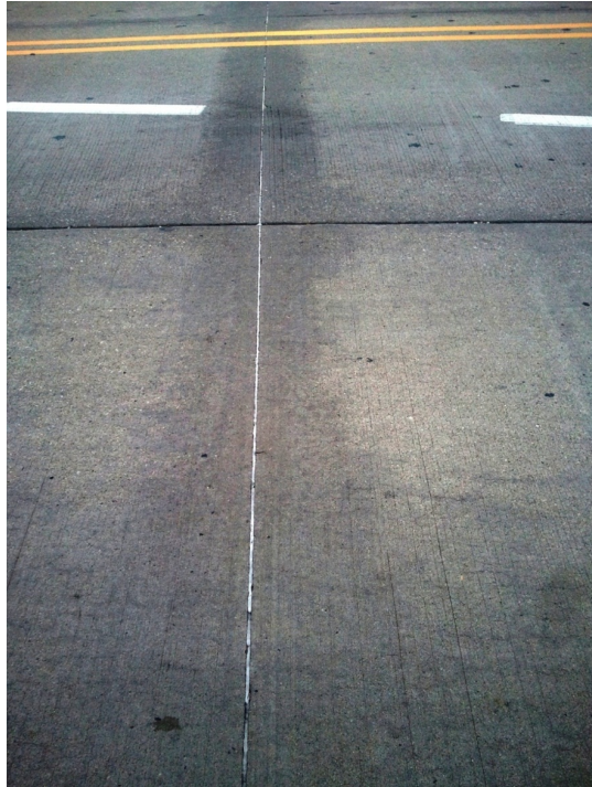
Shadowing - Potential sign of saturation
