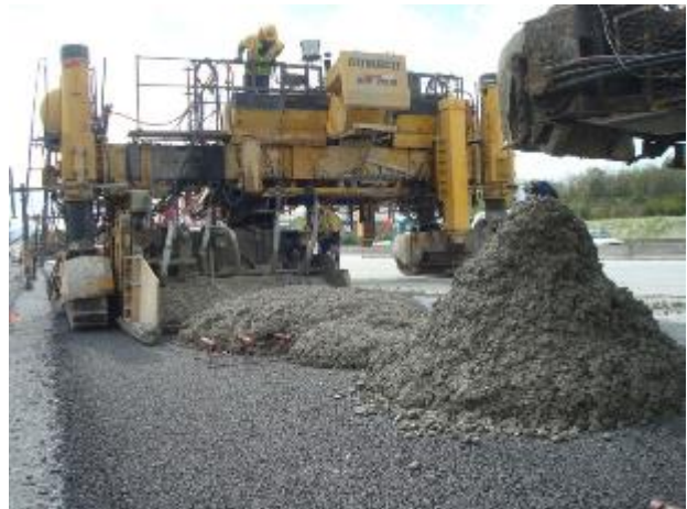
d. Mix placement and paver.
