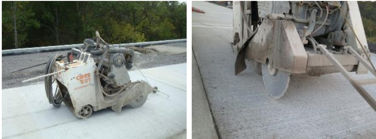
Figure 11. Photo. Transverse joint and saw.
