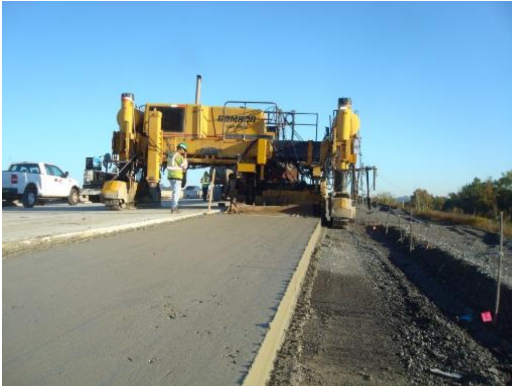
Photo E-41. Day 2 bottom lift placement, viewed from behind paver.
