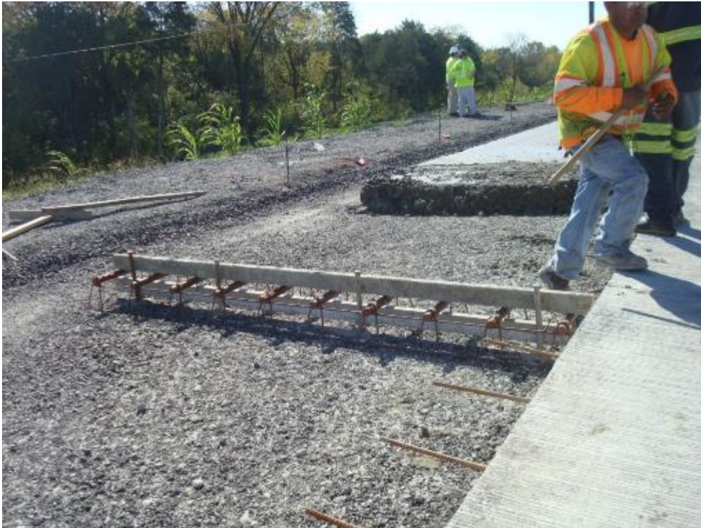
Photo E-43. Construction of Day 2 header.
