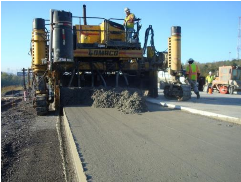
Photo E-42. Day 2 top lift placement, viewed from in front of paver.
