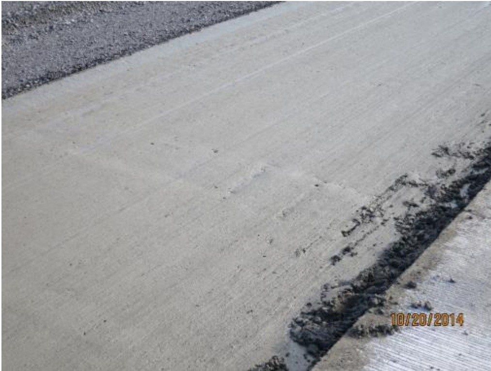
Photo E-23. Dowel “shadowing” and surface depressions and debris near end of Day 1 placement of bottom lift.
