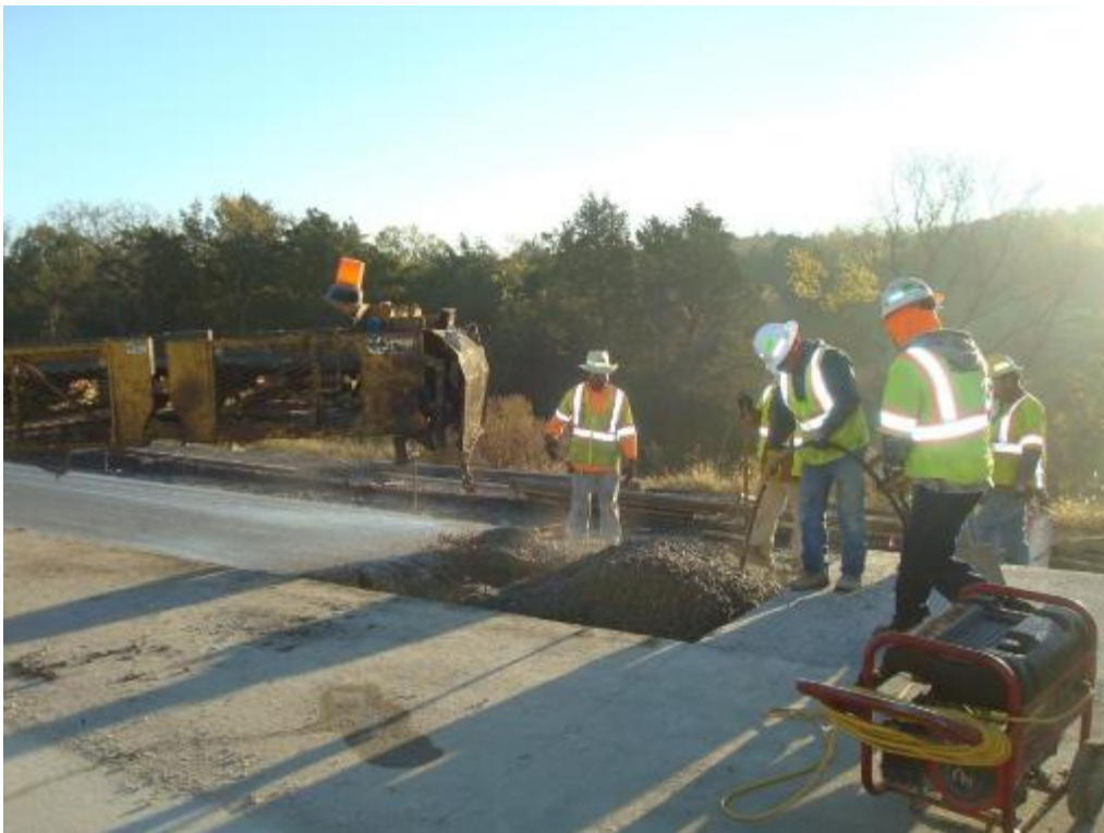
Photo E-40. Hand placement to close gap with header at start of Day 2 paving.
