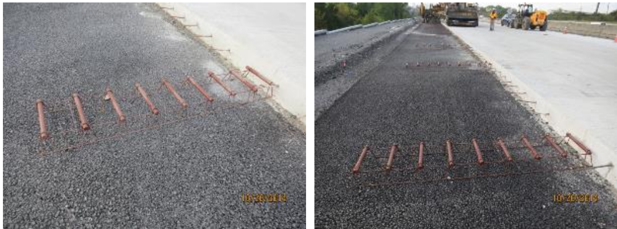
Figure 6. Photo. Dowel bar and tie bar configuration.
