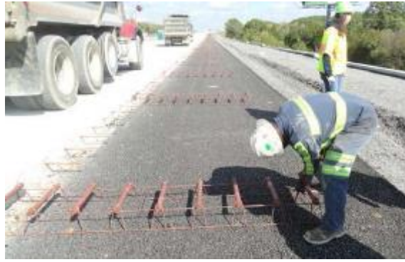
Figure 45: Shipping Wires being Cut
