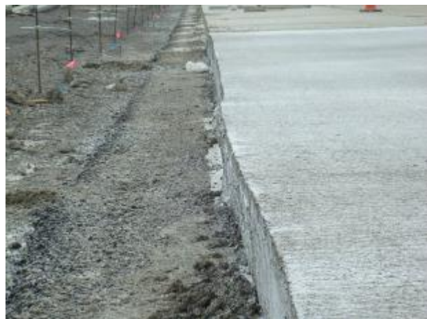
d. Wandering edge in high slump area.
