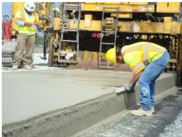
c. Workers effort to repair edge slump.
