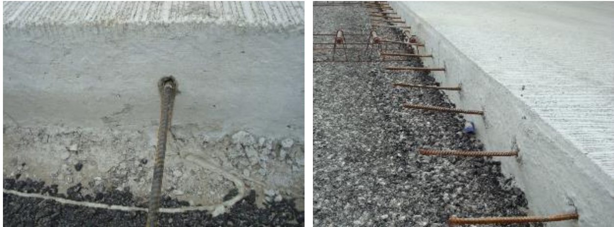
Figure 5. Photo. Tie bar placement.
