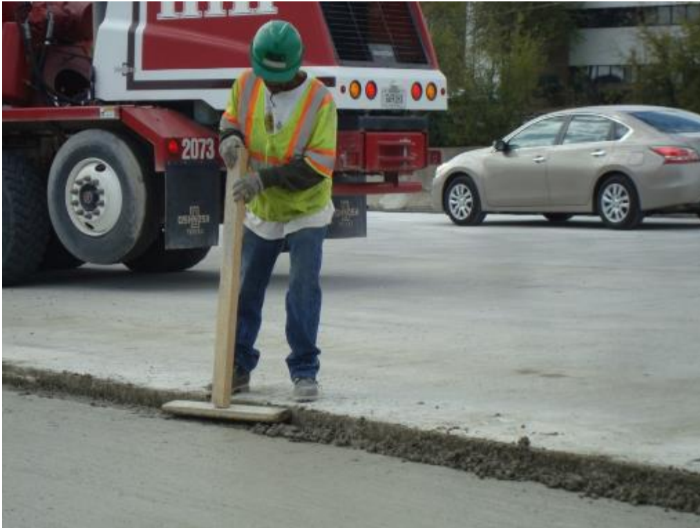
Photo E-21. Worker tamping down excess concrete at lane/shoulder joint after placement of bottom lift.
