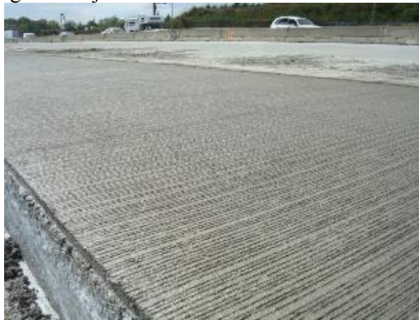
c. Completed transverse tining
