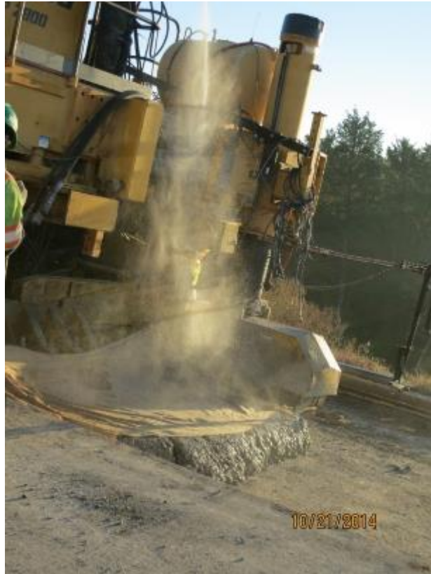
Photo E-39. Water being sprayed on burlap drag at start of Day 2 placement.
