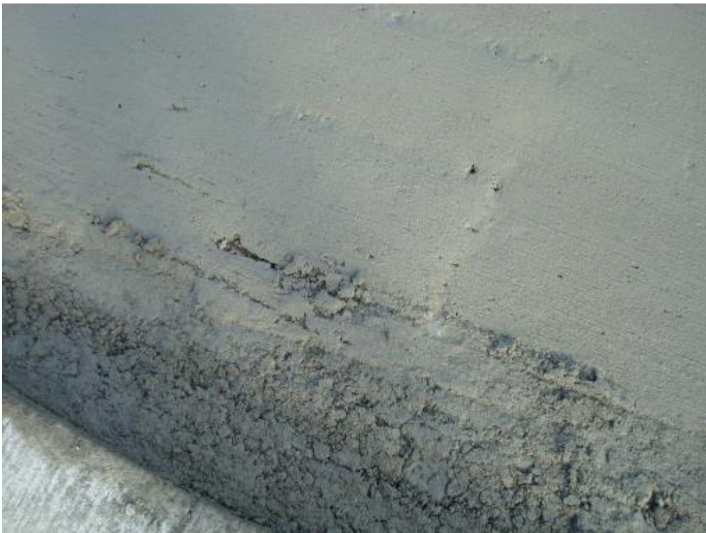
Photo E-24. Exposed dowel end in bottom lift due to thin lift.
