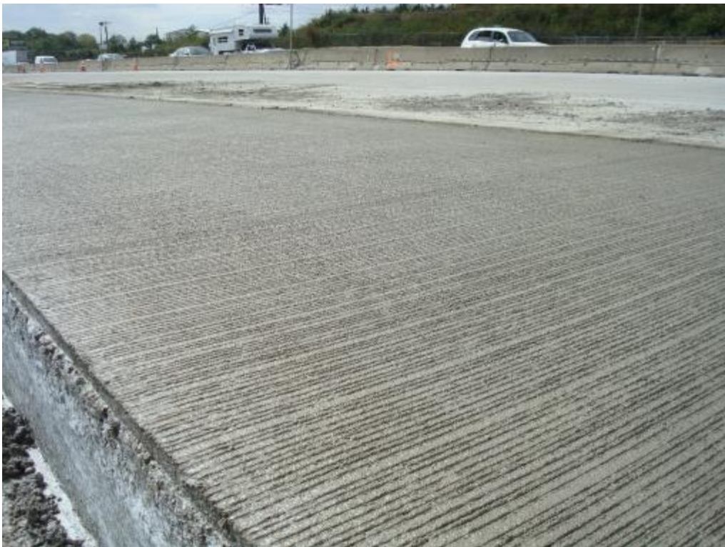
Photo E-50. Tined pavement surface.
