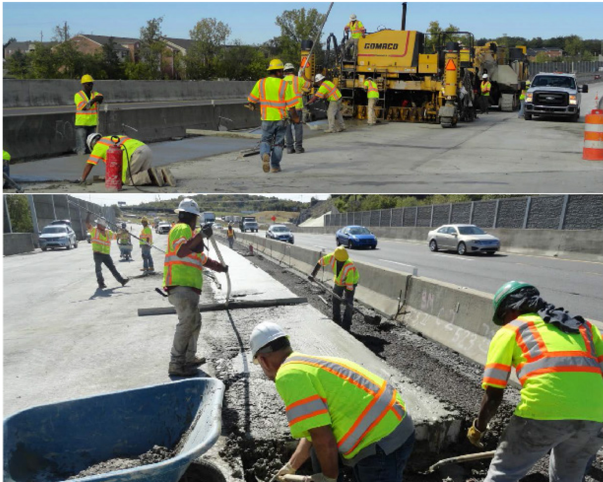
Figure 16: Construction of the shoulder using the conventional mixture
