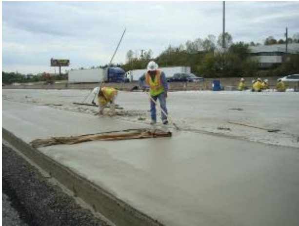
a. Maintaining longitudinal joint.
