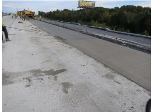
b. Concrete tining.
