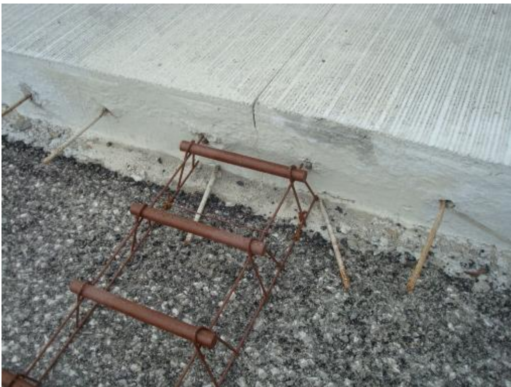
Photo E-4. Dowel basket placement showing proximity to travel lane and interfering with tie bars.
