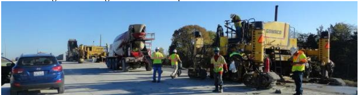
Figure 19: Paving Train for the Composite Lift Pavement Construction
