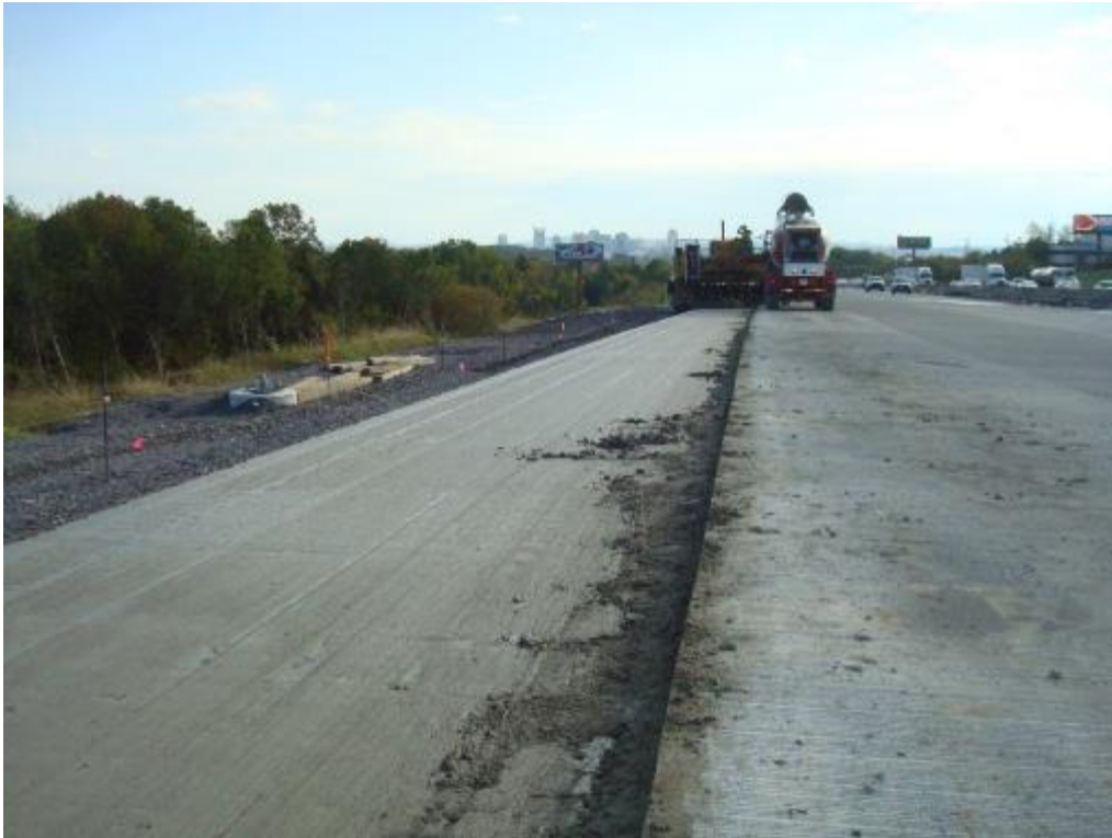
Photo E-25. Dowel “shadowing” in bottom lift surface and surface condition ahead of top lift placement at end of Day 1.
