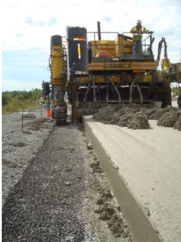
Photo E-27. View of top lift paving from in front of paver.
