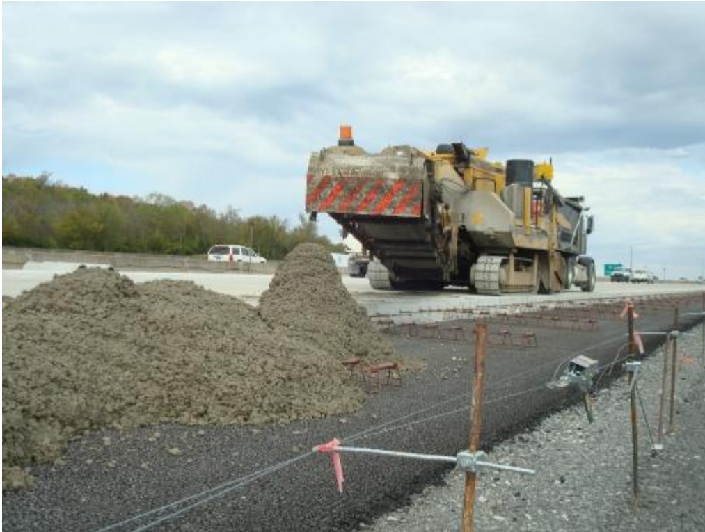
Photo E-13. Bottom lift concrete deposited on base by belt placer ahead of paver.
