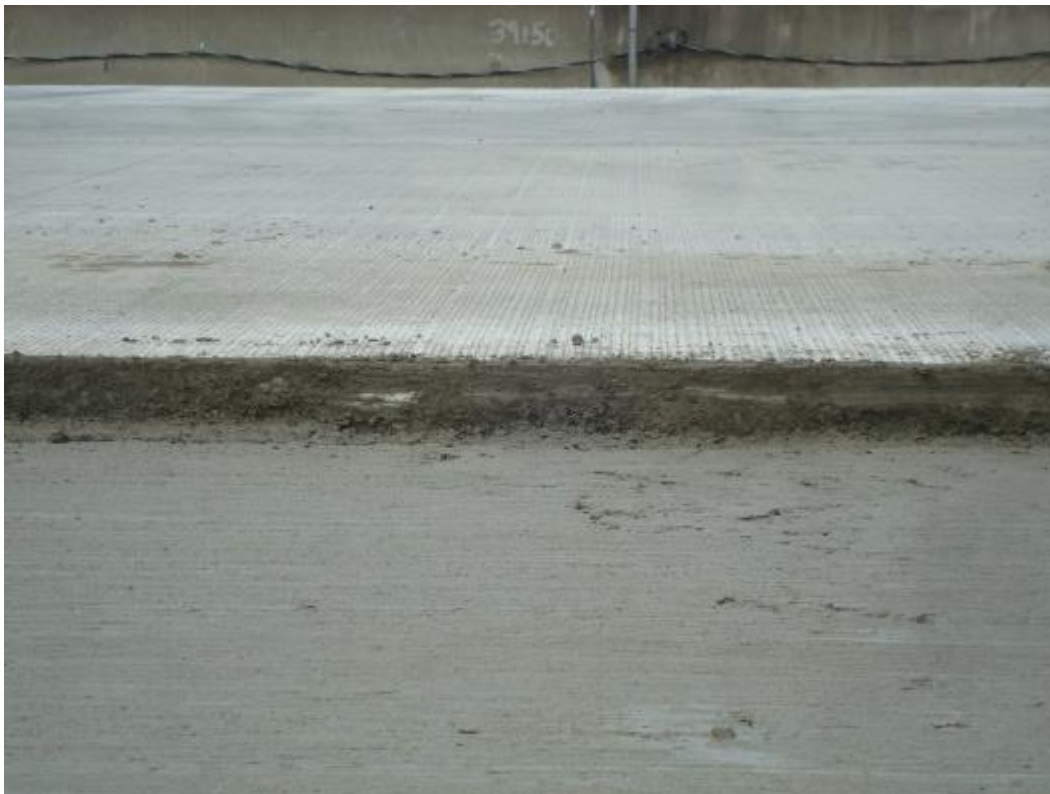
Photo E-20. Bottom lift surface behind paver (note: top lift will need to be more than 3 inches thick in this area).
