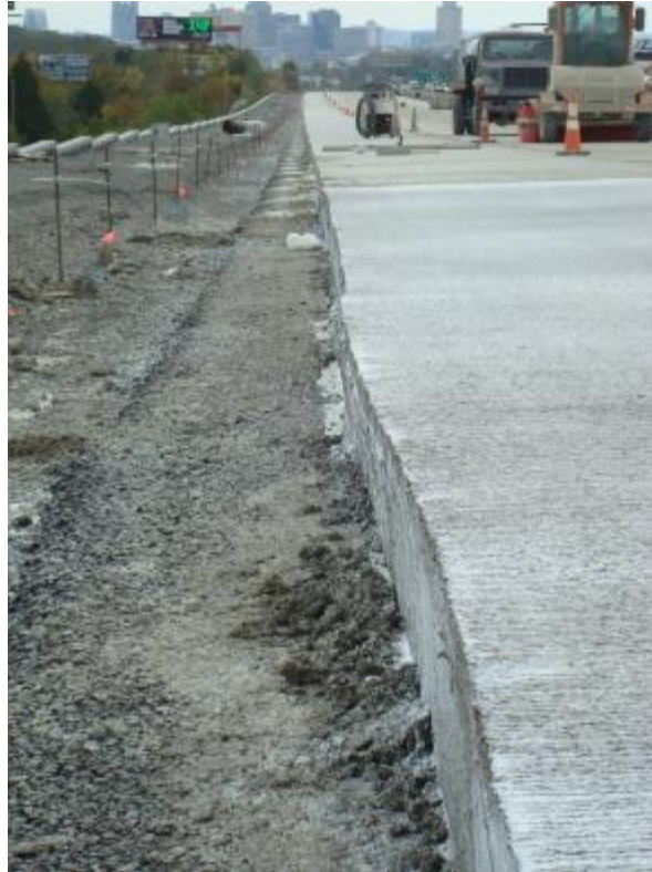
Photo E-33. Edge blowout #2 after repair.
