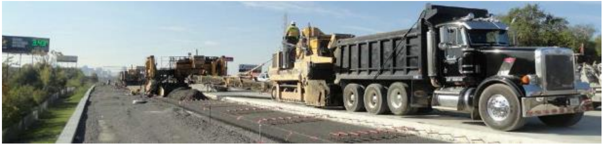
Figure 18: Paving Train for the Composite Lift Pavement Construction
