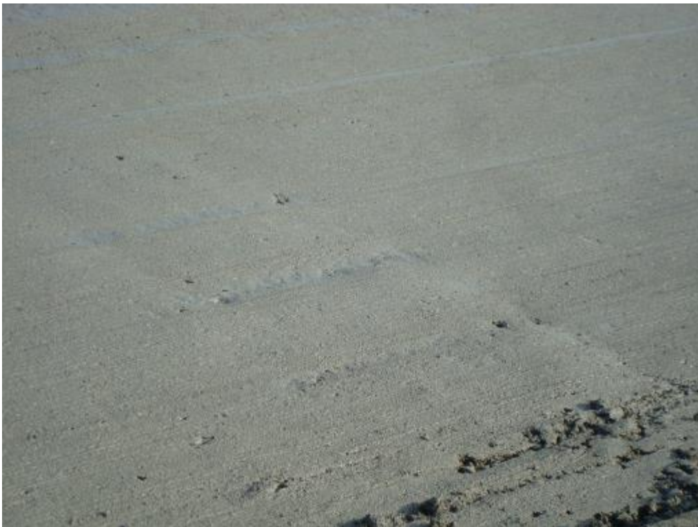
Photo E-22. Bottom lift surface "shadowing" due to proximity of dowels (thin lift).
