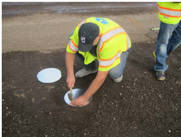
a. Placement of metal discs.
