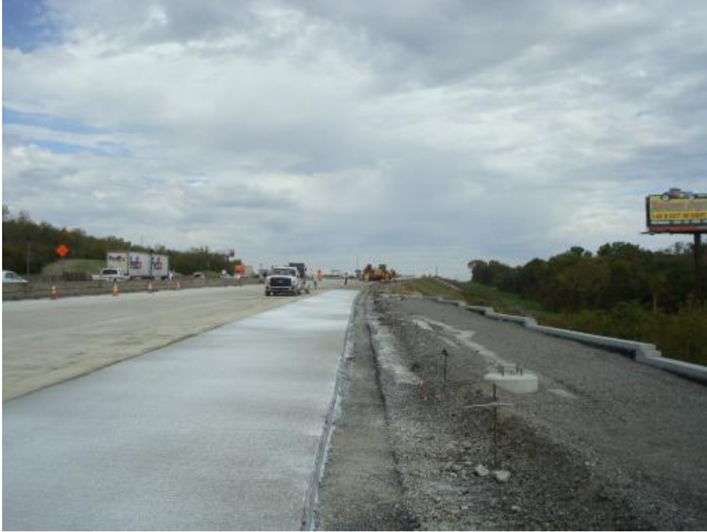
Photo E-53. Shoulder appearance after typical cure application.
