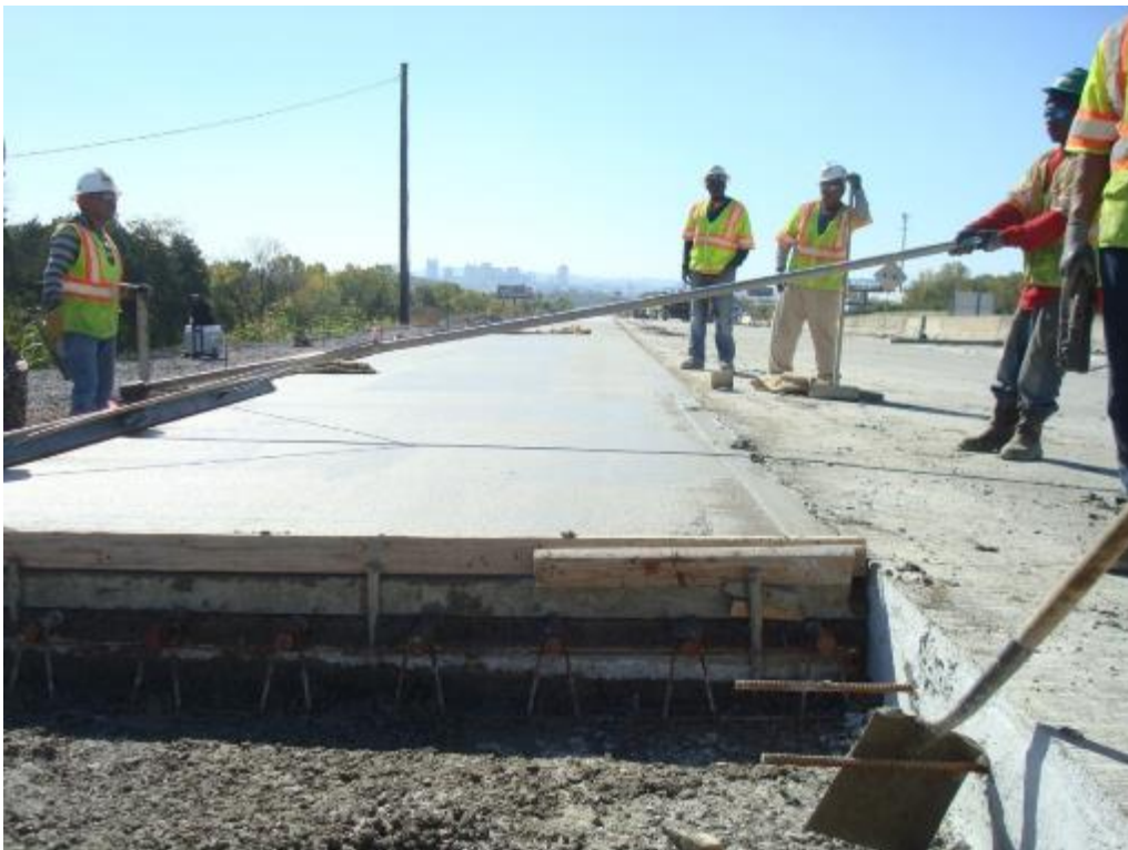
Photo E-44. Finishing pavement at Day 2 header.
