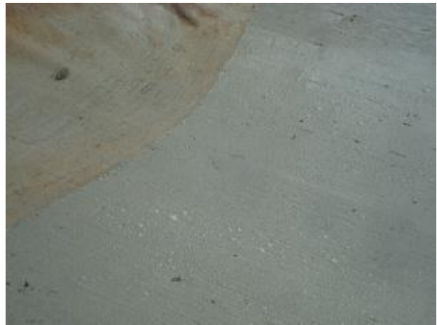
b. Surface water bubbles.
