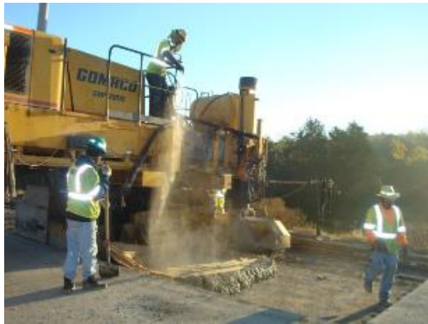
a. Watering burlap on bottom lift.
