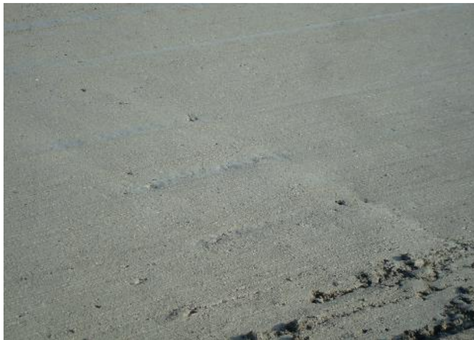
Figure 14. Photo. Thin bottom lift with dowel bar “shadowing.”
