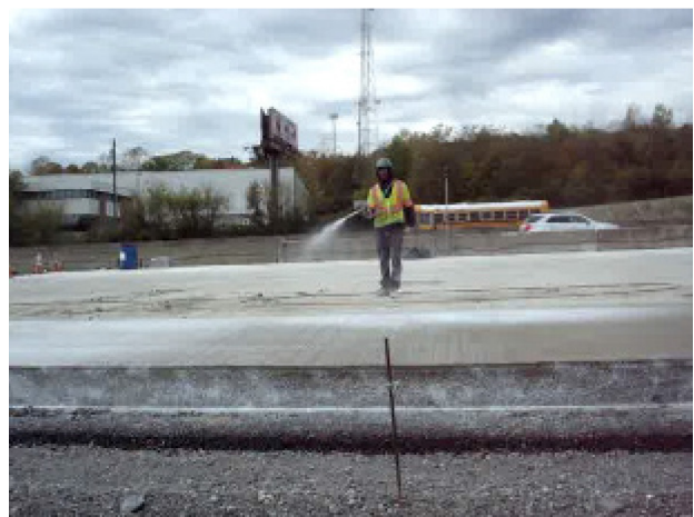
b. "Hand" spraying curing compound.
