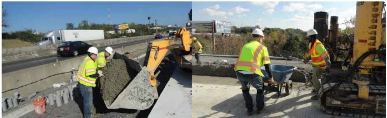
Figure 20: Sampling on the Grade
