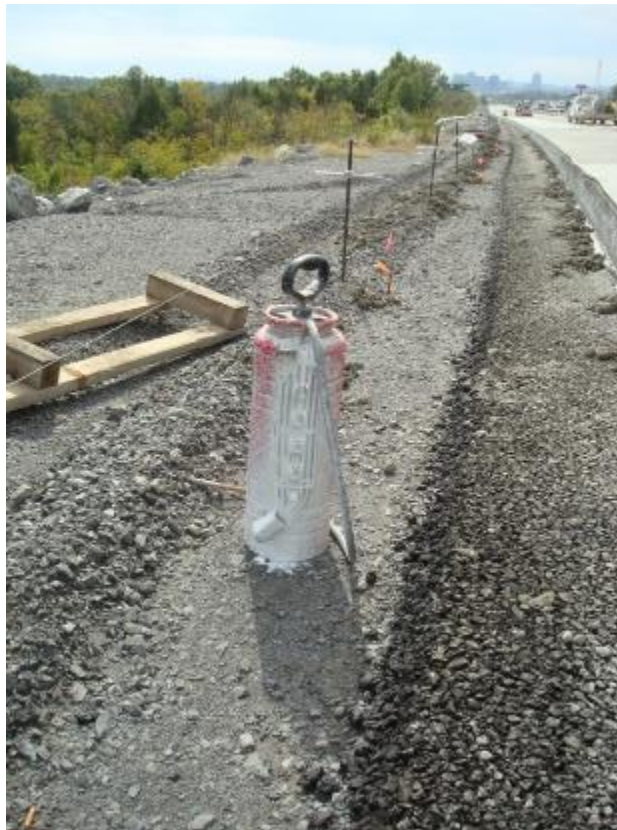
Photo E-54. "Garden sprayer" used for applying cure compound to outside shoulder edge.
