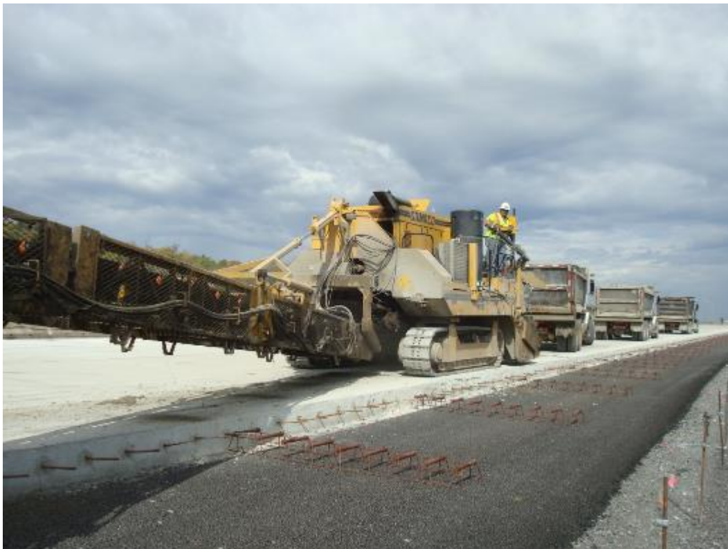
Photo E-12. Dump trucks and belt placer used for transport and placement of bottom lift concrete.
