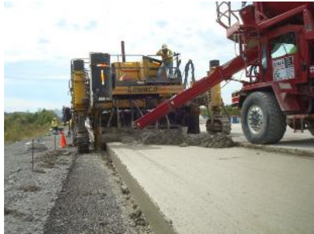
b. Mix delivery and paver.
