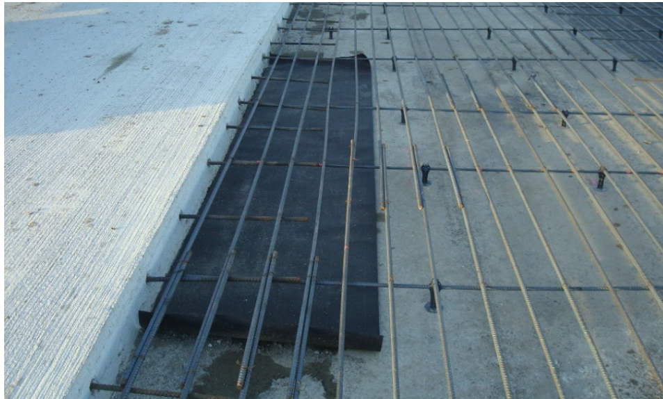
Figure 17. “Tar paper” covering paver track damage to asphalt interlayer.
