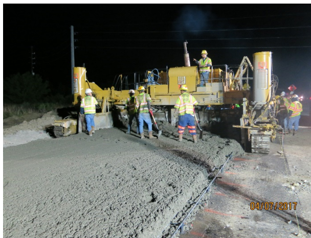
b. Bottom-lift paving.
