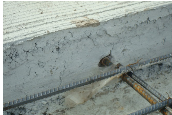
b. Consolidation issues and shrinkage cracking at longitudinal construction joint.
