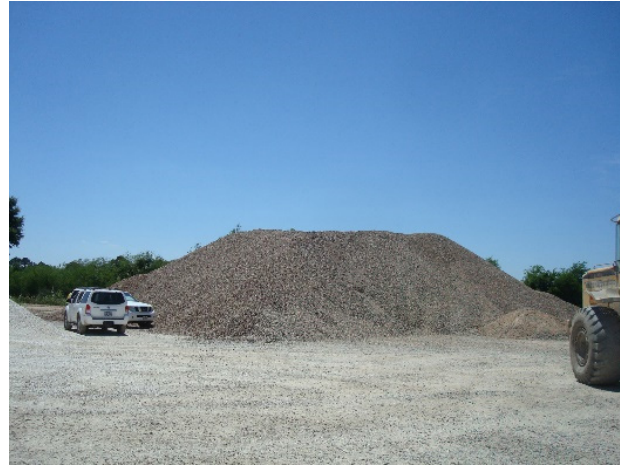
b. Coarse aggregate stockpile.
