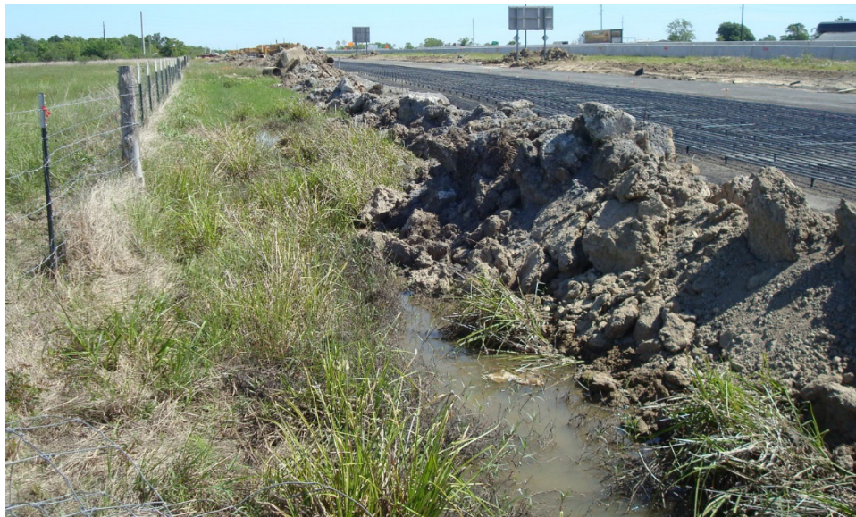
Figure 3. Typical wet ditch conditions along north side of project roadway near west end.
