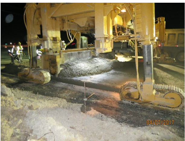
c. Top lift placer-spreader.
