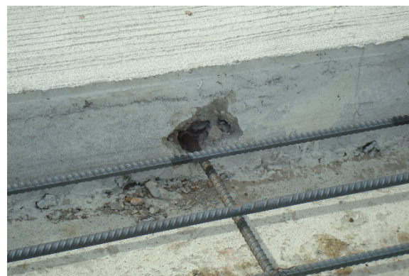
d. Consolidation problem and concrete loss at coupler along longitudinal construction joint.
