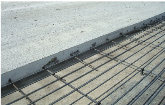
g. Example of concrete loss near some transverse steel couplers.
