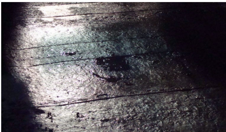
Figure 19. Oil leaked on pavement surface from top lift spreader at approximately Station 1433+75, night 2.
