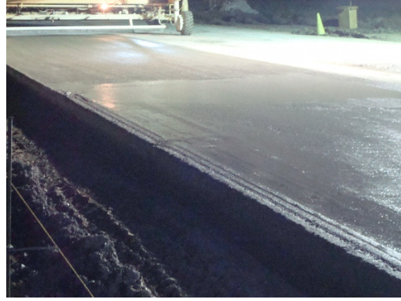
b. Example of rough top surface edge in top surface paving, night 2.
