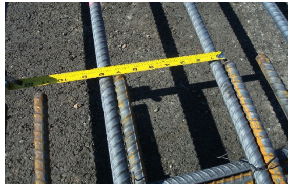
b. Longitudinal steel, No. 6 bars at 7-inch (178-mm) spacings.
