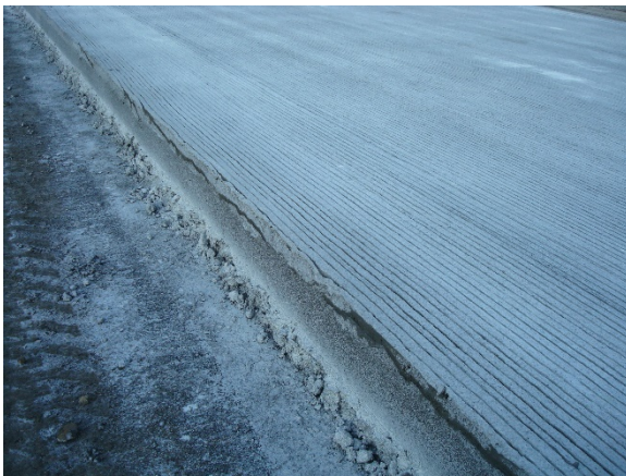
a. Tining intersecting shoulder pavement edge, night 2.
