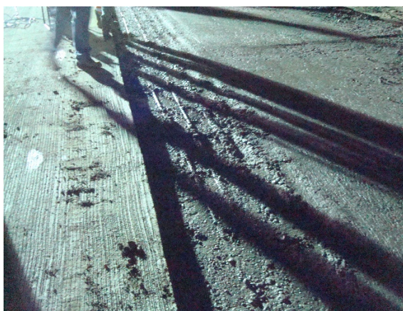
b. Exposed steel, start of night 2 paving.
