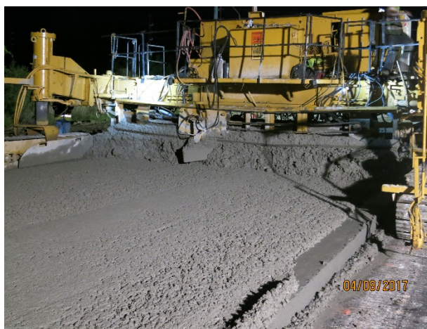
d. Top lift placer-spreader.
