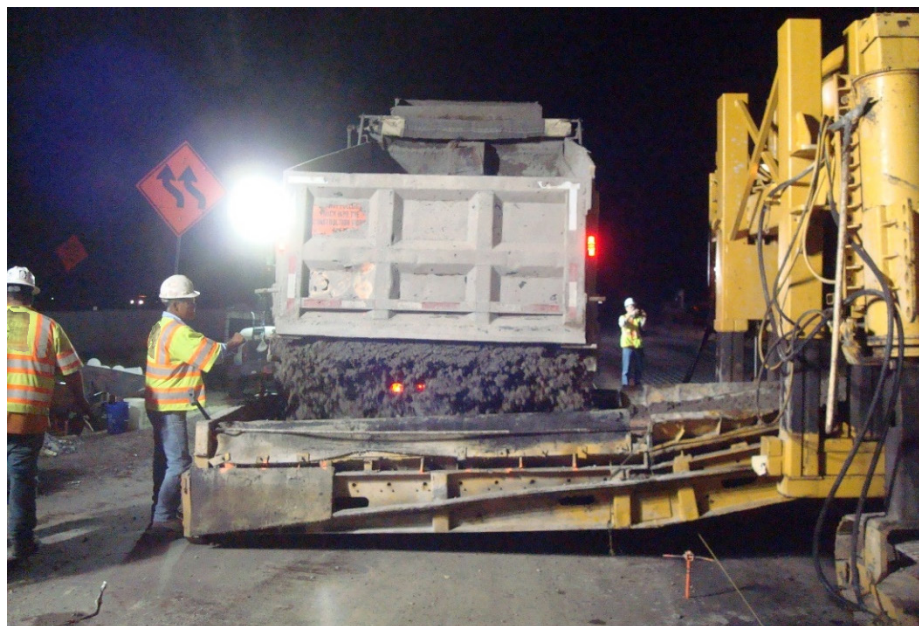
Figure 8. Concrete dump truck discharging load into conveyor for placement machine.
