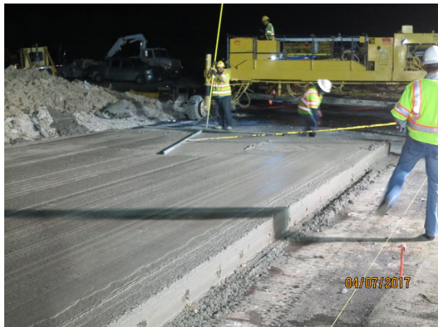
b. Hand work behind paver near header.
