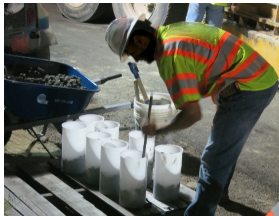
d. Preparation of test cylinders.
