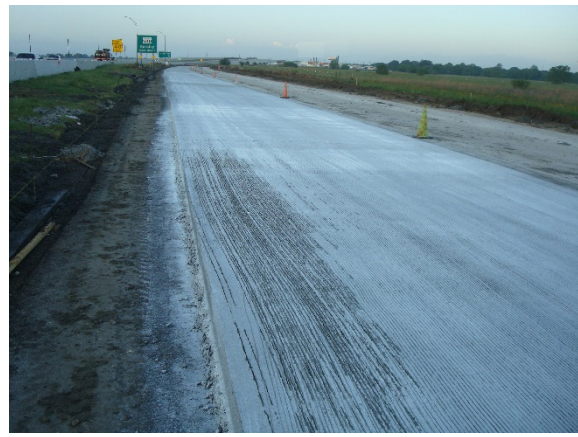
b. Deep, wandering tining near north end of night 2 paving.
