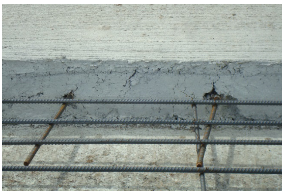
c. Shrinkage cracking and concrete loss at couplers along longitudinal construction joint.
