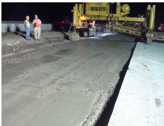
d. Filling low bottom lift areas with top lift.
