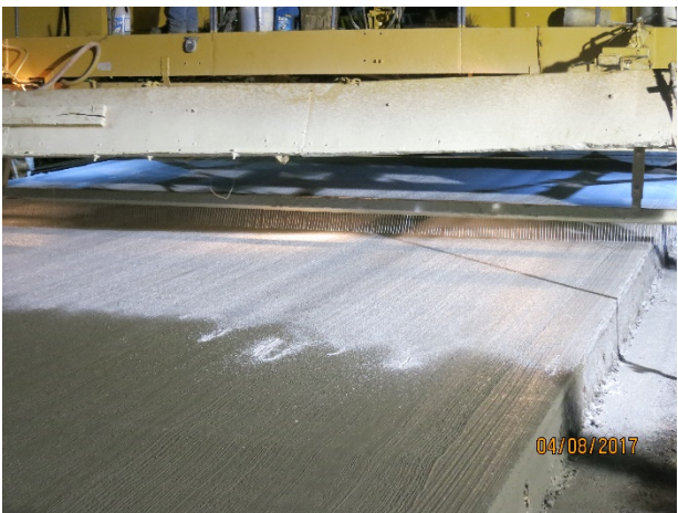
a. Tining and curing the pavement surface.
