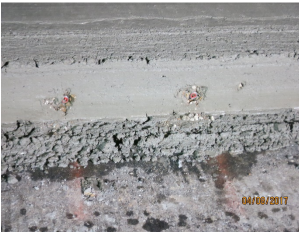
a. Exposed rebar couplers.
