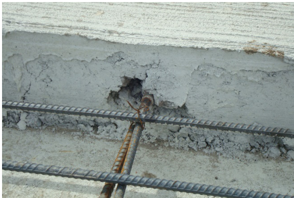
a. Excessive loss of concrete at steel coupler.
