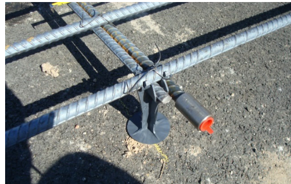
d. Transverse tie bar coupler between lanes.
