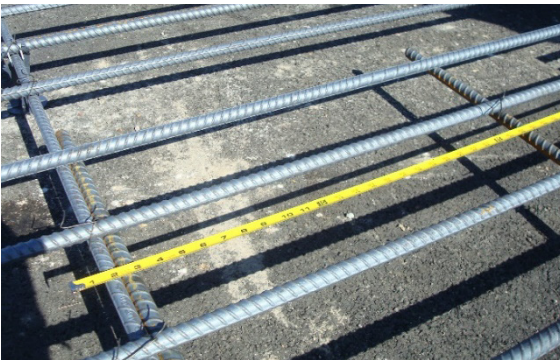
c. Transverse steel, No. bars at 48-inch (1219-mm) spacings.
