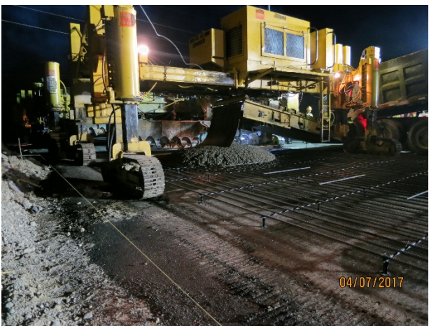
a. Bottom lift placer-spreader.
