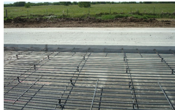
f. Coupled transverse reinforcement and tie bars (Day 2).
