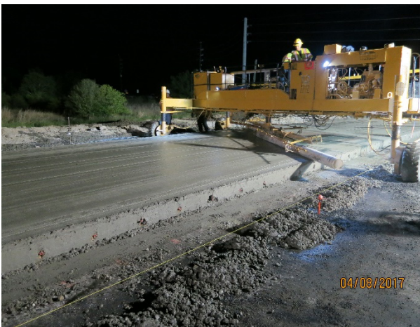
c. Tube float finishing.
