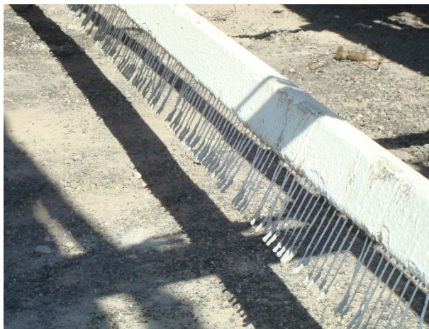
b. Rake for longitudinal tining.
