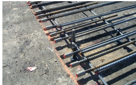
h. Construction header and reinforcing (transverse construction joint).
