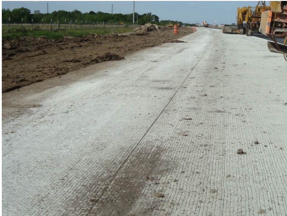
Figure 12. Lane-shoulder joint sawed in concrete placed on first night of paving.
