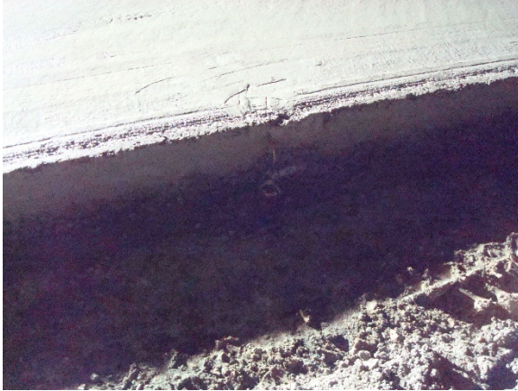
a. Example of rough top surface edge in top surface paving, night 2.
