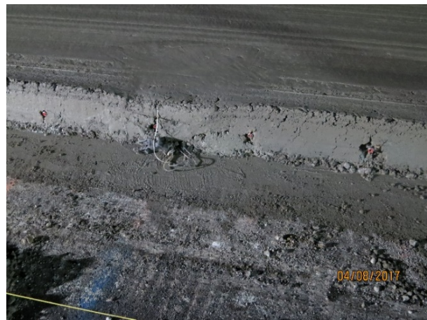
b. Sensors after paving
