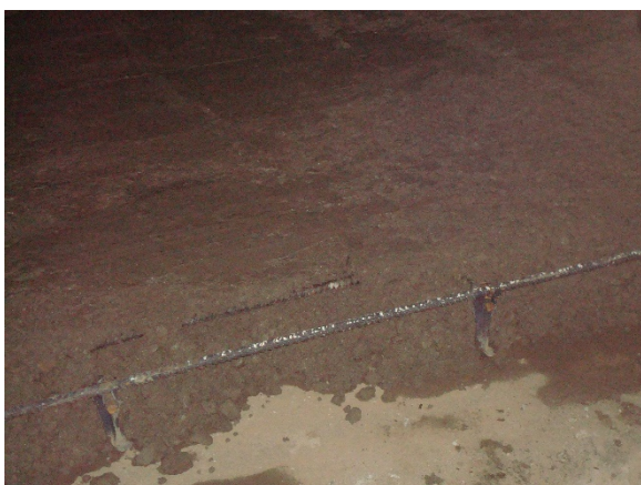
a. Exposed steel, start of night 2 paving.
