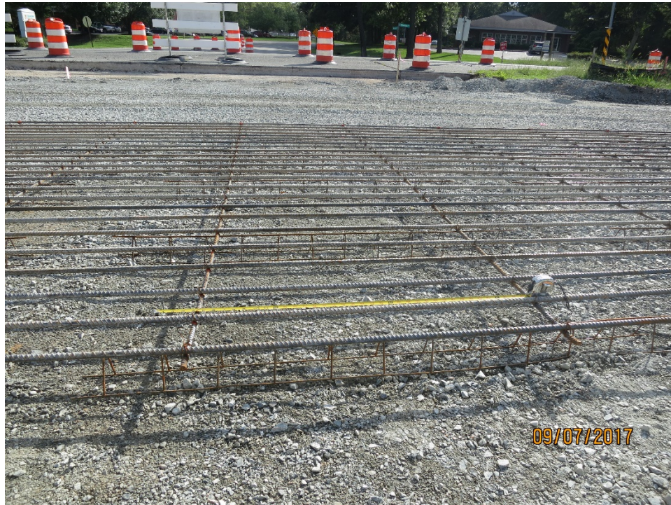
Photo B-3. Transverse reinforcement spacing.
