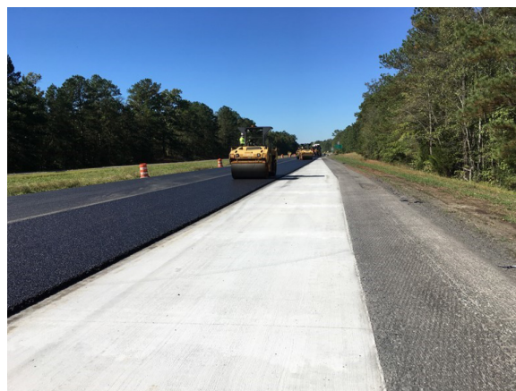
b. Compaction with smooth rollers in passing lane.
