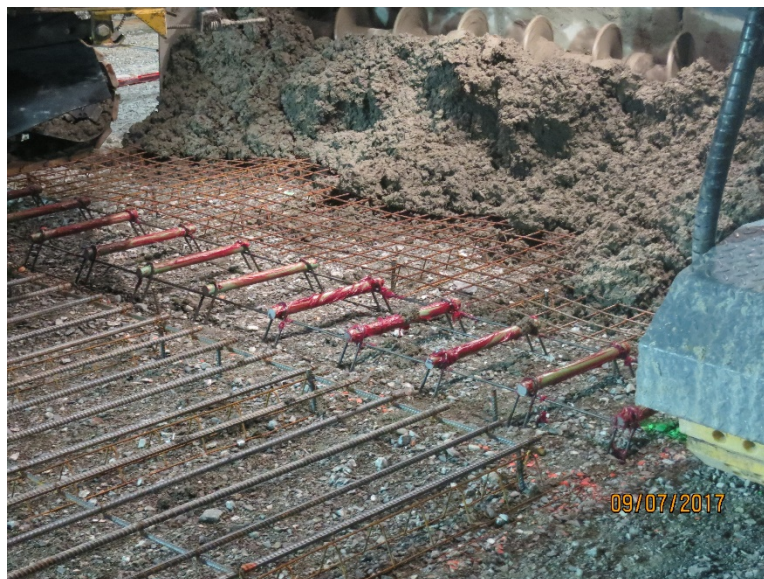
Photo B-14. Dowel bar placement in transition slabs near east end of project.
