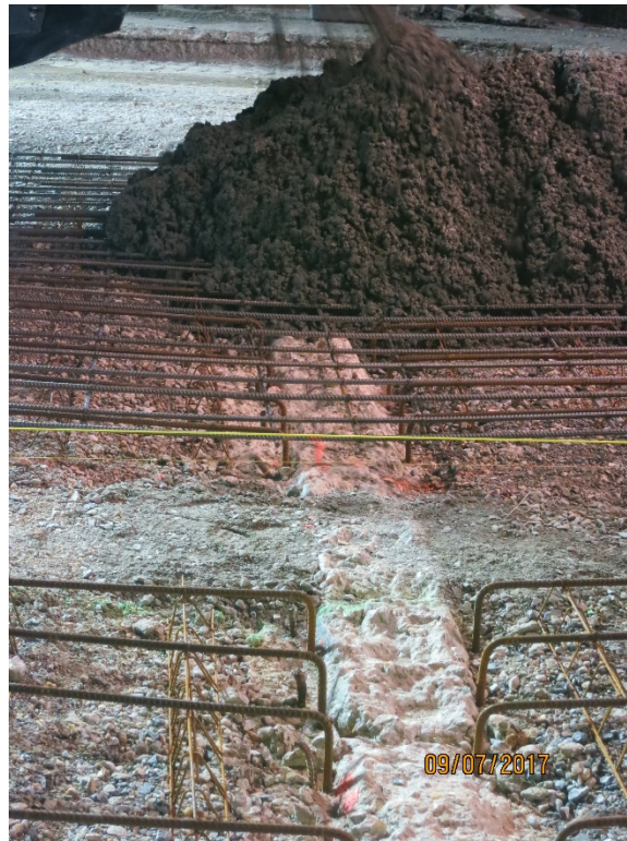
Photo B-17. Material delivery at existing anchor lug.
