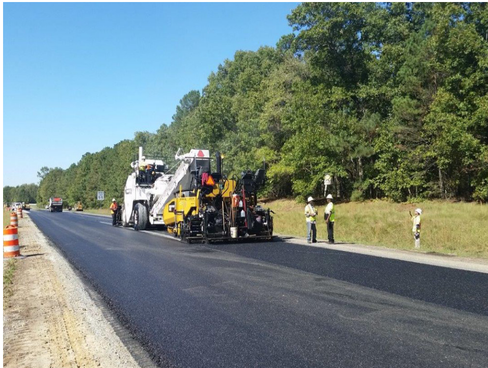
Photo B-20. Asphalt paving operation.
