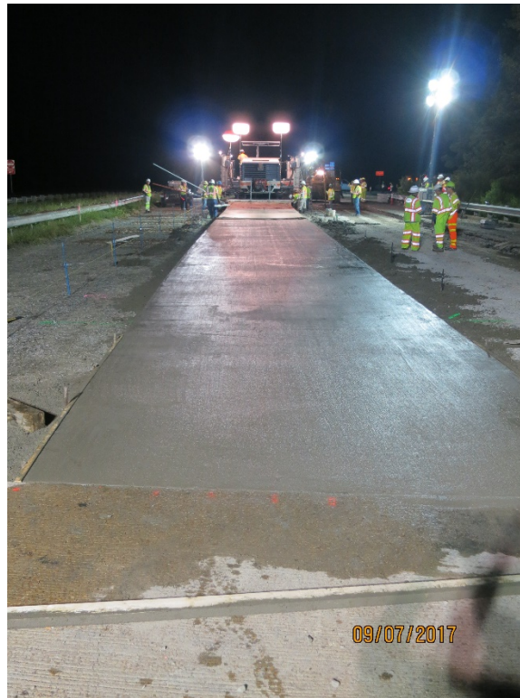
Photo B-19. Finished concrete surface.
