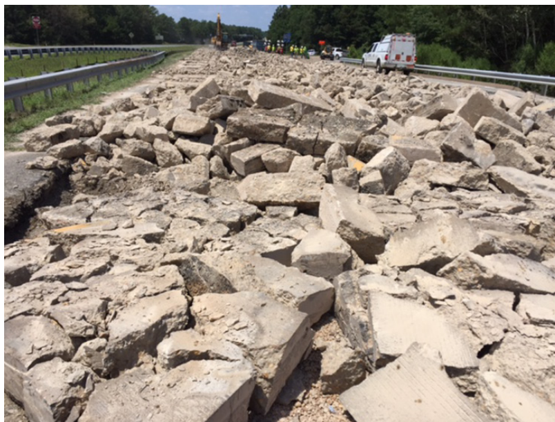
Figure 3. Broken up PCC on grade.
