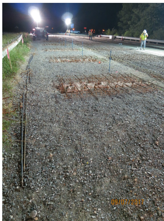
Photo B-12. Existing anchor lugs.
