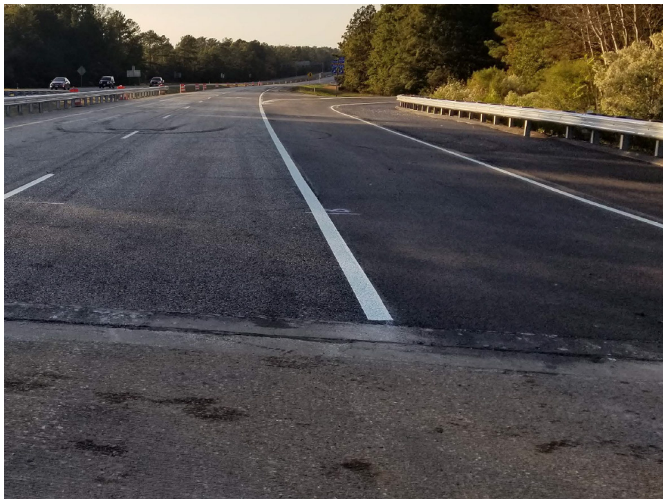
Photo B-22. Final surface view of the composite pavement.
