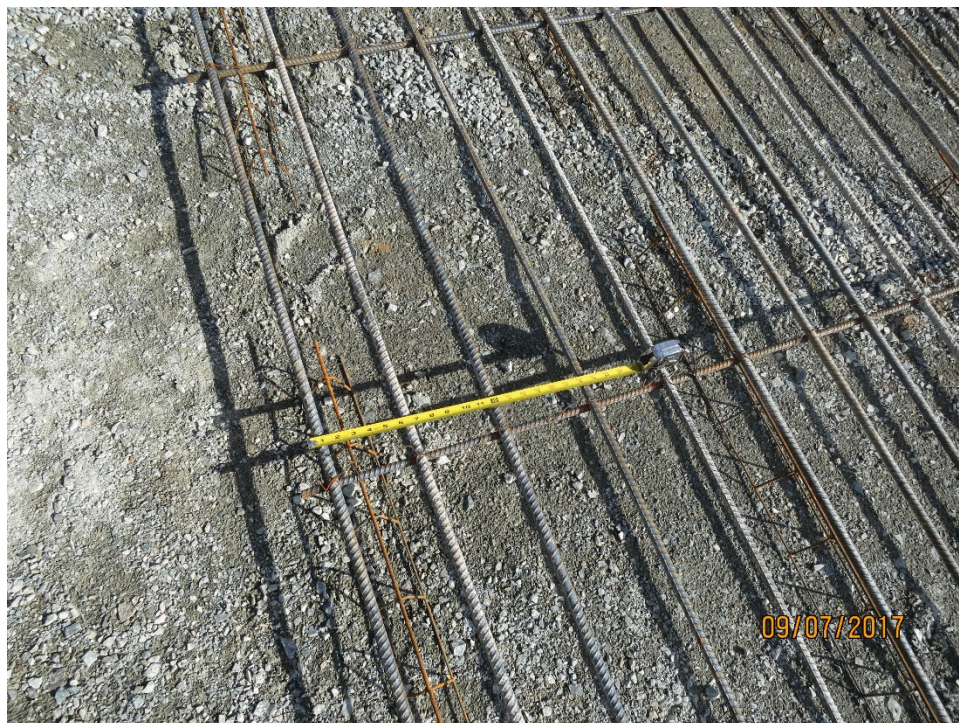
Photo B-4. Longitudinal reinforcement spacing.
