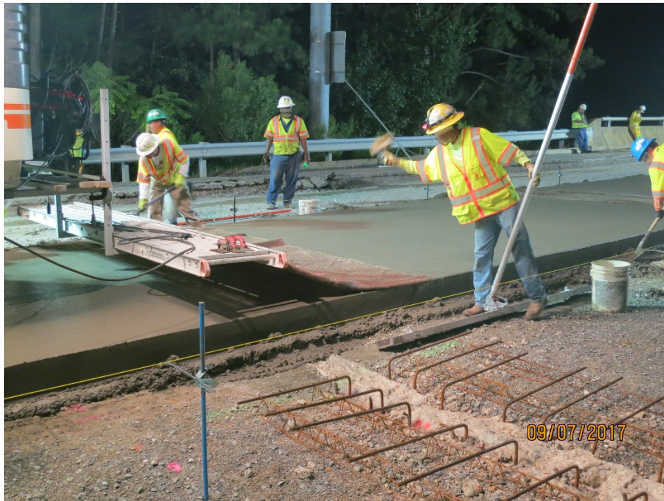
Photo B-18. Burlap drag finishing.
