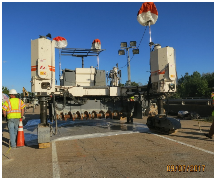
Photo B-11. Concrete paver.
