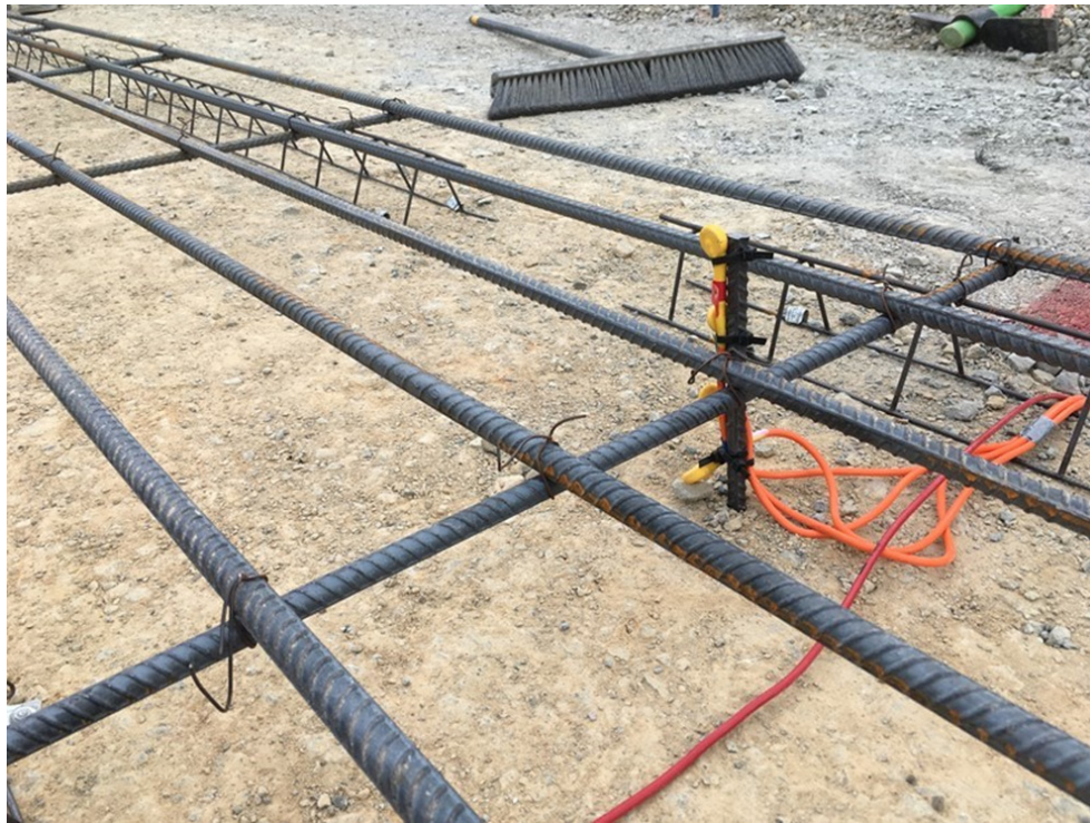
Photo B-9. Temperature logging sensors installed in slab.
