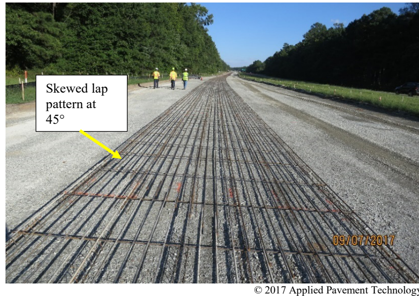
Figure 4. Layout of reinforcing steel, single lane.
