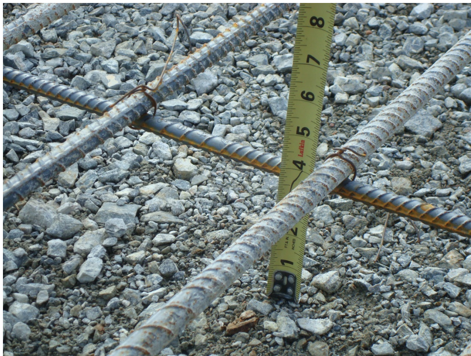
Photo B-6. Reinforcement depth.
