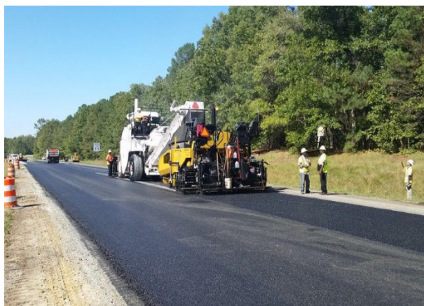
a. SMA paving in driving lane.
