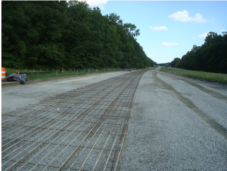
Photo B-5. Layout of steel reinforcement.
