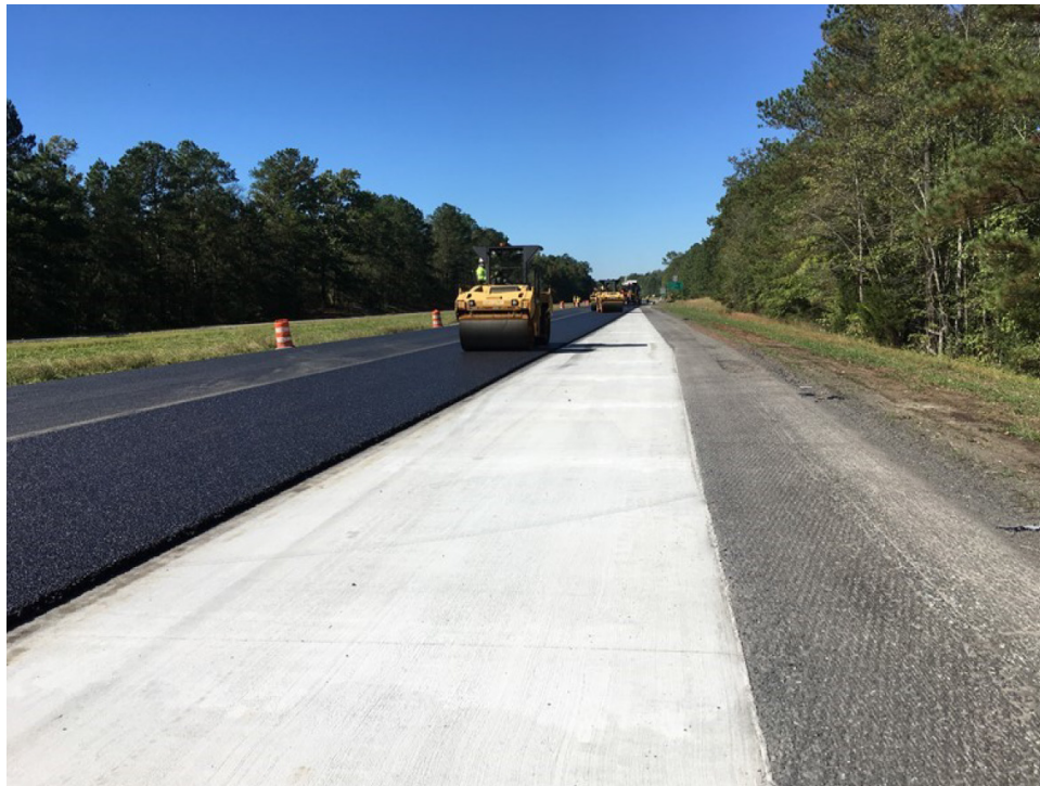
Photo B-21. Asphalt compaction operation.
